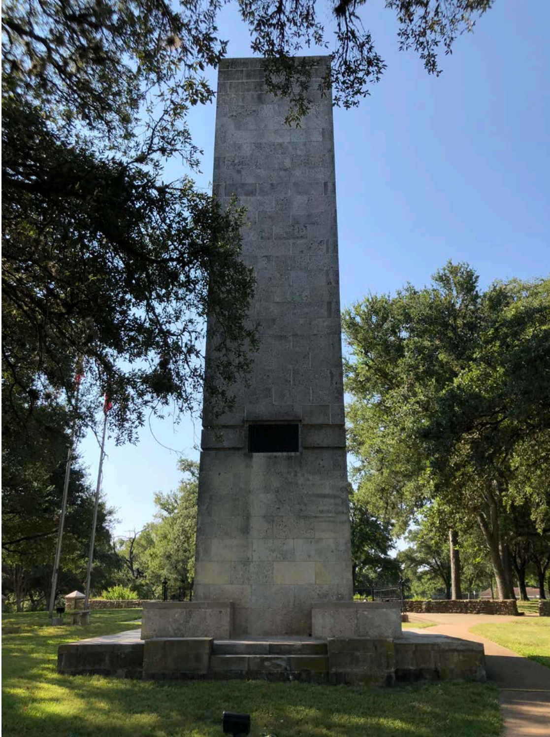
Photo 13: Centennial Monument rear elevation—camera facing southeast.
