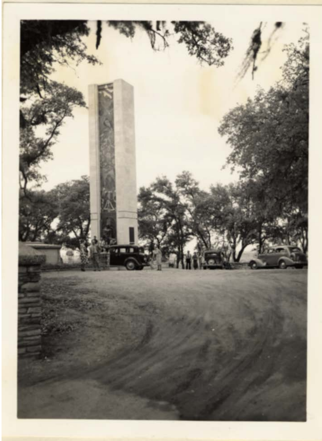
Figure 18: In 1938, the park was within a larger parcel owned by the Kreische Family. Visitors to the monument and tomb accessed it via a state highway that bisected the Kreische property to a 0.36-acre fenced park. Source: Texas Department of Transportation Archives
