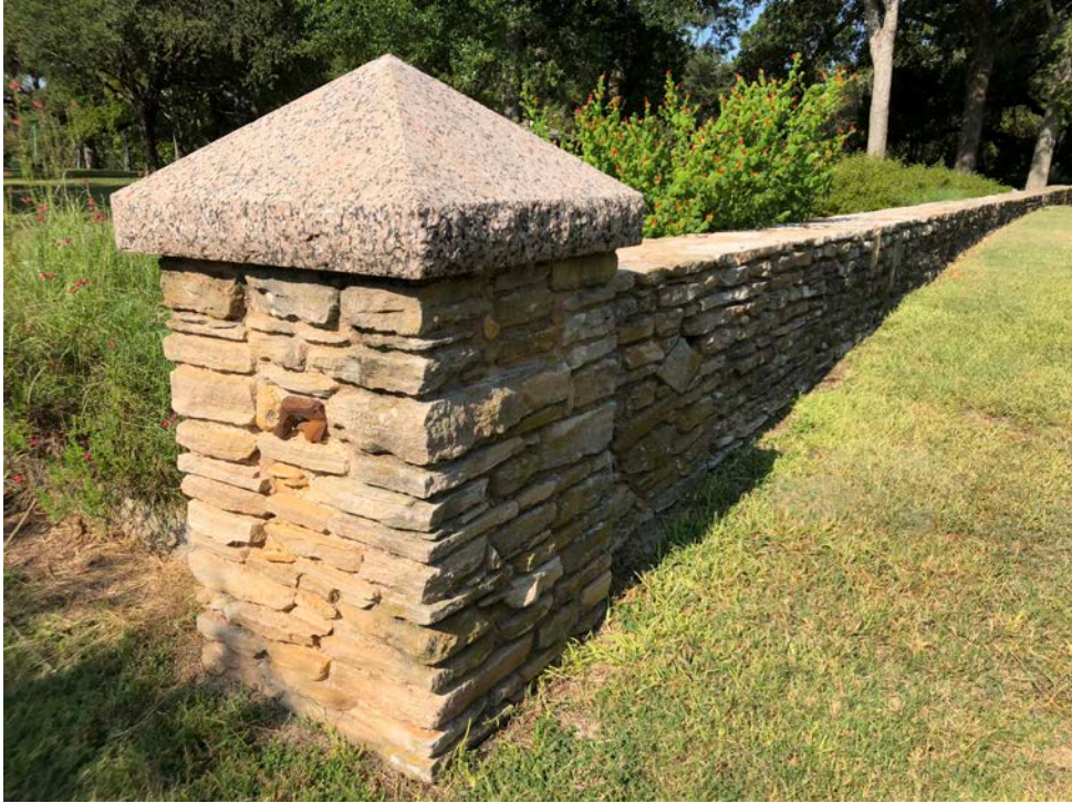
Photo 4: Stone fence and entry column with granite cap—camera facing southwest. The fence (considered a contributing structure) is a park improvement constructed by the Texas Highway Department in 1933.
