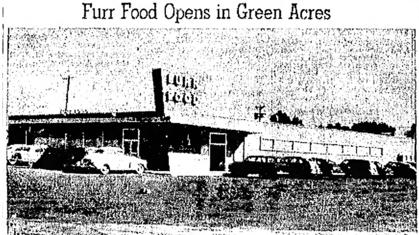
Figure 6. Historic photo of Furr Food store, one of the commercial buildings associated with the Green Acres development, Amarillo Daily New , October 13, 1950, p26.
