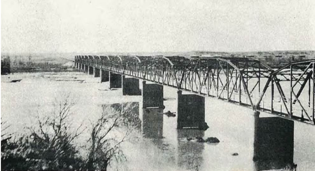
Figure 26. Red River Bridge on SH 2 in Montague County, completed 1931. (Source: Gibb Gilchrist, Texas Highway Department 1927-1937, 109)
