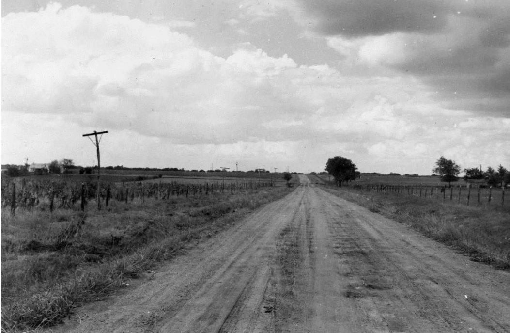
Figure 38. FM 155 in Fayette County before improvement. (Source: TxDOT Library)
