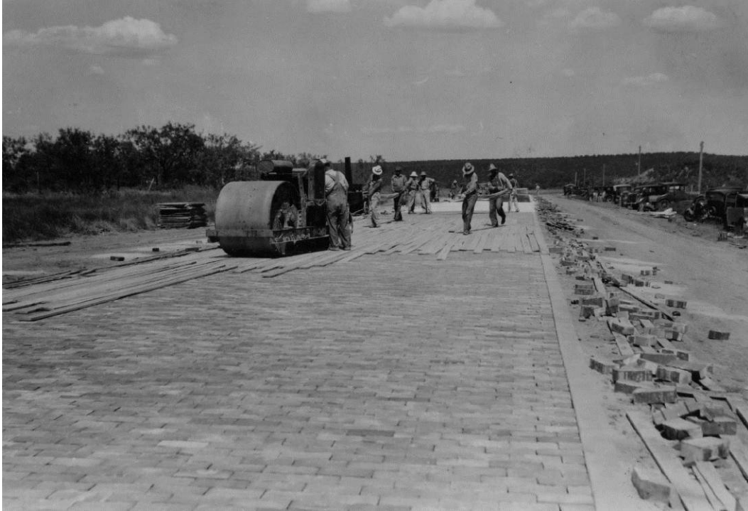
Figure 36. Installing brick pavement on US 180 in Parker and Palo Pinto Counties, 1938. At the time, the roadway was designated as Alternate US 80 and roughly followed the historic alignment of the Bankhead Highway route. (Source: Texas Department of Transportation Photo Library)
