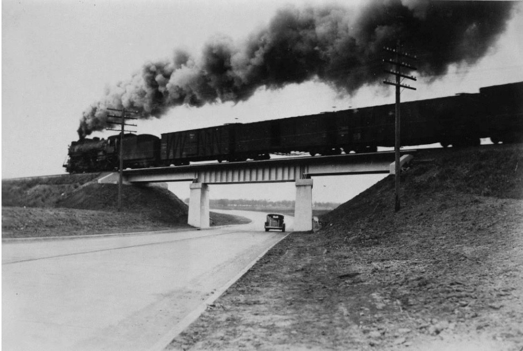
Figure 37. Recently completed grade separation structure, US 81 in Montague County, November 1936. (Source: Texas Department of Transportation Photo Library)
