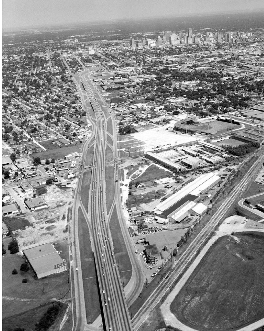
Figure 41. 1950s aerial view of the Gulf Freeway looking toward downtown Houston and illustrating the use of the frontage road
