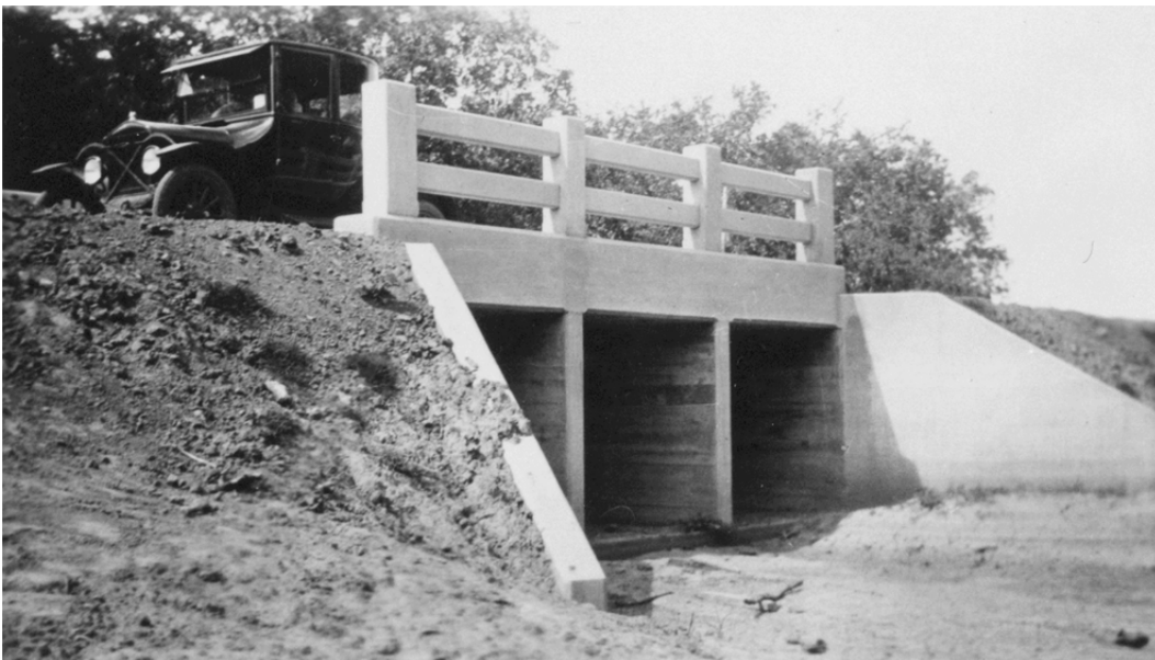
Figure 20. Photo of a culvert from the early 1920s. (Source: Texas Department of Transportation Photo Library)
