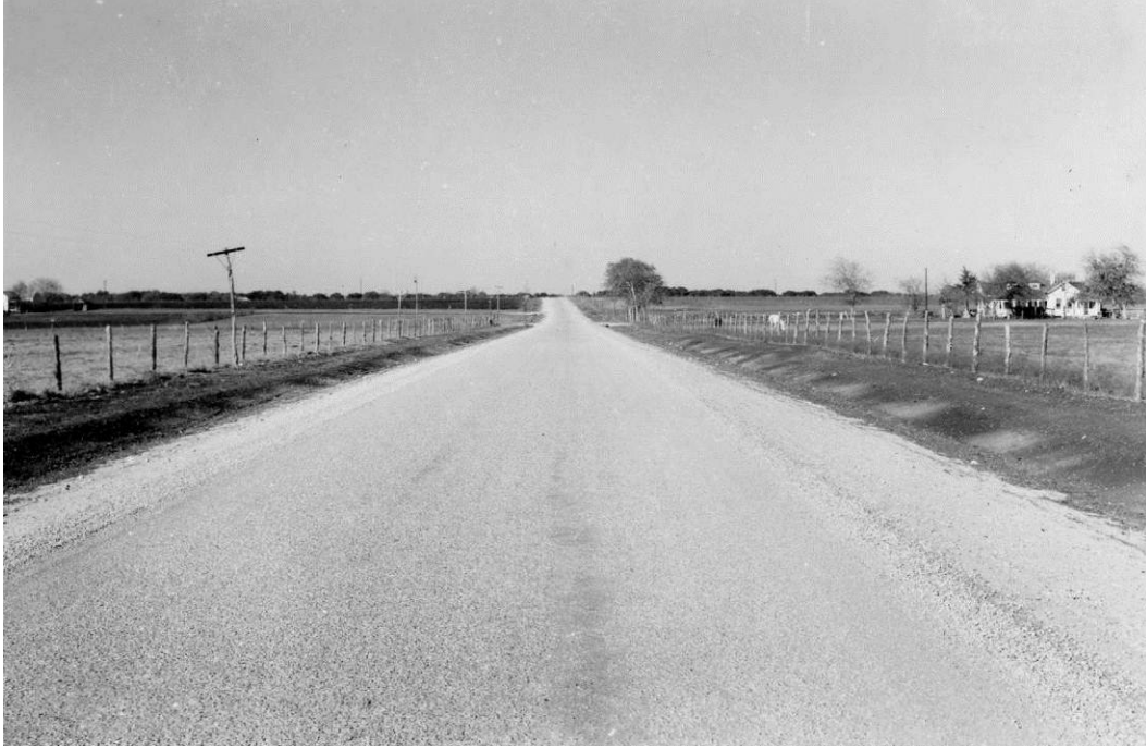
Figure 39. FM 155 in Fayette County after improvement. (Source: TxDOT Library)
