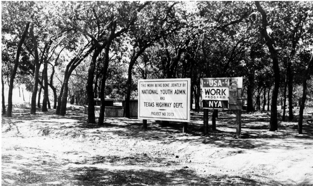
Figure 31. Joint THD/NYA roadside park construction project (Source: Texas Department of Transportation Photo Library)
