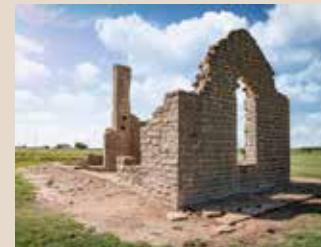
Administration building ruins
