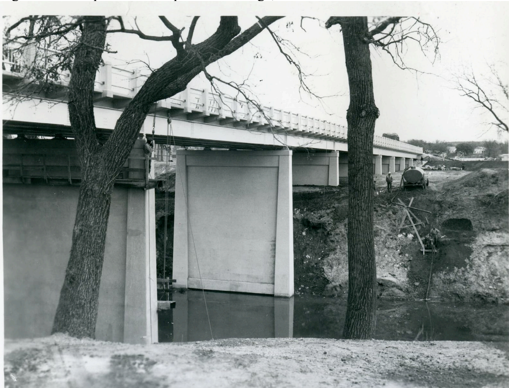
Figure 6: WPA photo of Bosque River Bridge, 12/30/1940. Source: Ibid.
