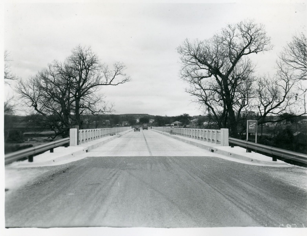
Figure 5: WPA photo of Bosque River Bridge, 12/30/1940. Source: Ibid.
