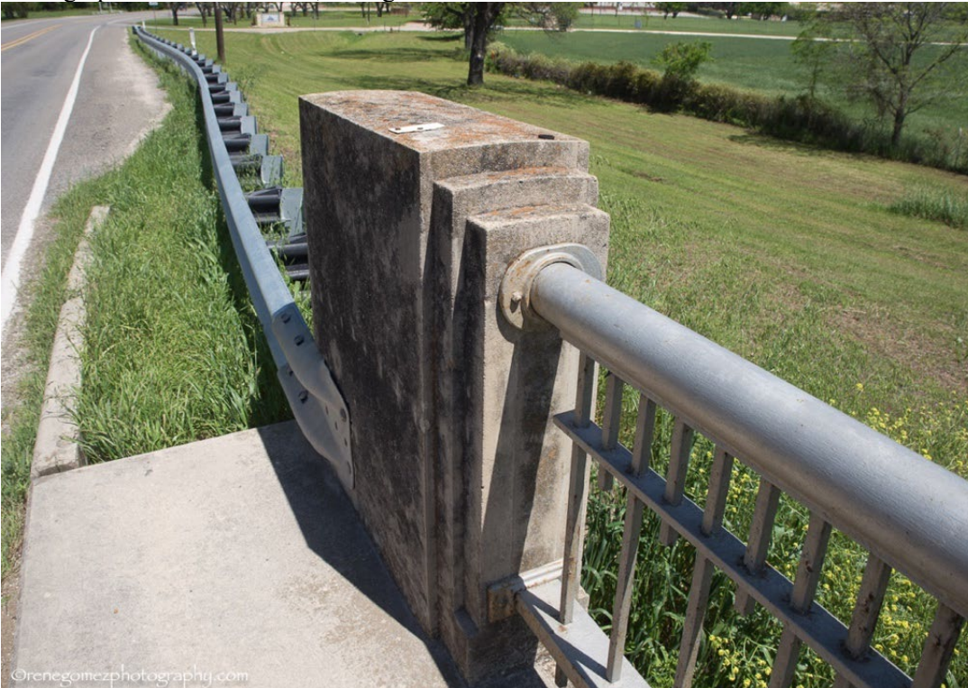
Photograph 8: South elevation, facing north
