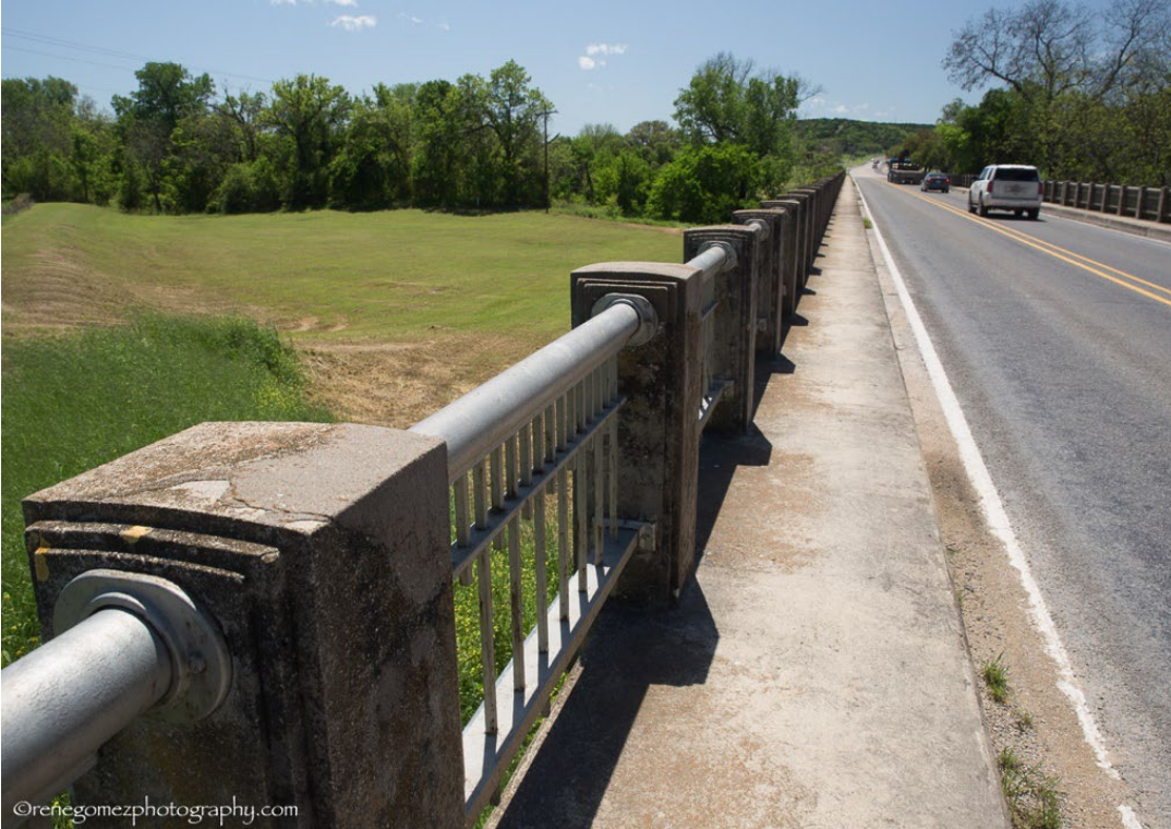
Photograph 7: North elevation, facing south
