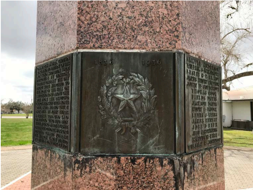
Photo 6: Bronze-cast state seal on granite pylon base—camera faces south, February 15, 2018.
