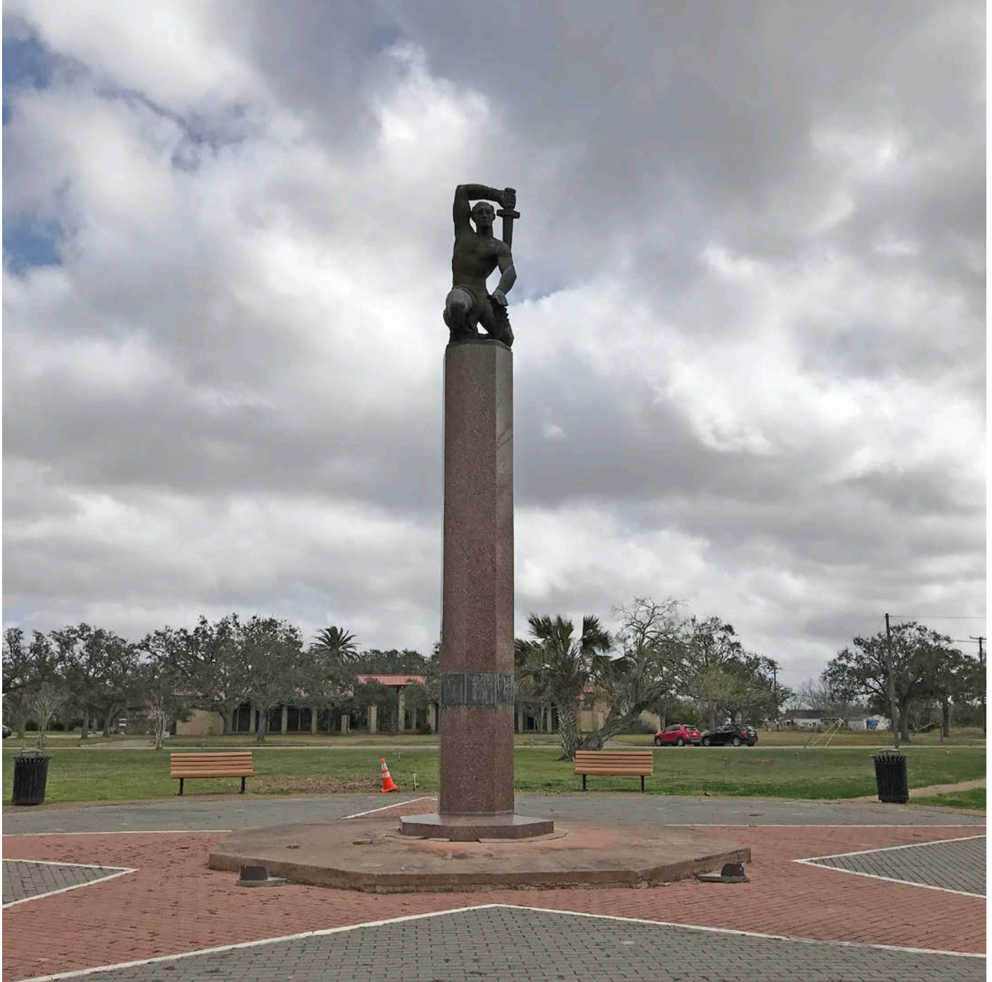
Photo 2: King's Men monument (front/west elevation)—camera faces east, February 15, 2018.
