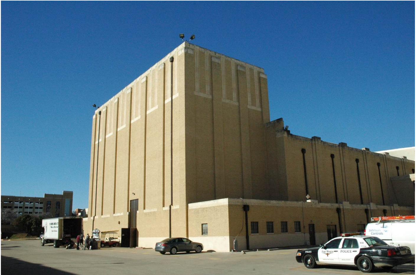
Will Rogers Auditorium, in service court, looking northwest at fly loft
