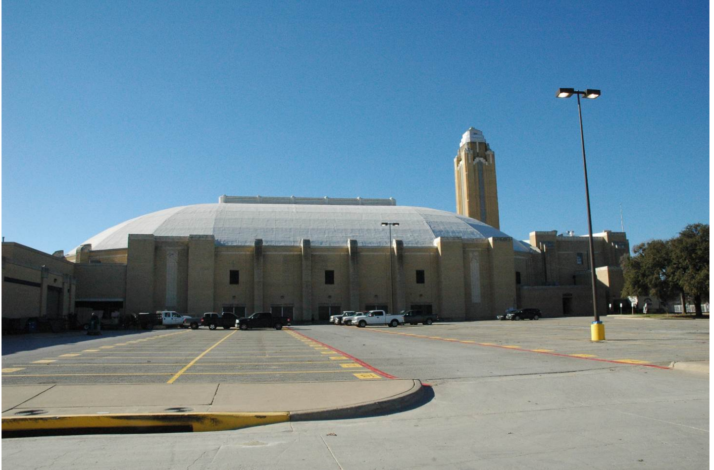
Photo 10 East elevation, camera facing west
