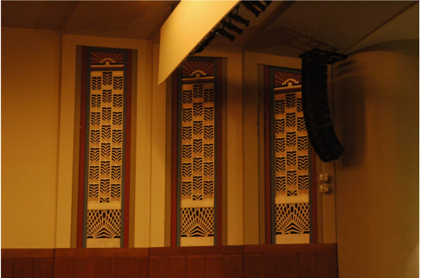
Photo 17 Auditorium stage metal screens and wood paneling
