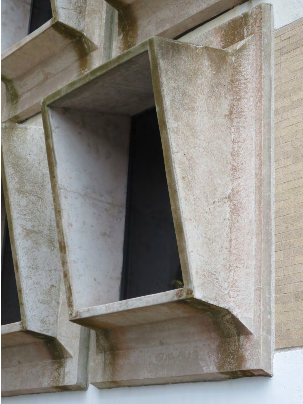
Photo 10 Close-up precast concrete sunshade
