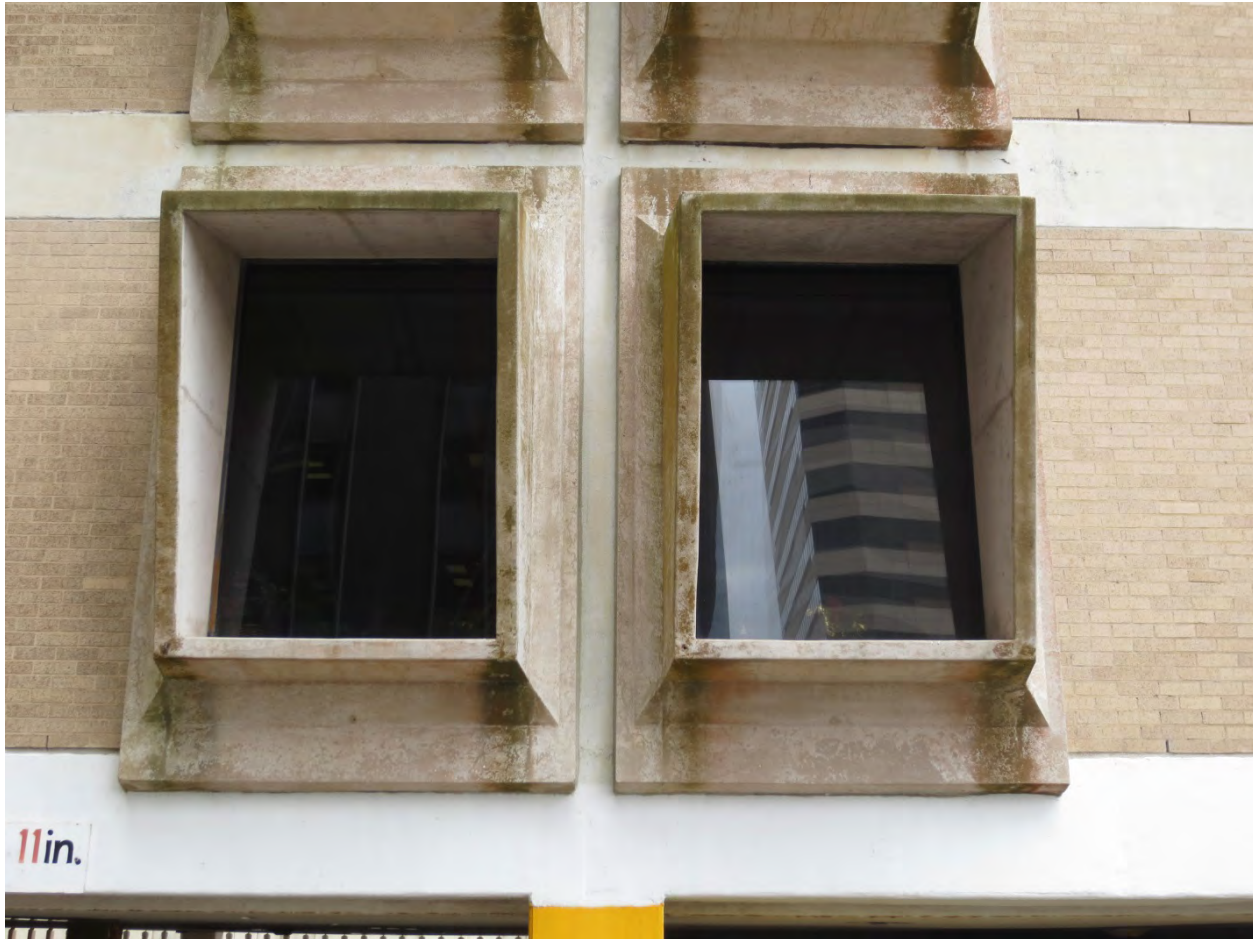
Photo 11 Close-up pair of precast concrete sunshades
