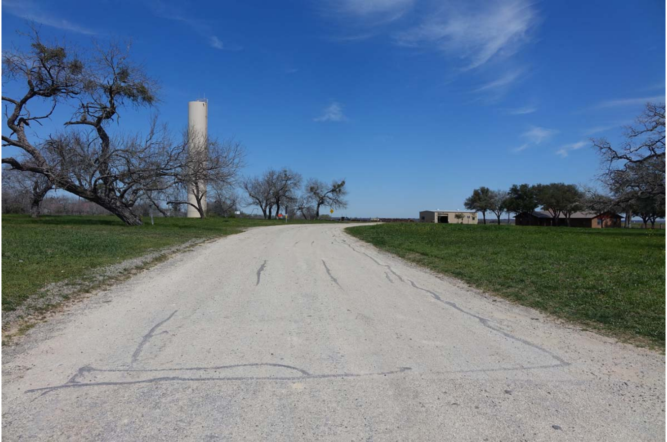
Photo 12 Spur 95 from Centennial Roadside Park Camera facing NW
