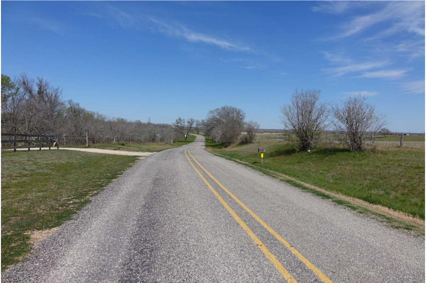
Photo 23 Spur 95 leaving Centennial Roadside Park Camera facing north
