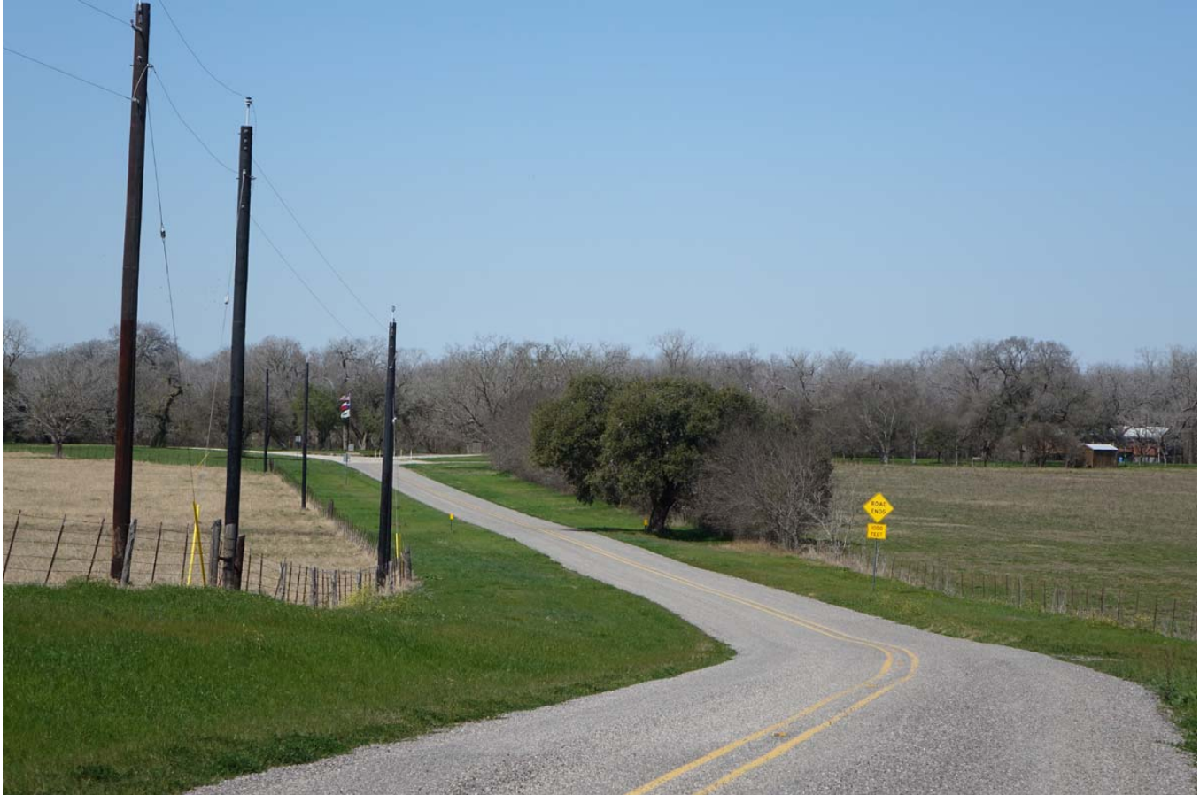
Photo 20 Spur 95 approaching 1903 Monument Park Camera facing north
