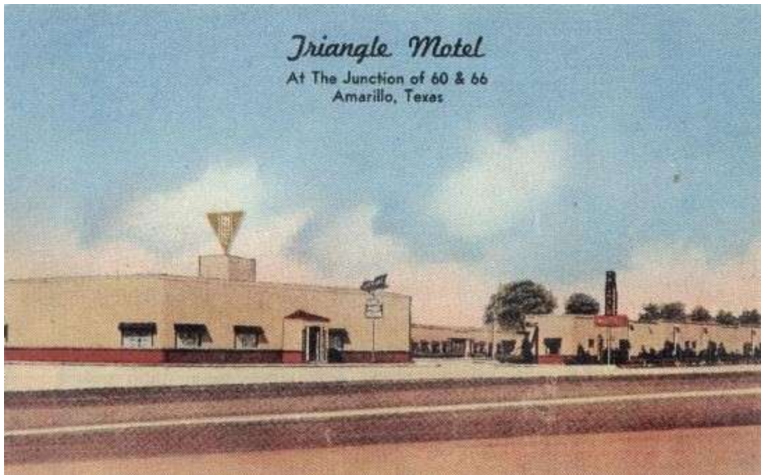
Figure 3. Triangle Motel after remodeling in 1956. View northeast from US 66 (1926-1956).
