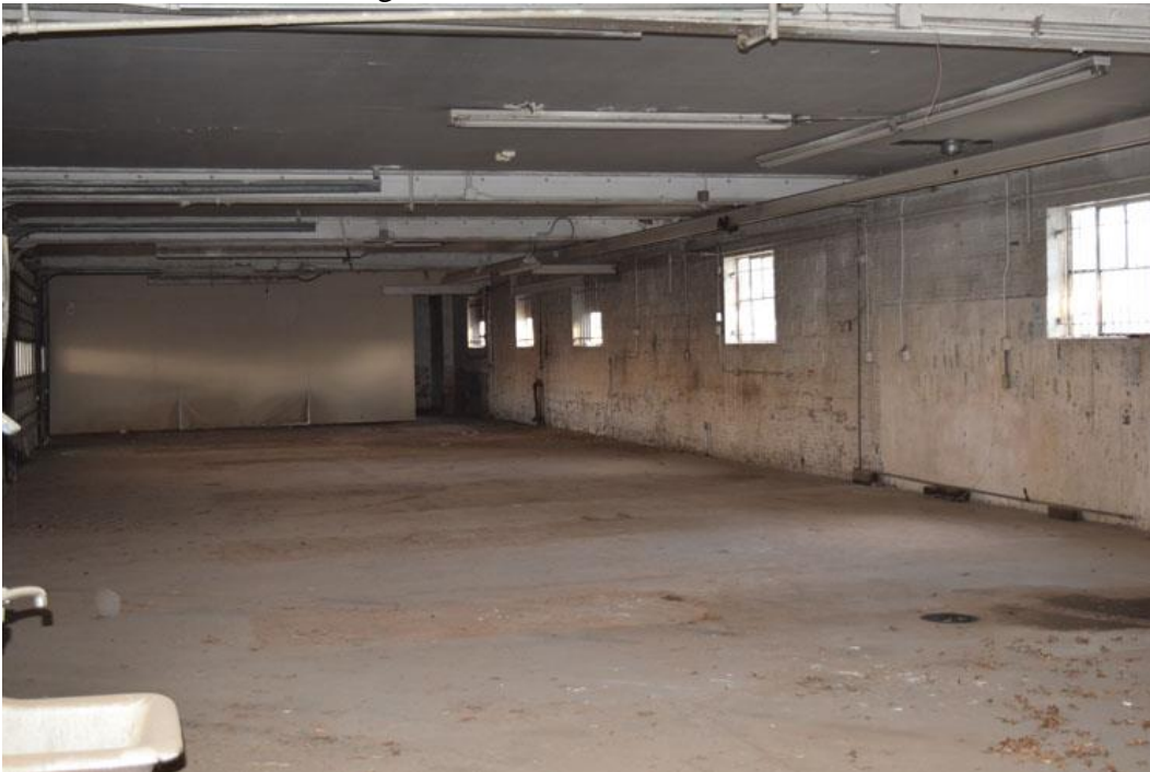
Photo 12: Service area. Camera facing east.
