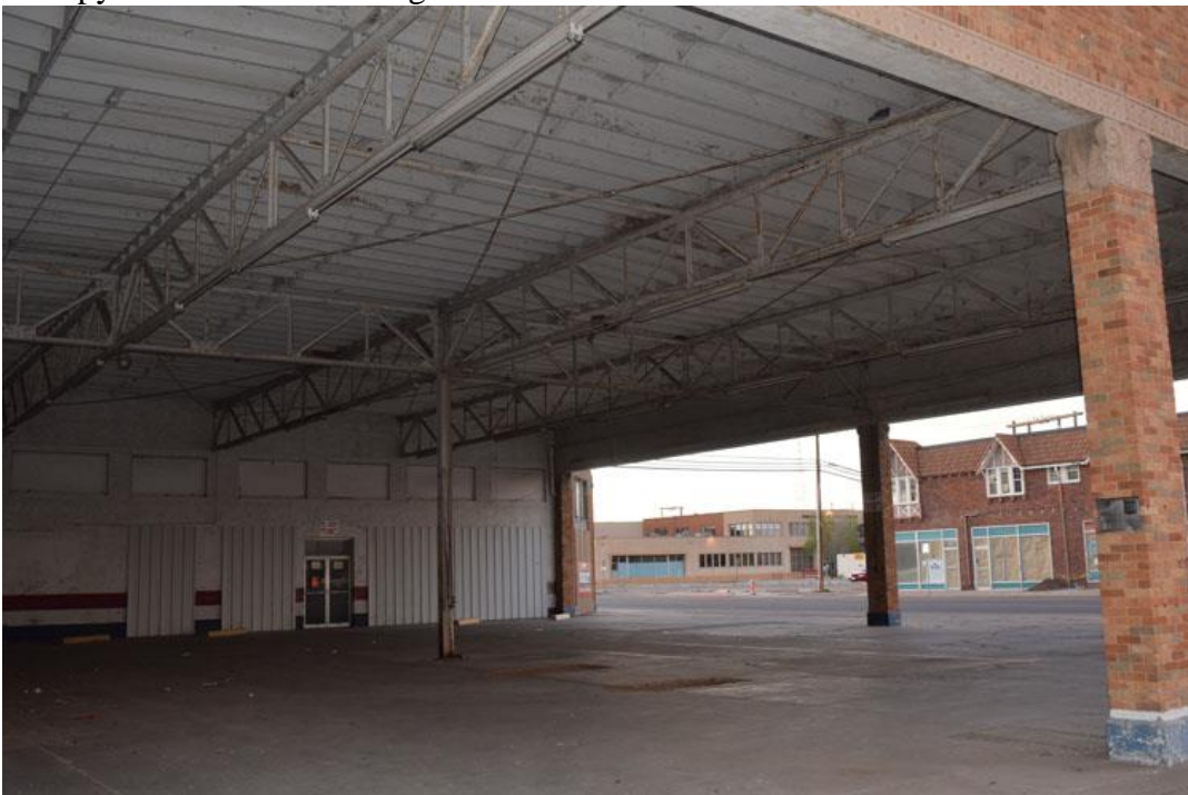
Photo 8: Canopy detail. Camera facing northwest.
