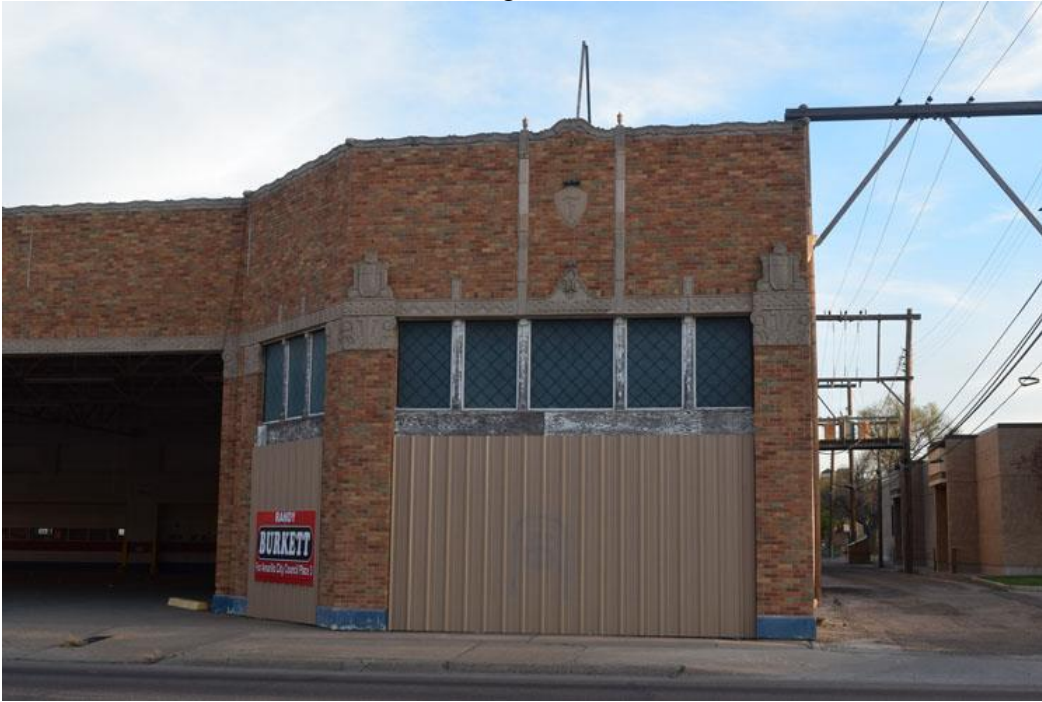
Photo 3: Detail of north elevation. Camera facing south.
