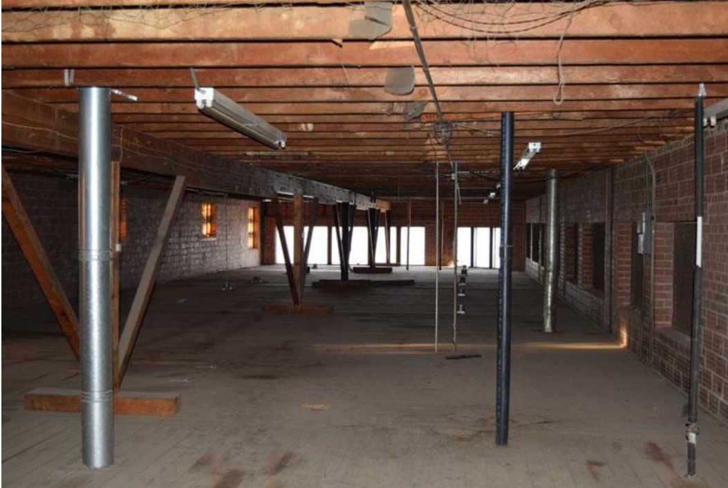
Photo 15: 2 nd floor tire storage area. Camera facing north.
