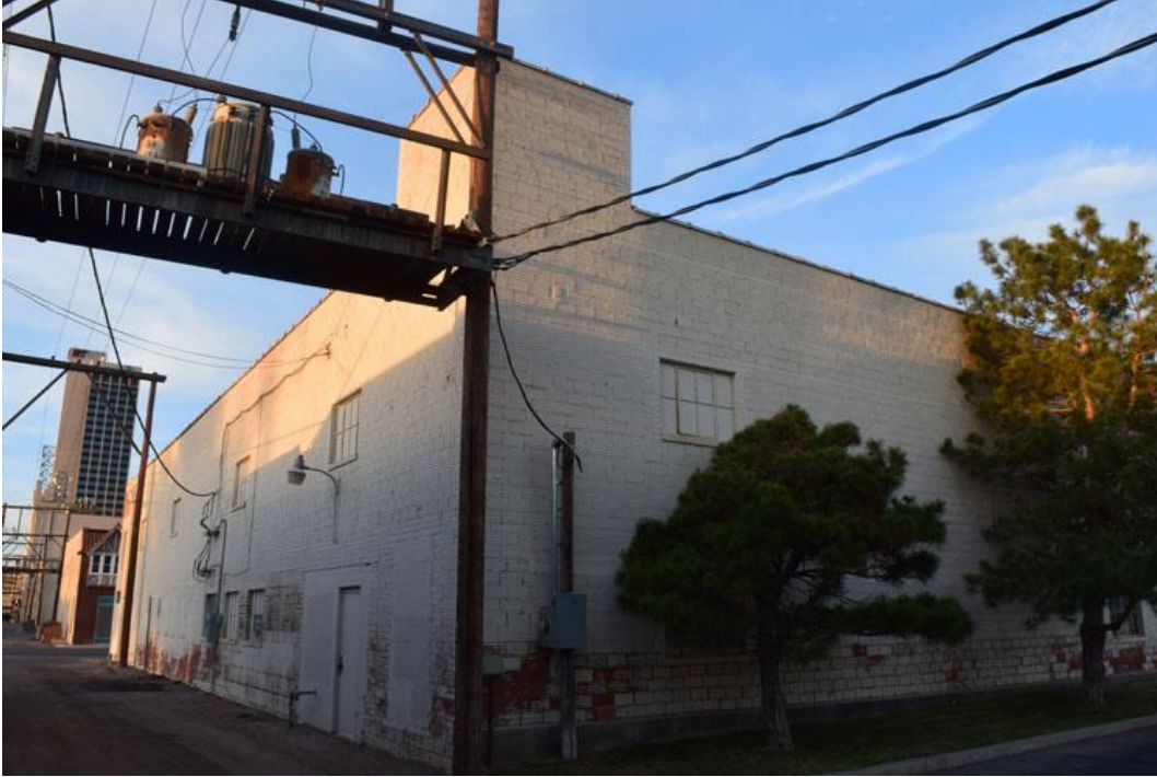
Photo 7: Partial southwest oblique. Camera facing northeast.
