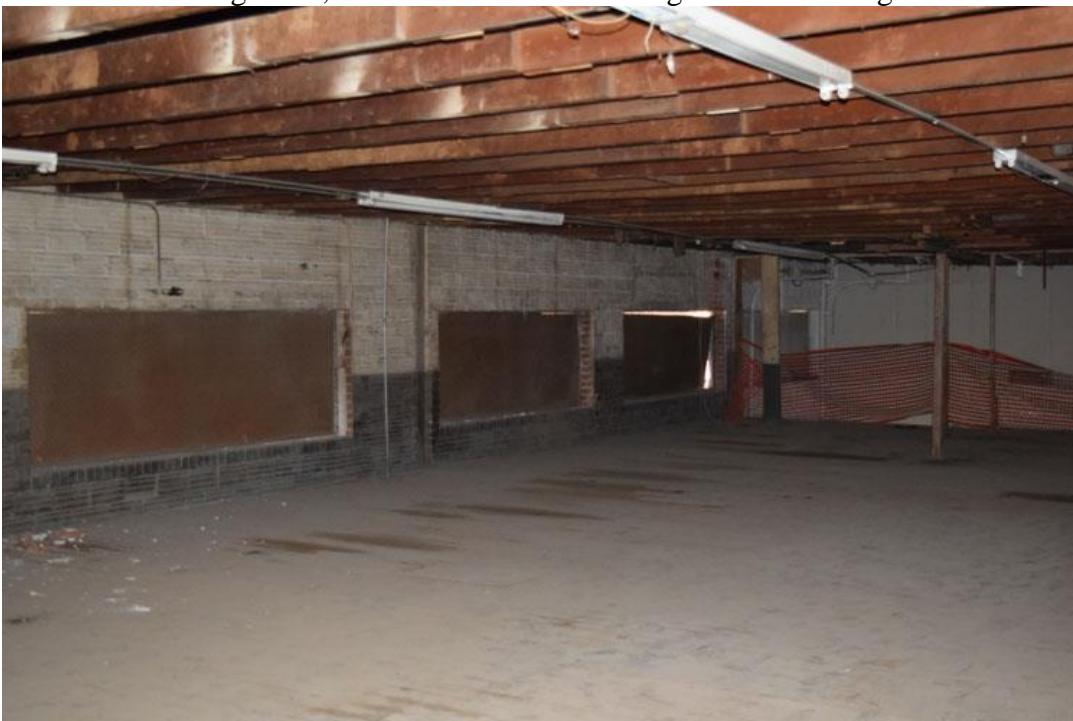
Photo 16: 2 nd floor tire storage area, over service area. Showing the north facing windows. Camera facing northeast.
