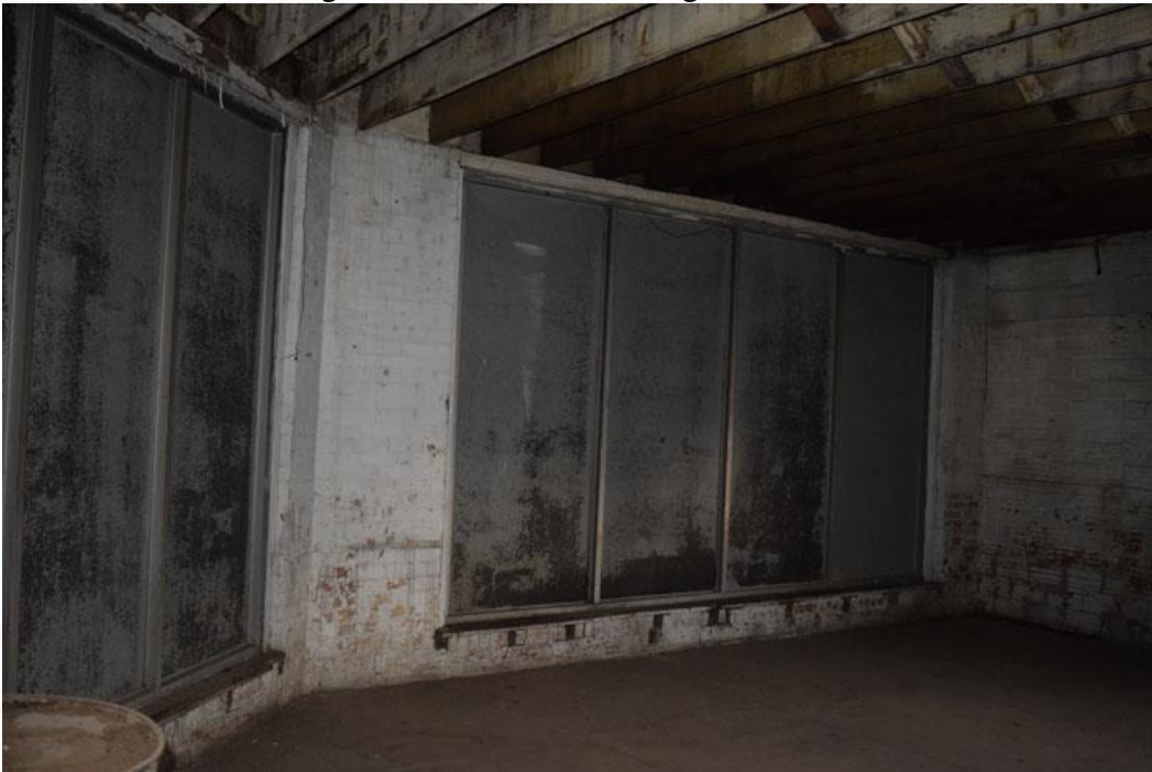
Photo 14: Room in the east-facing elevation. Camera facing northeast.
