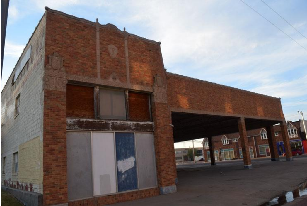
Photo 5: Detail of east elevation. Camera facing northwest.
