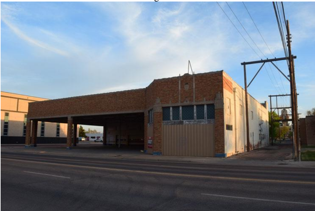
Photo 2: North elevation. Camera facing southwest.
