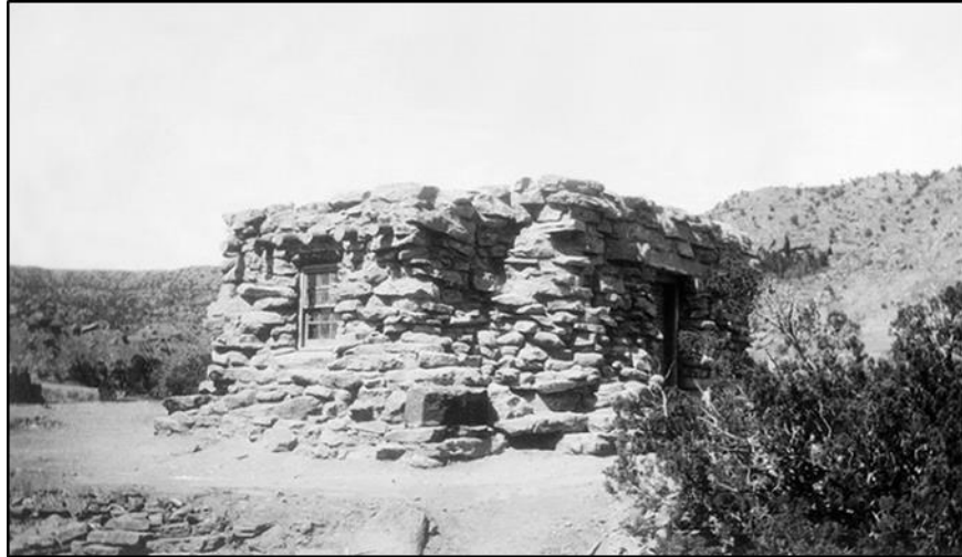
Figure 217. Photograph of a stone cabin within the new Palo Duro Canyon State Park, Randall County, ca. 1935. Note the design of the cabin using rubble masonry and a flat roof to reflect the natural appearance of the surrounding canyon and plateaus. Source: Texas Parks and Wildlife Archives, http://texascccparks.org/archive/#/h/parks/palo-duro (accessed April 8, 2014).
