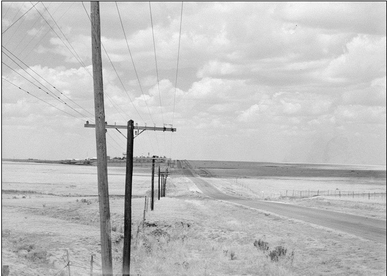
Figure 213. Photograph of the highway north of Amarillo, Randall County, taken by Dorthea Lange in 1939. This segment passes through the southern end of the Great Plains, which produced large yields of wheat before the Dust Bowl. The North Texas Highway was used to transport cattle and wheat to regional market centers. Source: Dorthea Lange, "Great Plains and highway north of Amarillo, Texas," Farm Security Administration/Office of War Information Collection, Black-and-White Negatives, Library of Congress, http://www.loc.gov/pictures/collection/fsa/item/fsa2000004593/PP/ (accessed April 8, 2014).
