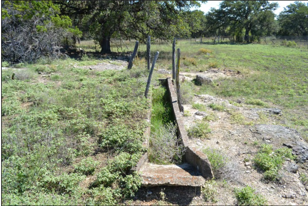
Figure 5-54. Concrete dipping vat.
