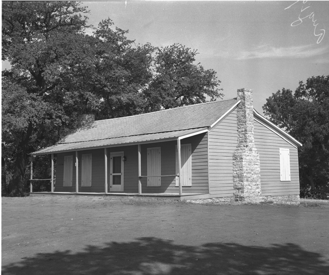
Figure 10: South and east elevations, after restoration, August 19, 1936., (Courtesy, Fort Worth Star-Telegram Collection. Special Collections, The University of Texas at Arlington Library, Arlington, Texas, AR406-6-#437).
