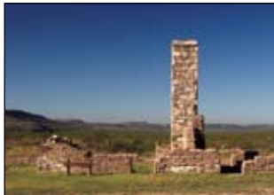
Company K Enlisted Men's Barracks
