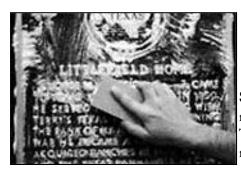
**Step 3:** Thoroughly clean the marker surface with soap and water. Towel dry and allow time for the marker surface to dry completely.
