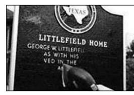
Step 7: After removing masking tape from the marker border and base, use a battery-operated or electric sander and 80 grit sandpaper or a hand sanding block to remove black lacquer from raised text. Use care not to remove black lacquer from flat surface areas. Lightly use the sander to clean marker border and base. Use 120 grit sandpaper to manually polish border and raised
