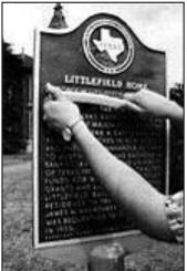
**Step 1:** Use a stiff wire brush to remove flaking or other debris; always use a side-to-side or left-to-right motion while cleaning the surface. Debris may also stick inside the raised lettering. If this happens, carefully use a sharp tool or knife to remove debris.
