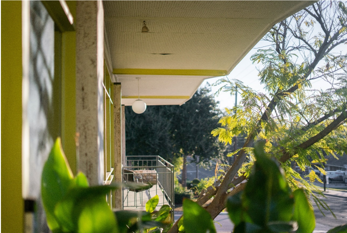
Photo 5: Soffitt detail. View east.
