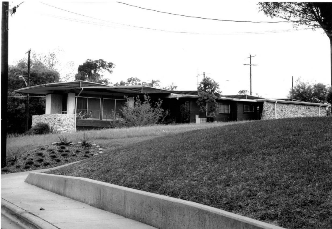
Photo 8: North elevation. View south.
