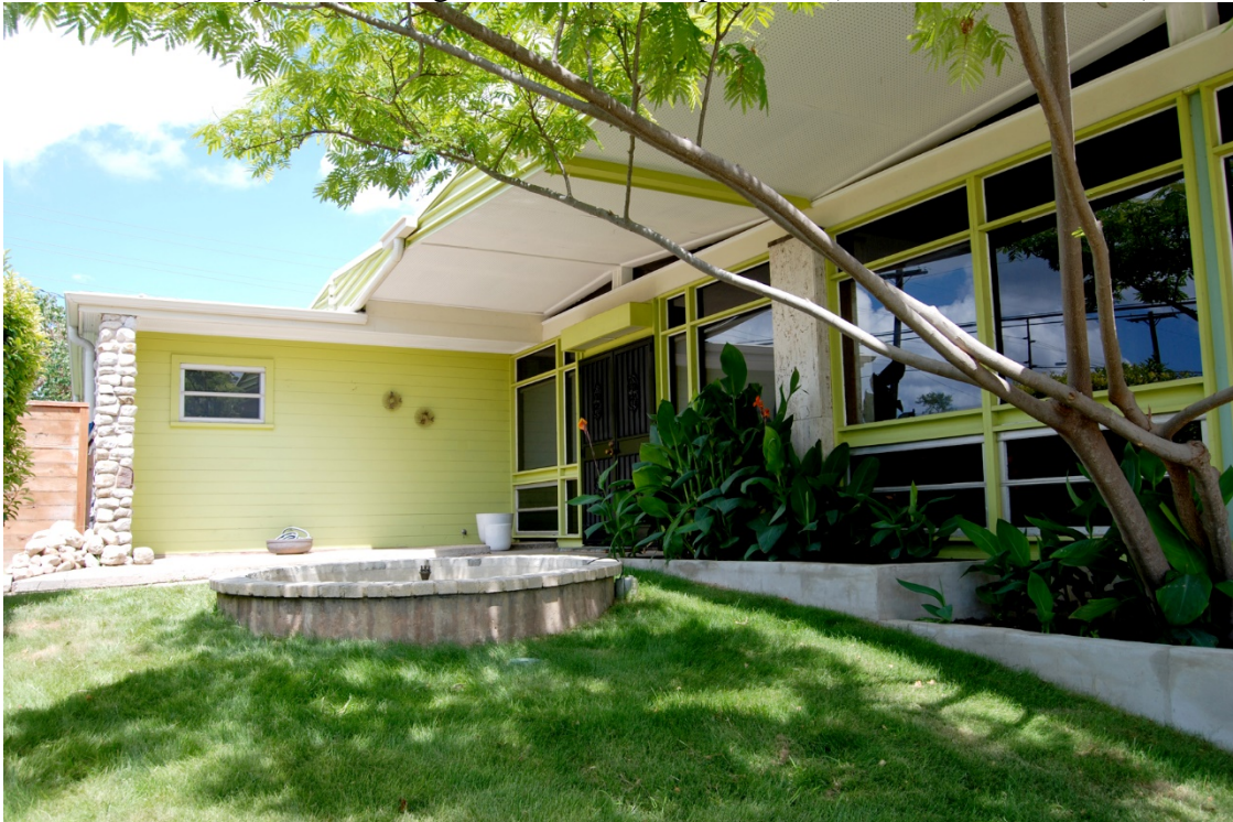
Photo 4: South façade with original fountain and planters. (Kathleen Conti, 2009)
