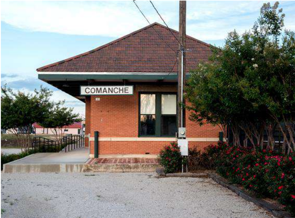
Photo 7: West elevation—camera facing east
