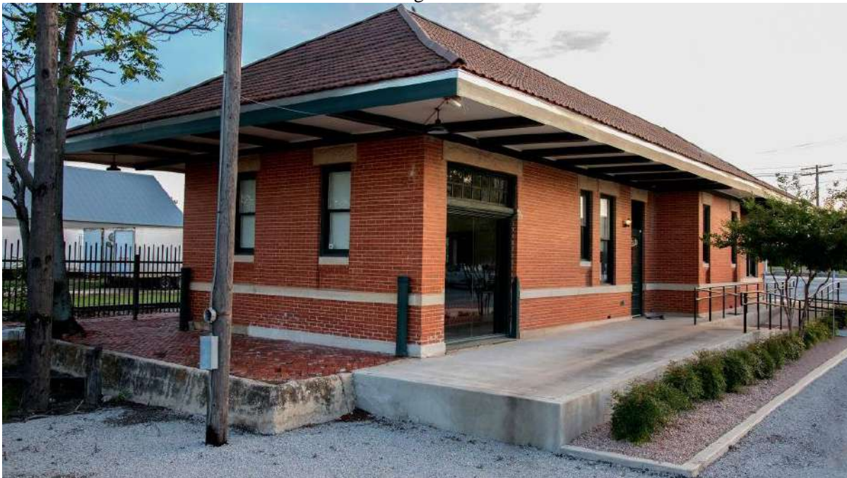
Photo 4: North and east elevations—camera facing southwest
