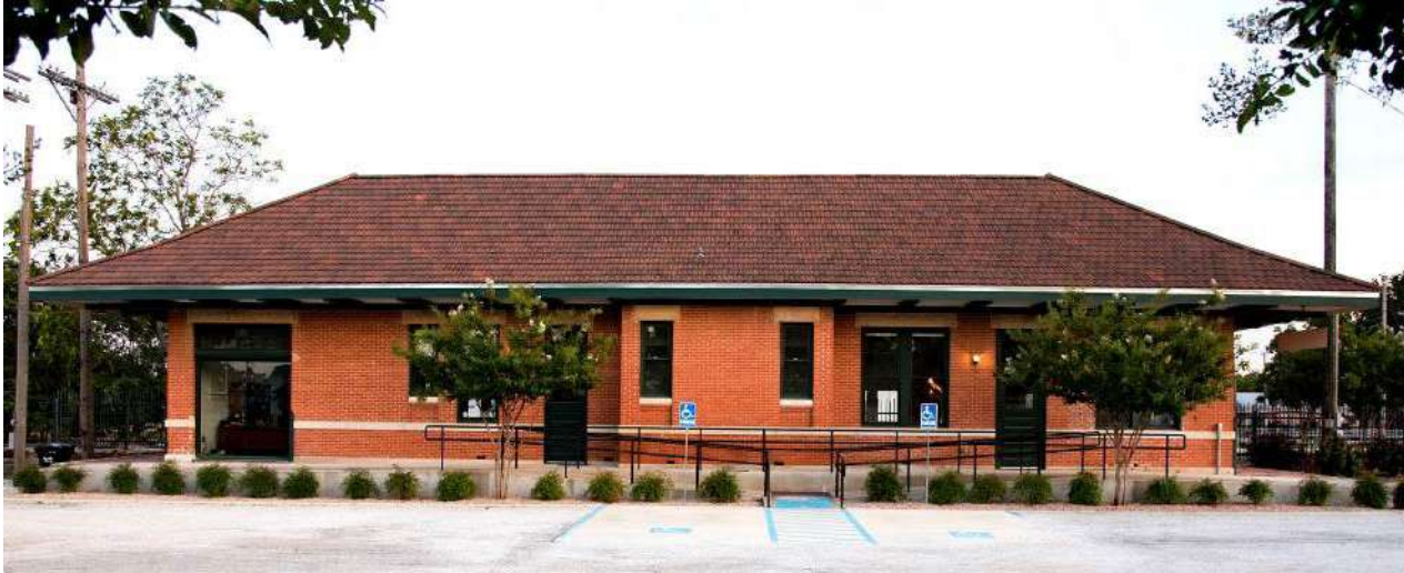
Photo 5: North elevation—camera facing south
