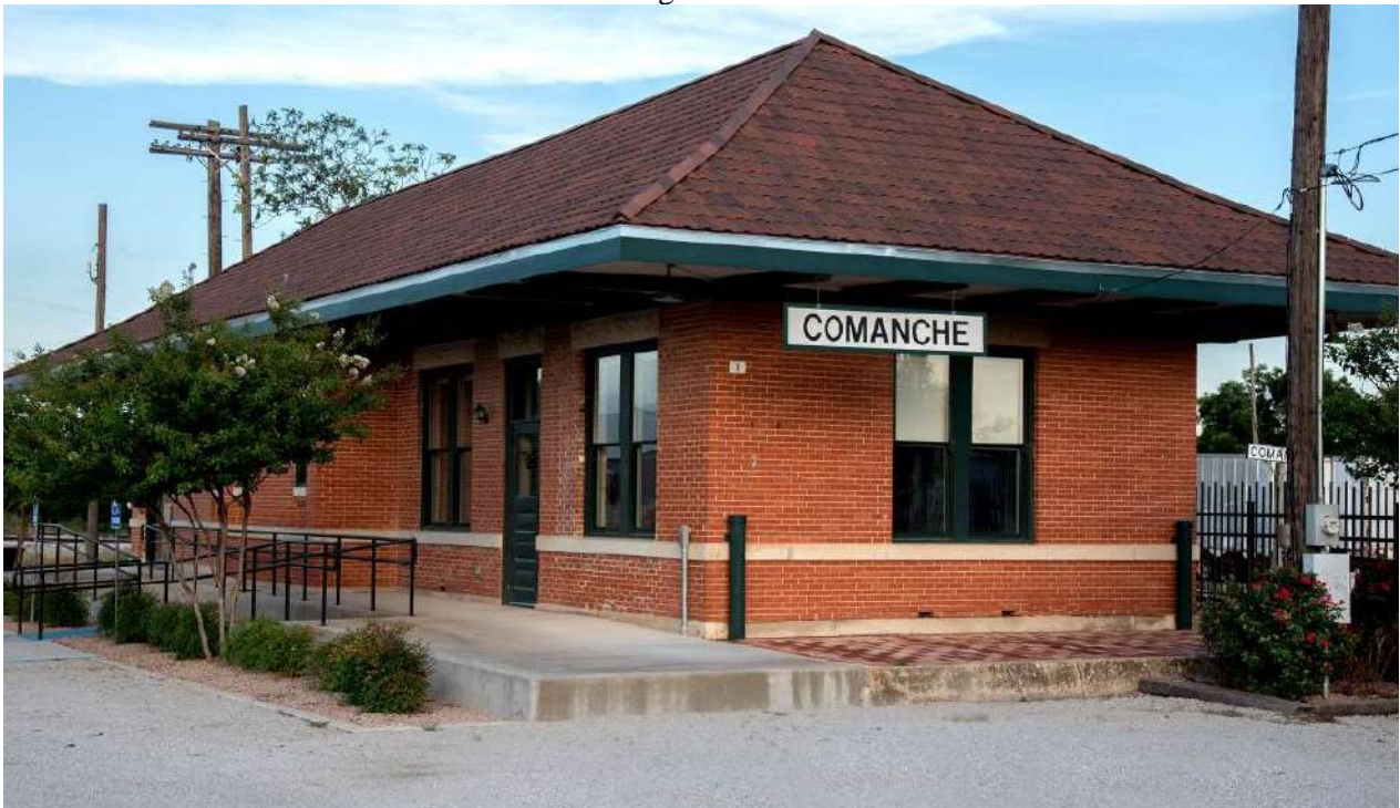
Photo 6: North and west elevations—camera facing southeast
