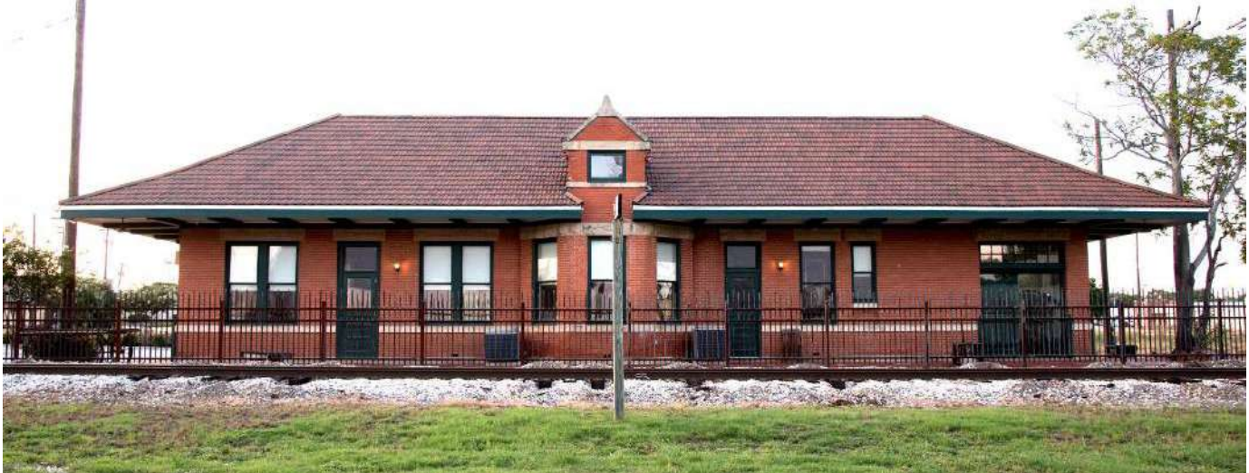
Photo 1: South elevation—camera facing north
