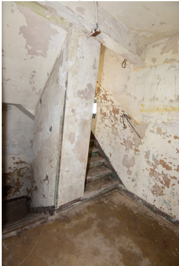
Photo 9 Second floor, staircase, view west
