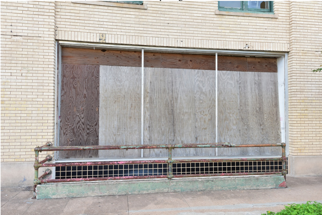
Photo 18. East elevation, detail of storefront opening and basement stair, view west, 2017.
