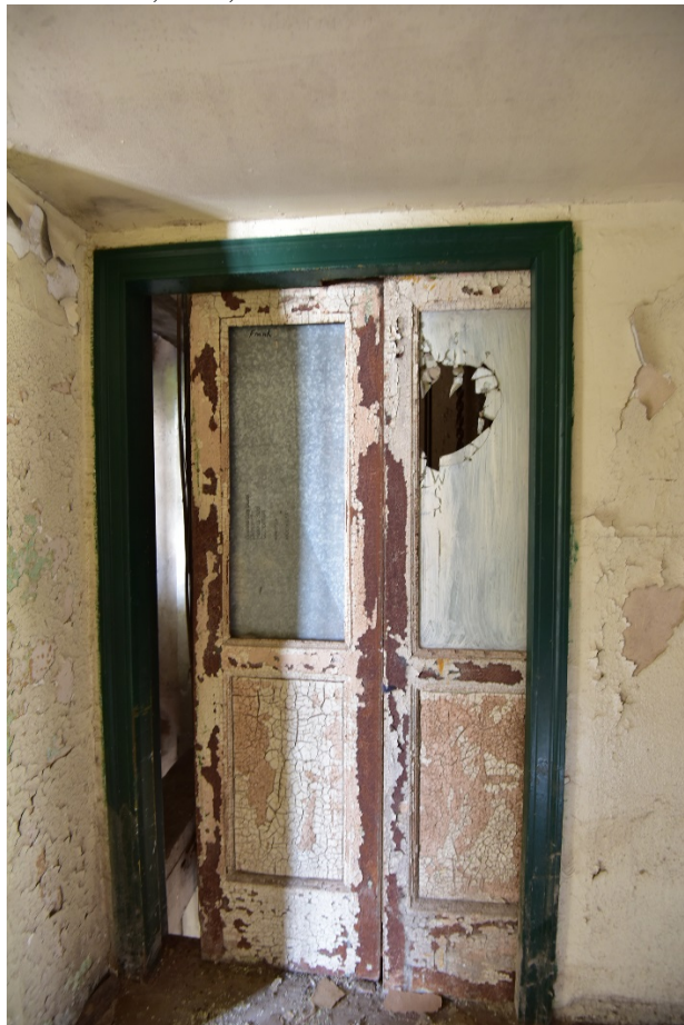
Photo 10 Third floor, door, view west
