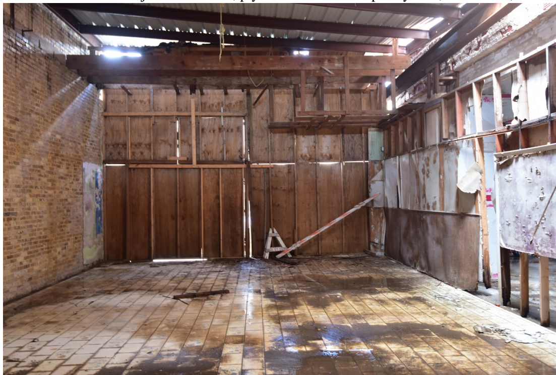
Photo 19. Interior of adjacent structure, plywood wall and temporary roof, view north, 2017.
