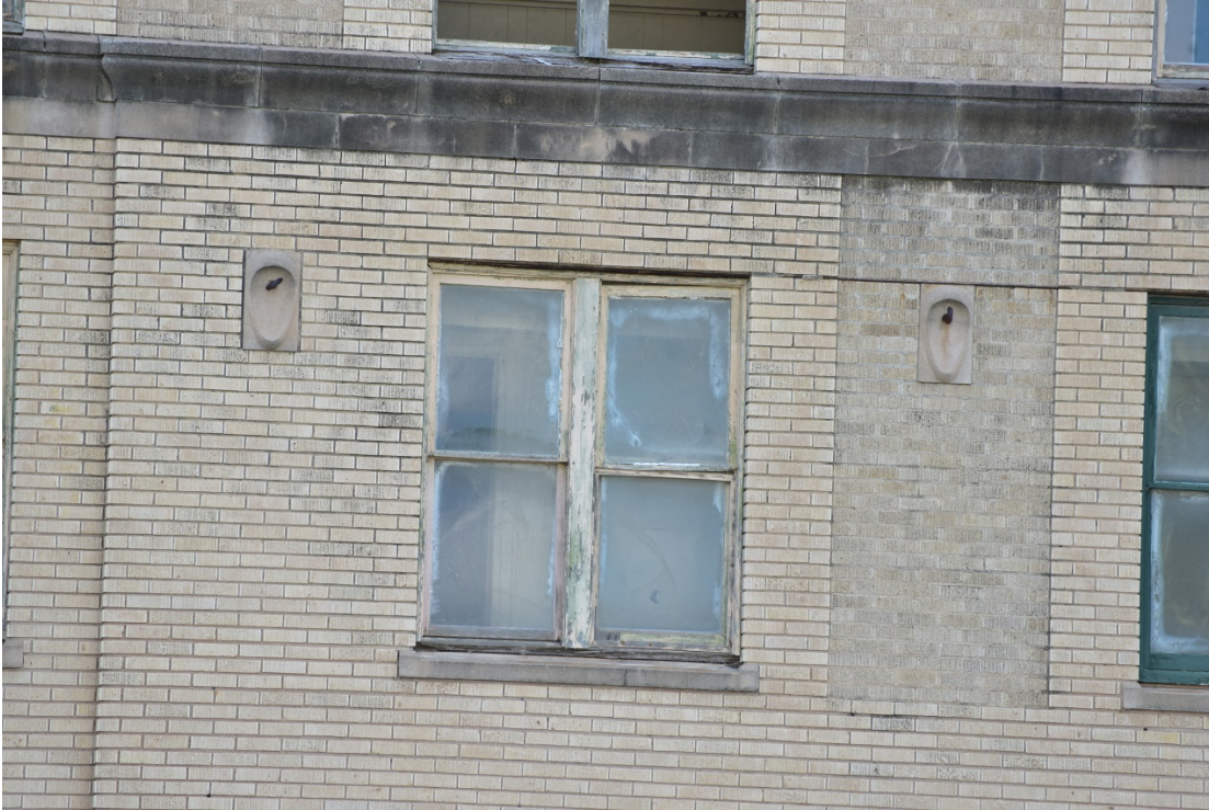
Photo 17. East elevation, detail of masonry canopy tie rod hooks, view west, 2017.
