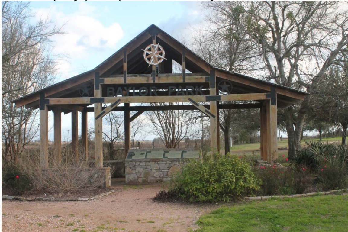
Photo 6: 2019 photograph of the pavilion (Non-contributing Resource 3), constructed in 2002, looking south.
