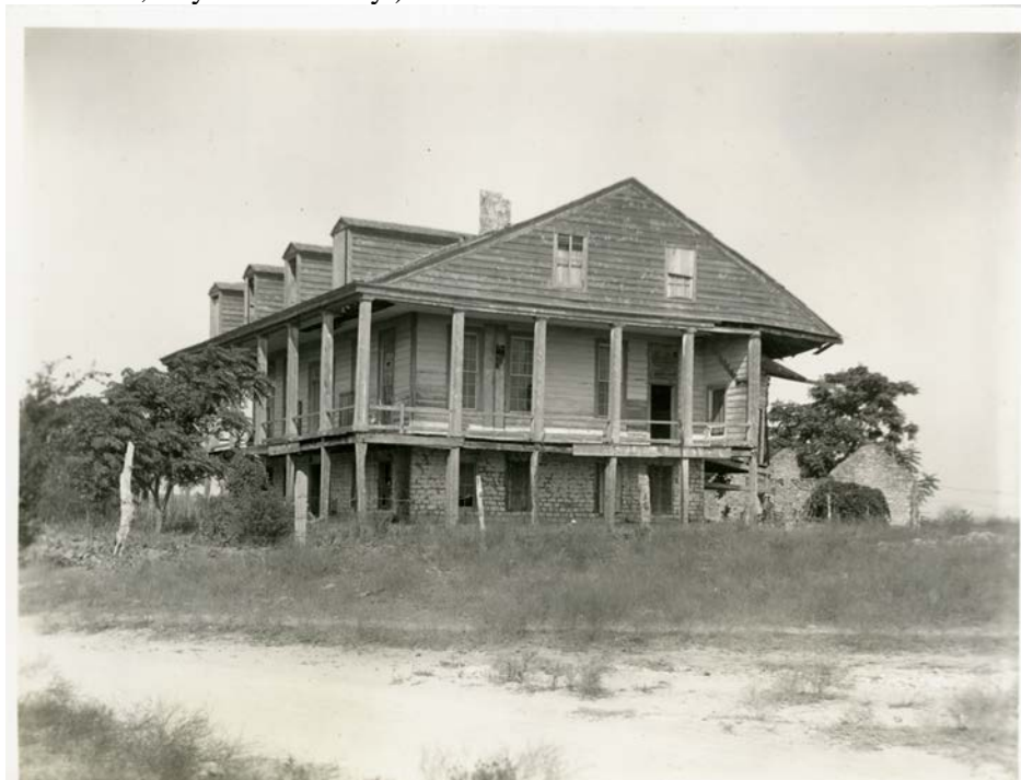
Figure 8: Boarding house in ruins, ca. 1920s-1930s. (BU Records: Photographs, Accession #22.01, The Texas Collection, Baylor University.)
