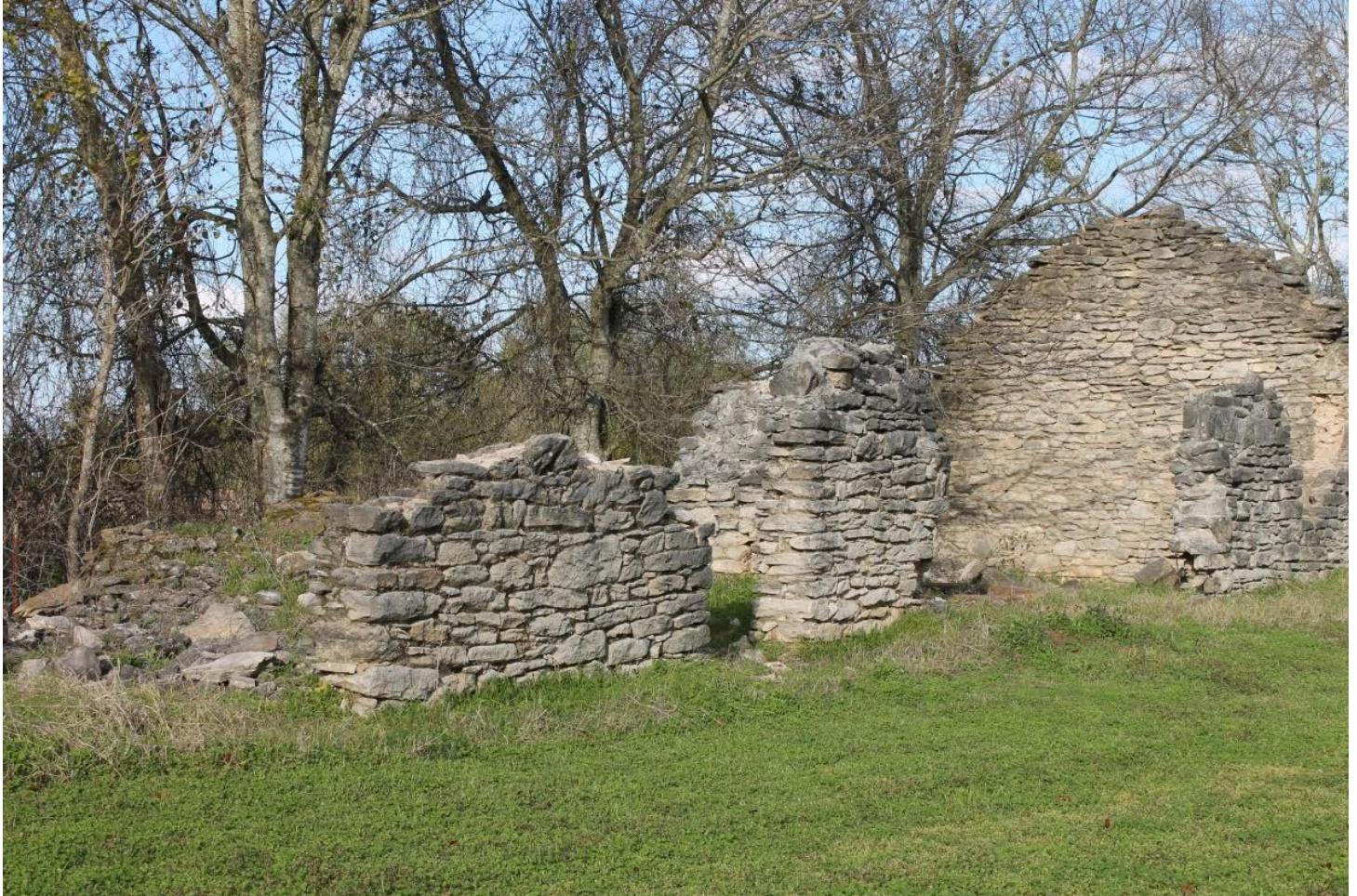
Photo 3: 2019 photograph of the kitchen duplex ruins, (Contributing Resource 1, Feature B) facing north.
