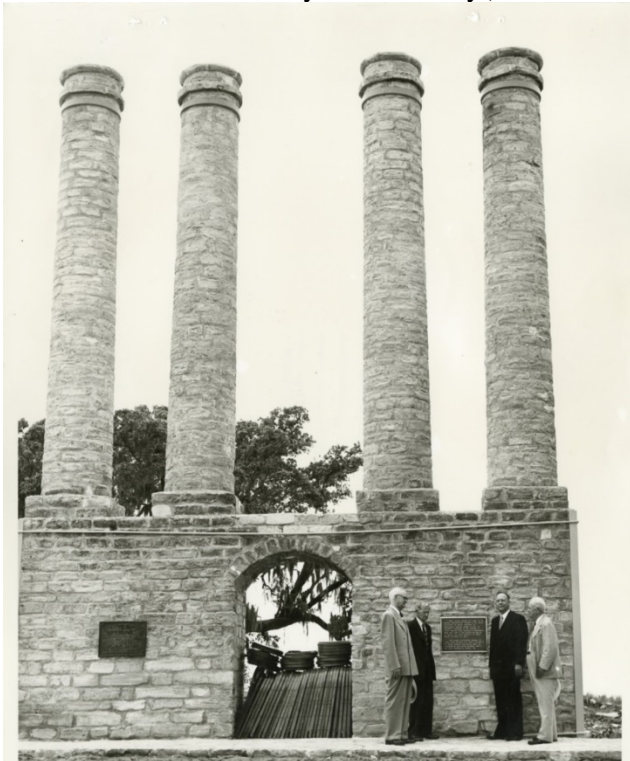
Figure 10: 1952 photograph of the academic building after stabilization. (BU Records: Photographs, Accession #22.01, The Texas Collection, Baylor University.)
