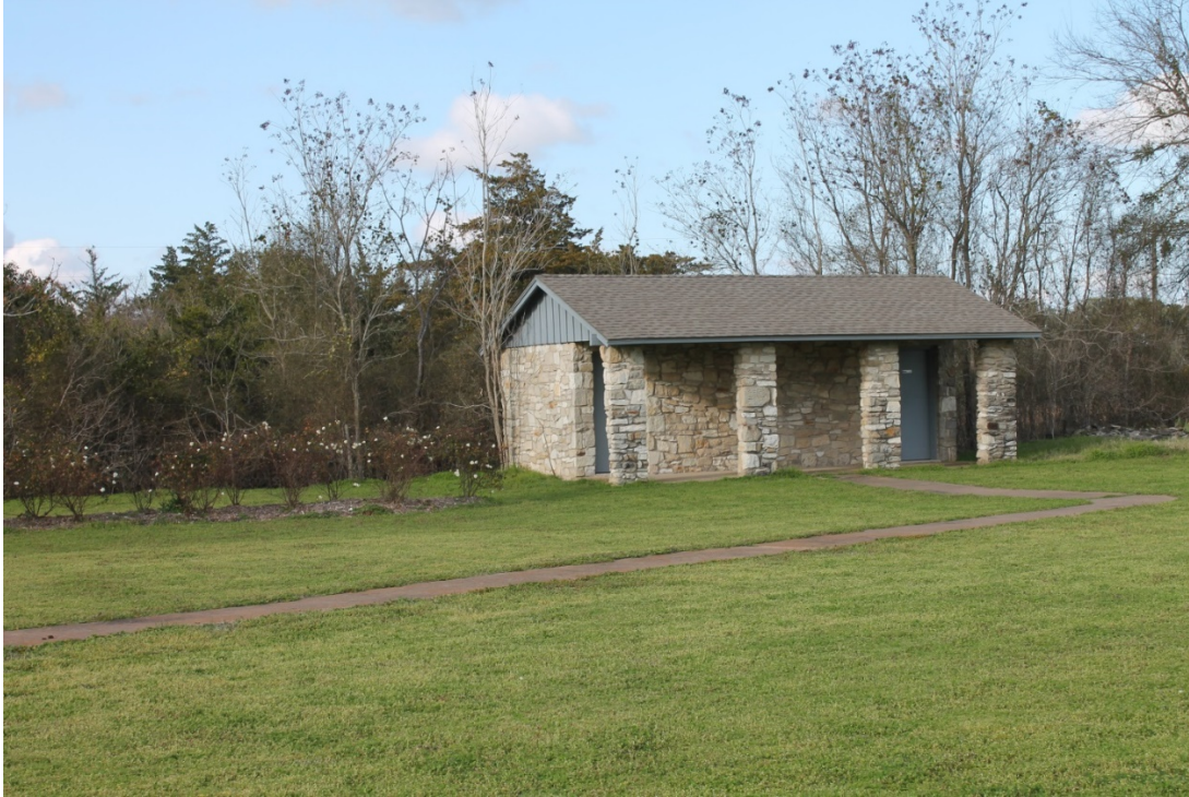
Photo 8: 2019 photograph of the possible location of the dining hall (Contributing Resource 1, Feature F), directly to the west (left) of the restroom, nooking north.
