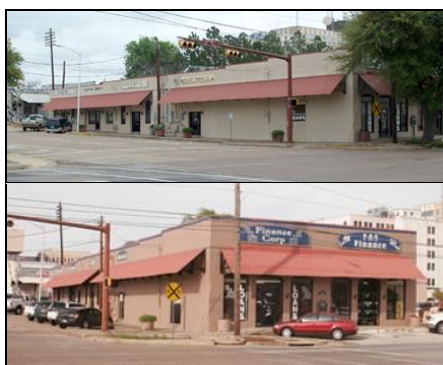
Before (top) and after (bottom): Longview’s first façade improvement grant in 2008 addressed sporadic plaster issues, windows, paint, and signage.
