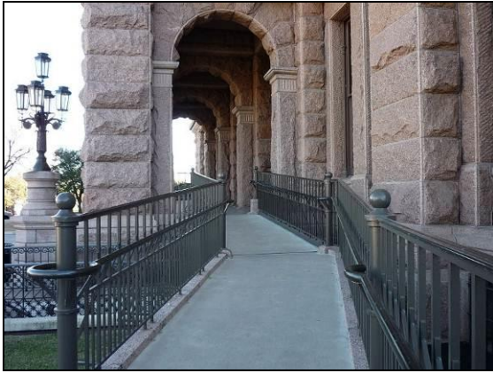
Accessibility ramp at the north entrance to the state capitol in Austin that fits into its environment through the careful use of color, materials, and ornamentation.
