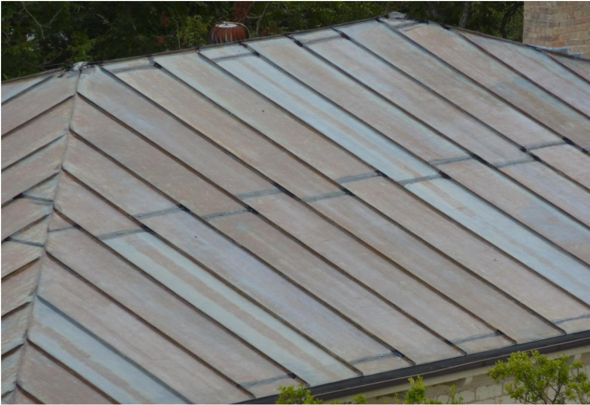
During 4, September 21, 2010, Photo taken from top of adjacent parking garage West side, Application of Karnack 89 Sta-Tack, note elastomeric sealant at joints
