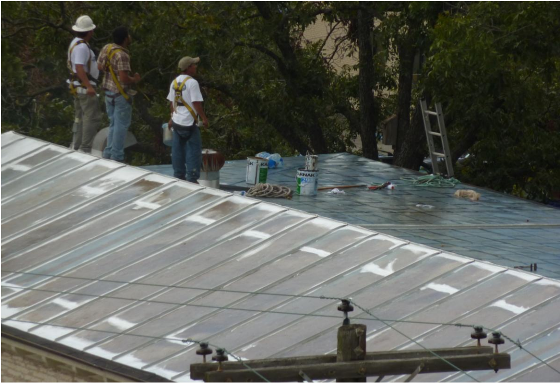
During 10, September 22, 2010, Photo taken from top of adjacent parking garage North side, Application of Karnack 298 Alum-R
