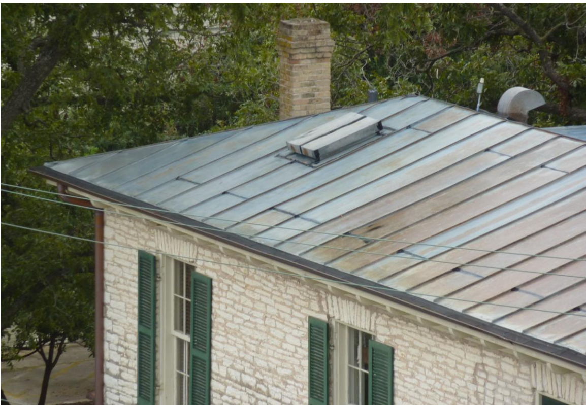
During 7, September 21, 2010, Photo taken from top of adjacent parking garage Southeast end, Application of Karnack 89 Sta-Tack, note elastomeric sealant at joints
