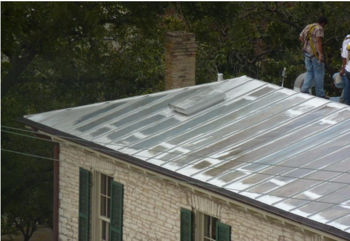
During 11, September 22, 2010, Photo taken from top of adjacent parking garage Northeast end, Application of Karnack 298 Alum-R
