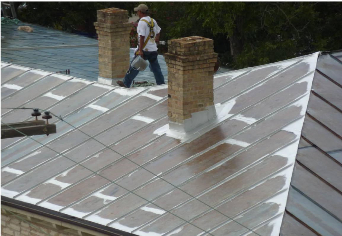
During 9, September 22, 2010, Photo taken from top of adjacent parking garage Northwest corner, Application of Karnack 298 Alum-R, note edges and joints done first
