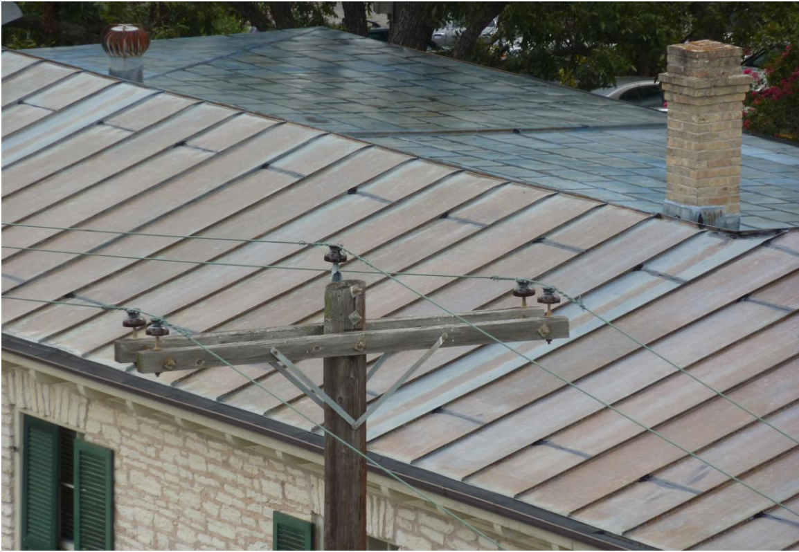
During 6, September 21, 2010, Photo taken from top of adjacent parking garage North side, Application of Karnack 89 Sta-Tack, note elastomeric sealant at joints
