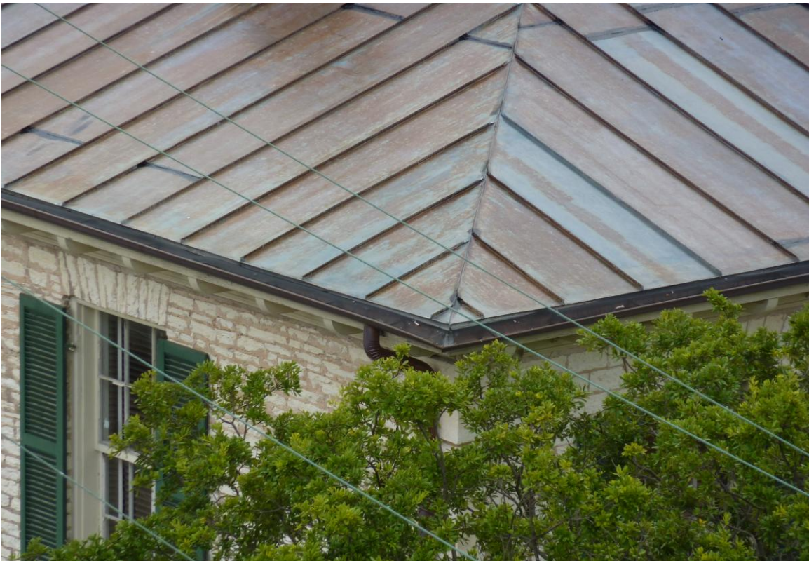
During 5, September 21, 2010, Photo taken from top of adjacent parking garage Northwest corner, Application of Karnack 89 Sta-Tack, note elastomeric sealant at joints
