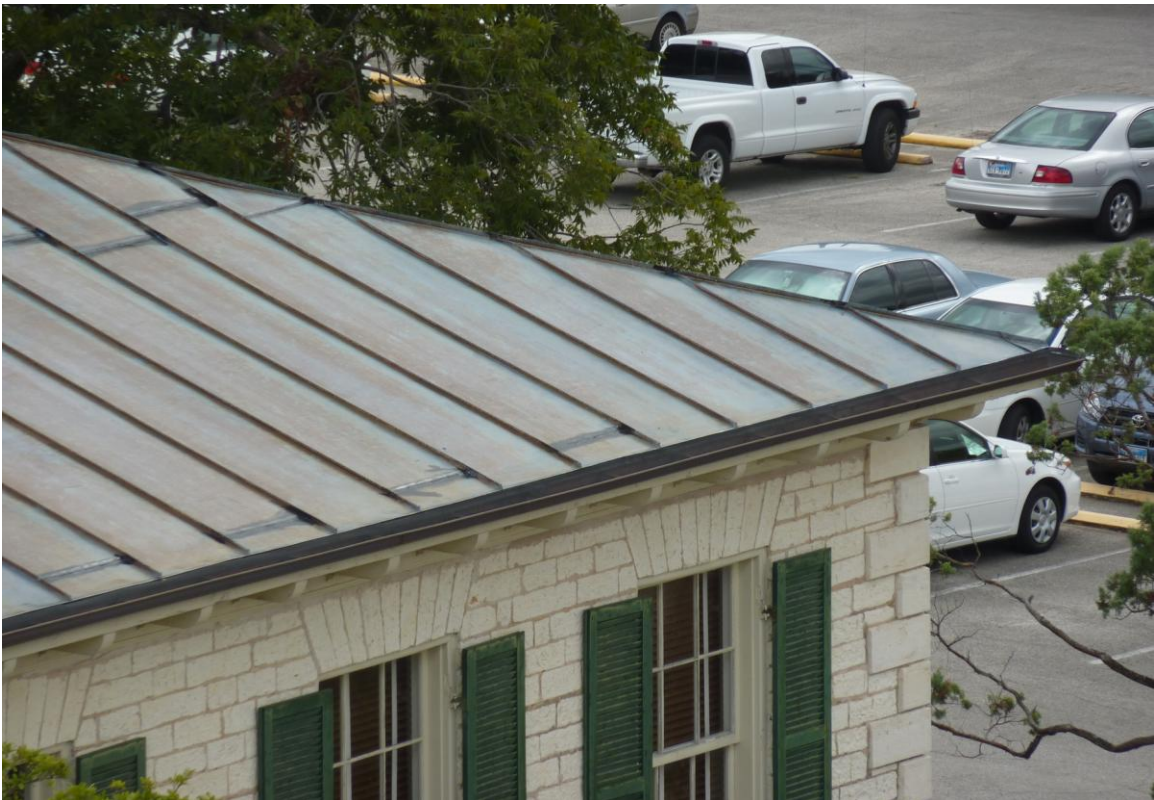
During 3, September 21, 2010, Photo taken from top of adjacent parking garage Southwest end, Application of Karnack 89 Sta-Tack, note elastomeric sealant at joints
