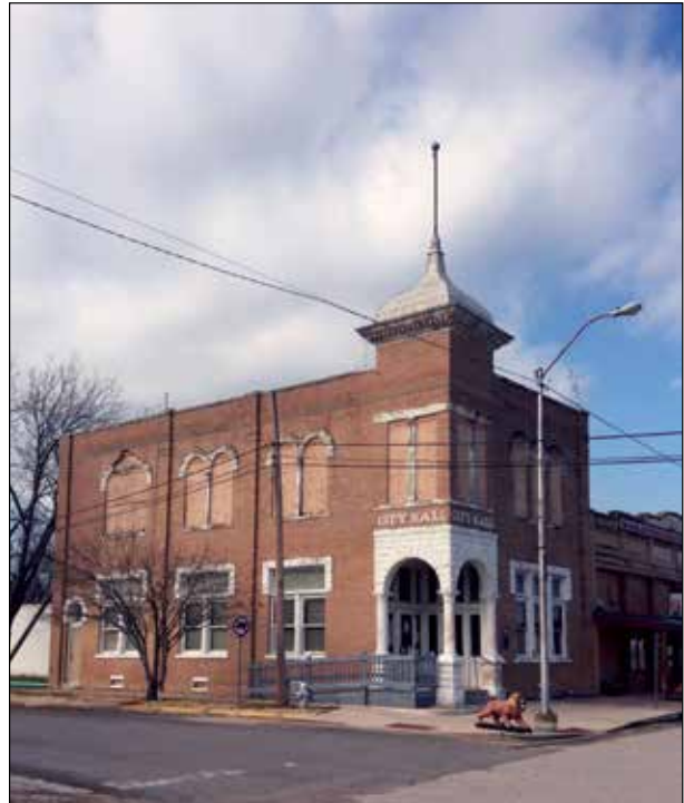
Granger City Hall, a Recorded Texas Historic Landmark, received a FY 2015 Texas Preservation Trust Fund planning grant for structural stabilization.
