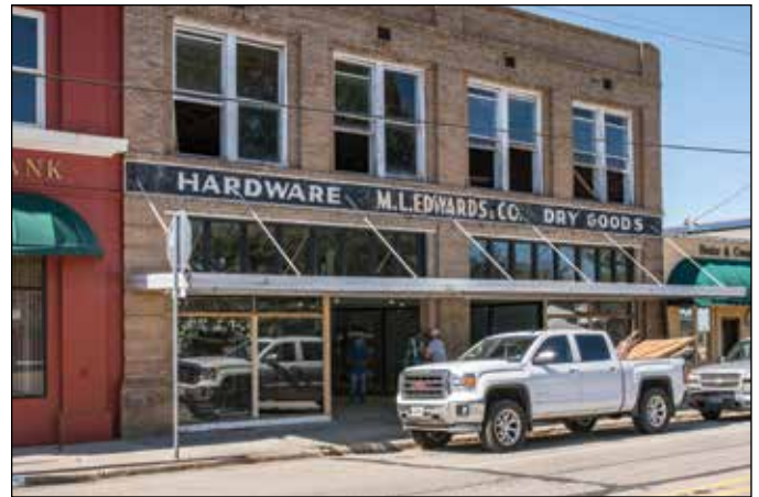
The M.L. Edwards Building in Mount Vernon (1916) once housed a hardware and general store. Through the state and federal tax credits, it has been rehabilitated into a retail shop and events venue.
