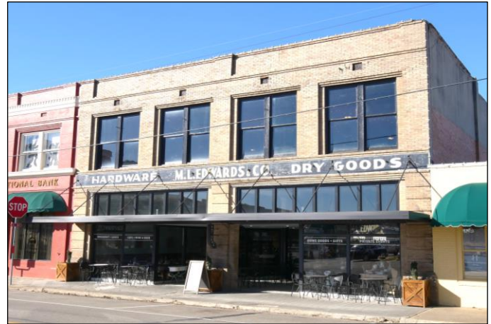
The M.L. Edwards Building in Mount Vernon (1916) once housed a hardware and general store. Through the state and federal tax credits, it has been rehabilitated into a retail shop and events venue.
