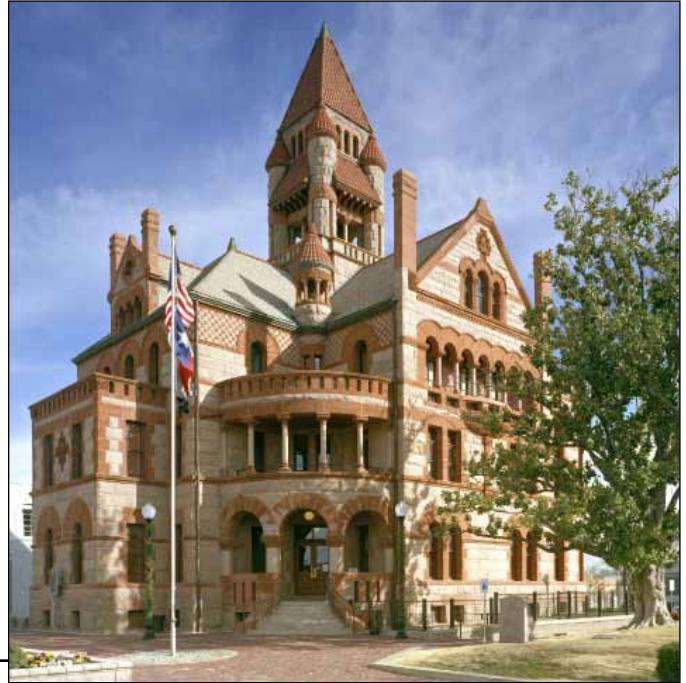
Hopkins County Courthouse
