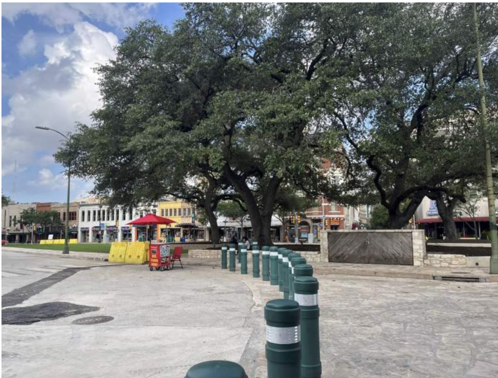
D - View from SW corner of Alamo arcade to SW at Plaza de Valero and future site of deck and shade structure. Note raised planters with heritage trees. Note electrical cabinet at front of raised plaza wall retained during interim condition.
