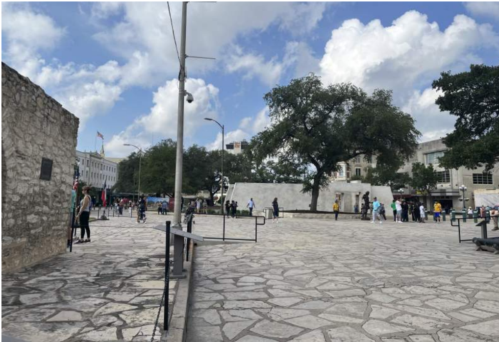
A - View from Long Barracks to the Mission Gate and Lunette exhibit. Note raised planters housing heritage trees in newly accessible zone of the plaza.
