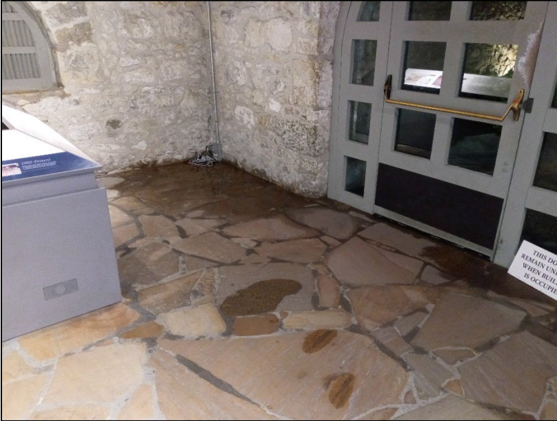
Figure 3. Northernmost room in the Long Barrack, near the exit door, facing northeast.
