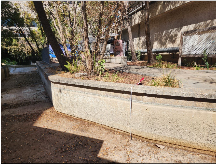
Figure 19. Photo of the depressed water feature at Lower Paseo, facing west.
