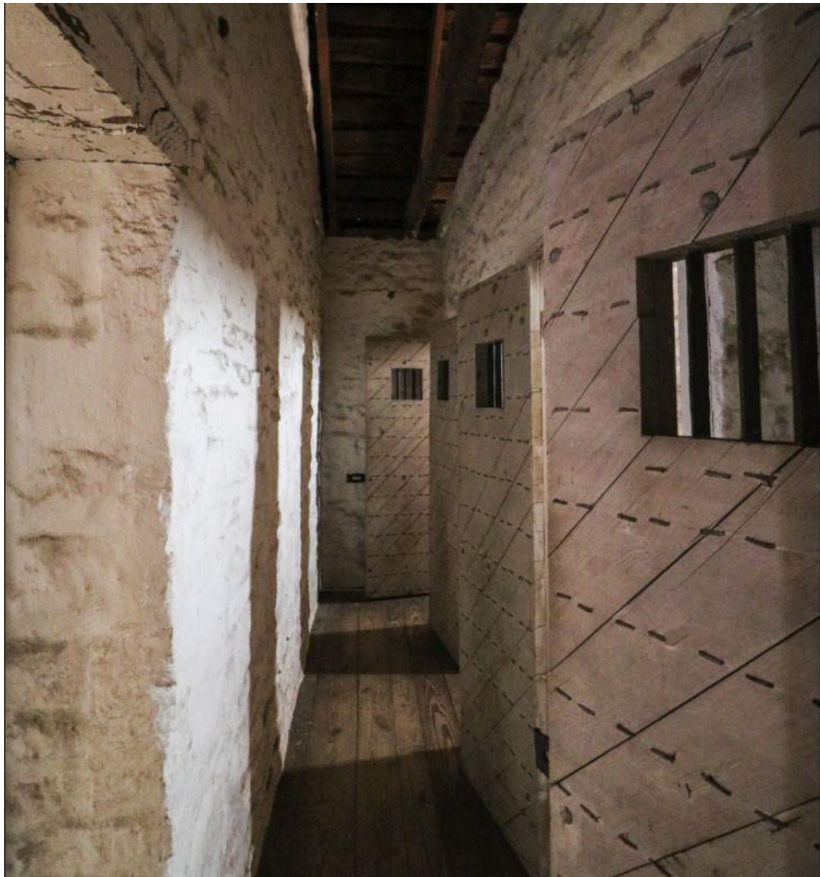
Figure 5 Jail Cells Located in Guardhouse
