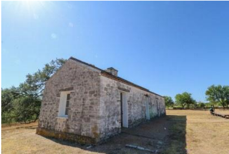
The Guardhouse is the only remaining original structure of the site
