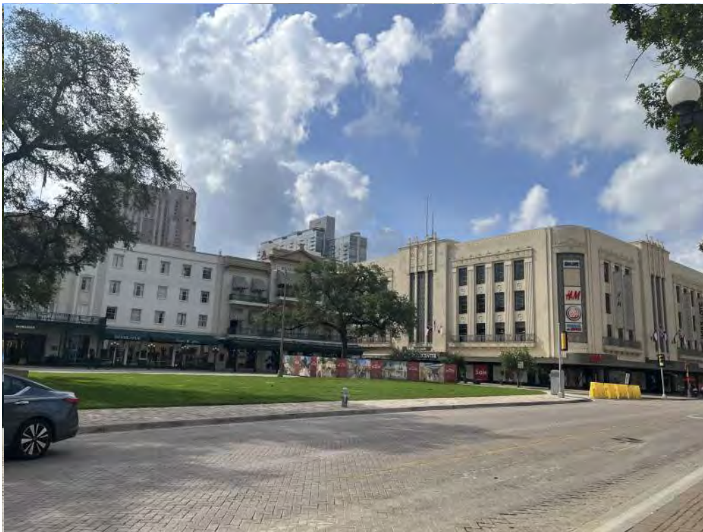
H - View from E Crockett to Plaza de Valero temporary event lawn. Note contained heritage tree protected by fencing and windscreen in anticipation of transplanting during full build condition.
