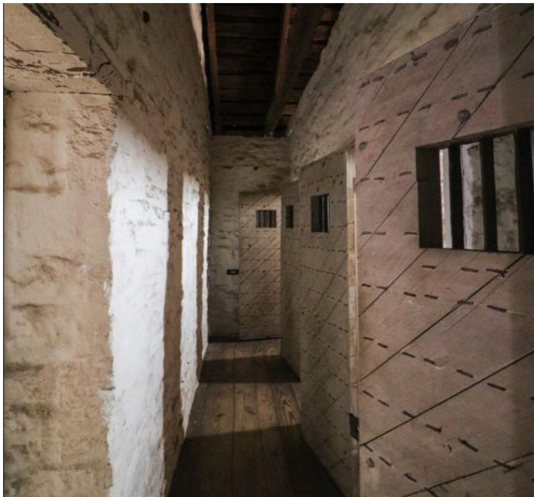
Figure 4. Jail Cells Located in Guardhouse
