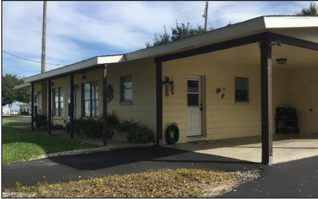
Harbor Lights Cottages, front and side (north and west respectively) elevations, facing east-southeast.
