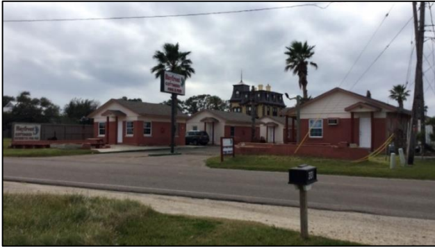
Bayfront Cottages, front and sides (east) elevations facing west-southwest.
