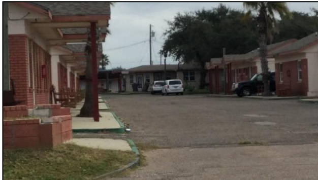
Bayfront Cottages, front and side (east) elevations, facing west-northwest.
