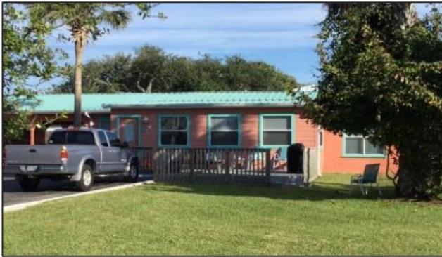
201 Palmetto Avenue, front (south) elevation, facing north.
