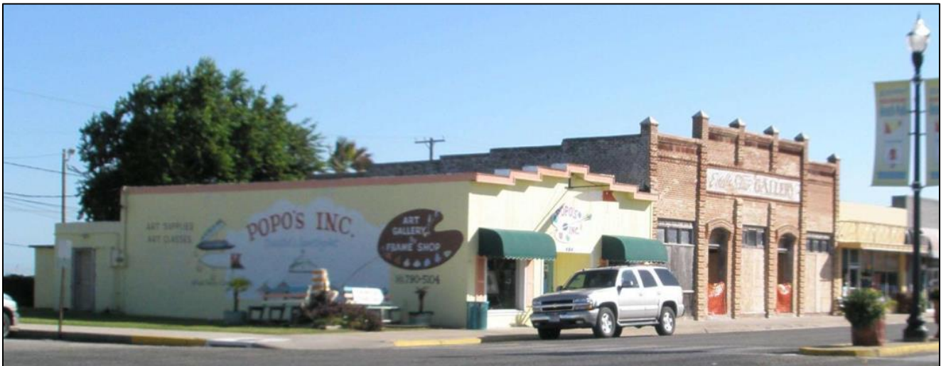
Figure 14: View of the Sorenson-Stair Building, a commercial building that functioned historically as a chandlery, a grocer, and is presently an art gallery (Texas Historical Commission 2007a).
