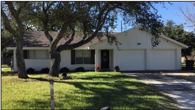
917 Oak Ave, Rockport, façade, facing west.
