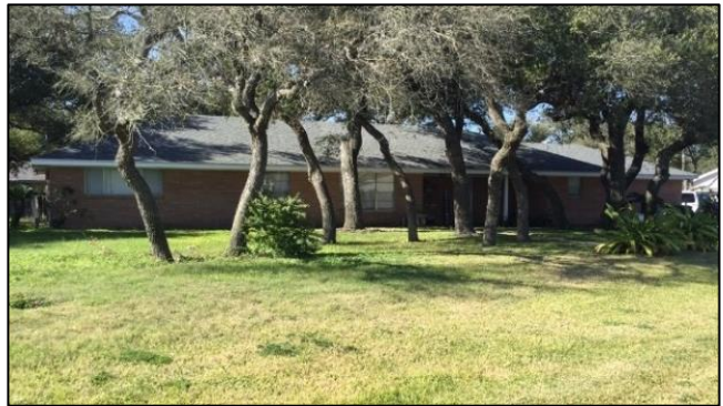
705 Oak Ave, Rockport, façade, facing west.
