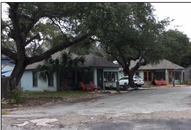
Fulton Beach Bungalows, front/side (south) elevations, facing north.
