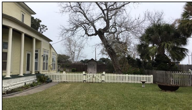
The dwelling at 902 East Cornwall Street is an 1881 Queen Anne style house. Now used as a bed and breakfast, the building retains its wood cladding including wood siding and patterned shingle and plank siding in the front gable,
