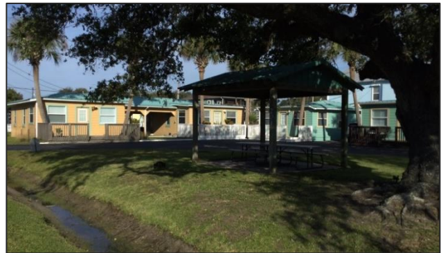
201 Palmetto Avenue, front (east) elevation and picnic shelter, facing west-northwest.
