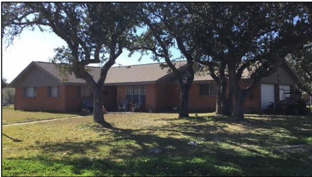
1005 Oak Ave, Rockport, façade and side elevation (southeast and northeast respectively), facing west.
