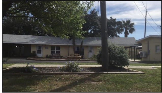
Harbor Lights Cottages, front and partial side of two buildings (north and east respectively), facing south.
