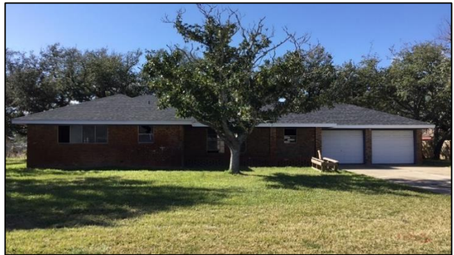
927 Oak Ave, Rockport, façade, facing west.
