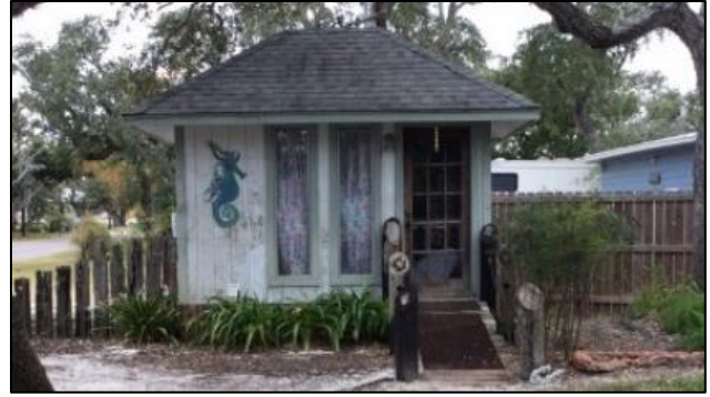
Fulton Beach Bungalows, front (east) elevation, facing west.
