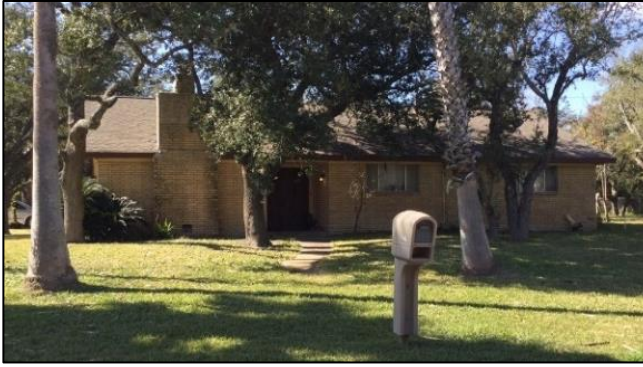
705 Pine Ave, Rockport, façade, facing west.
