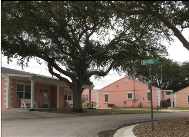
Sea Gunn Bay Homes, front and side of several cottages (south and west respectively) elevations, facing east-northeast.
