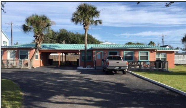
201 Palmetto Avenue, front (south) elevation facing north.
