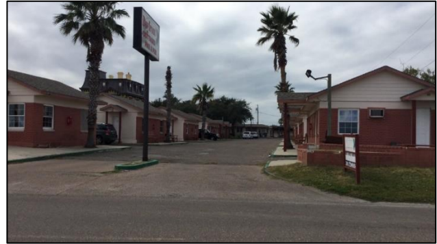
Bayfront Cottages, front (east) elevation, facing west.
