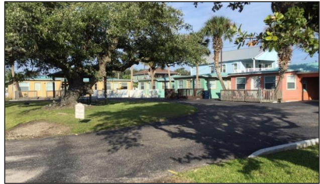
201 Palmetto Avenue, front (south and east) elevations of several cottages, facing north-northwest.
