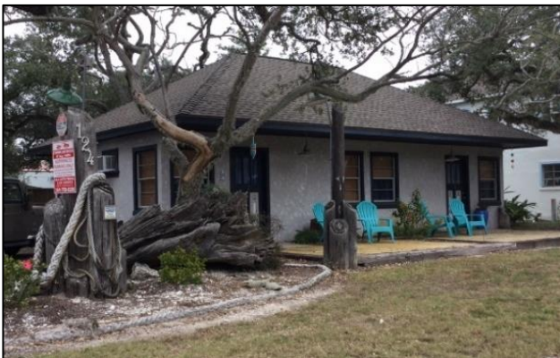
Fulton Beach Bungalows, front (south) elevation, facing north-northeast.
