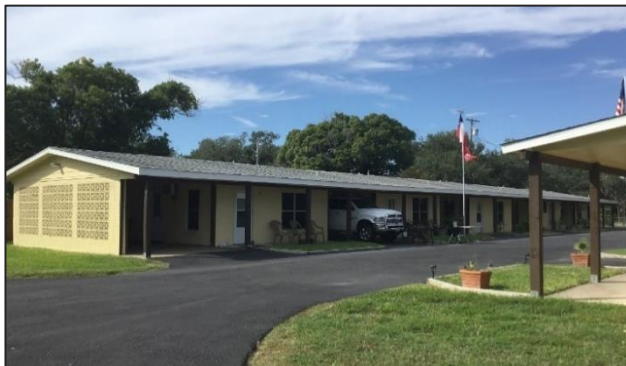
Harbor Lights Cottages, front and side (east and south respectively) elevations, facing north-northwest.
