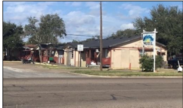
Cedar Lodge Motel, front (southwest) elevation and side (southeast) elevation facing north-northwest.
