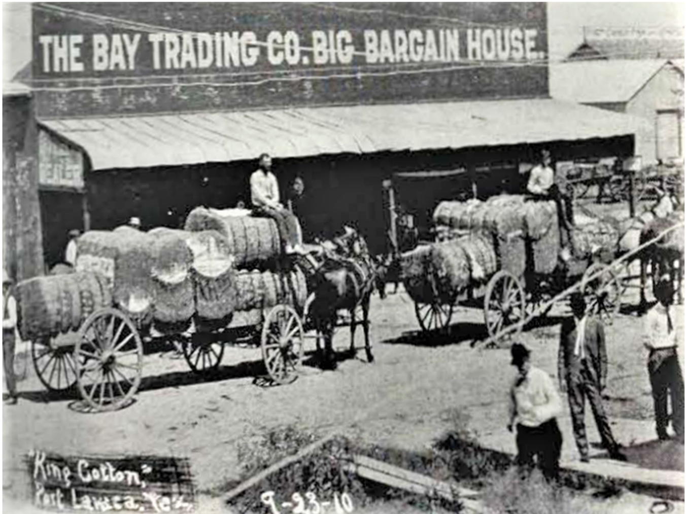
Figure 29. Horse-drawn drays with burlap-wrapped cotton bales are parked outside the one-story wood-frame Bay Trading Company's Big Bargain House, at the northeast corner of Main and Colorado Streets, in September 1910. The building's full-width porch had a metal-clad shed canopy with a false parapet above (Johnstone 2002b, 2:8). T. A. McKamey, W. T. Moore, and Roy Miller owned the company which purchased most of the cotton local farmers raised and traded general merchandise. This was the eventual location of the Ed Melcher Company (Johnstone 2016; 31, 166).
