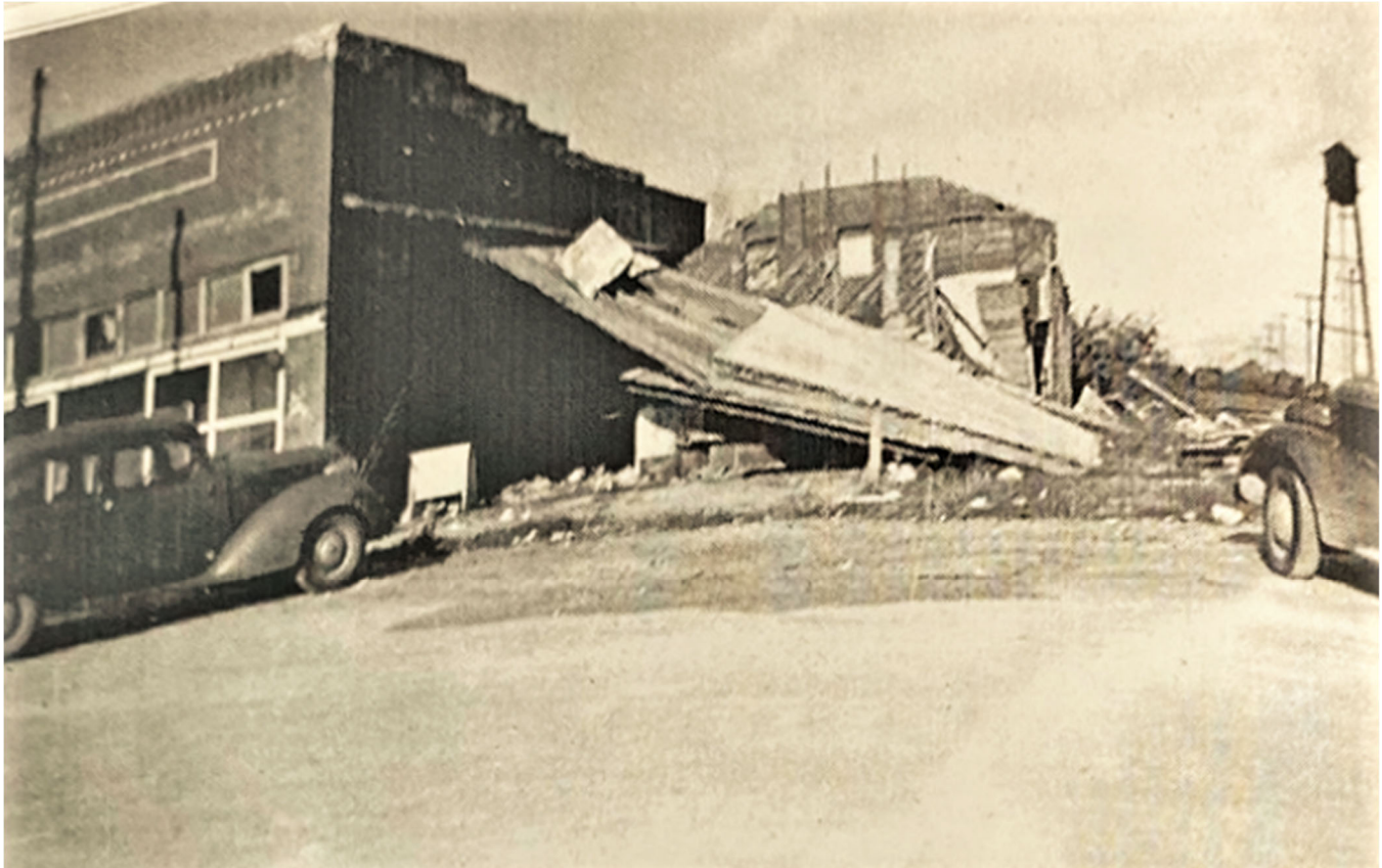
Figure 31. After the 1942 storm, masonry buildings (left) suffered window, door, and roof damage, and more-fragile wood-frame buildings (center) were destroyed. The precariously spindly metal water tower (far right) however, survived (Johnstone 2003b, 4:46).
