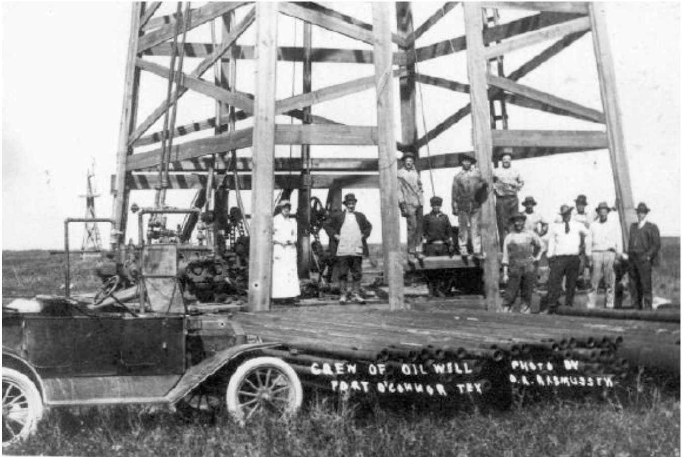
Figure 46. Visitors and oil field roughnecks pose in this undated image of a temporary wood derrick built for oil exploration near Port O'Connor (Johnstone 2016, 7).
