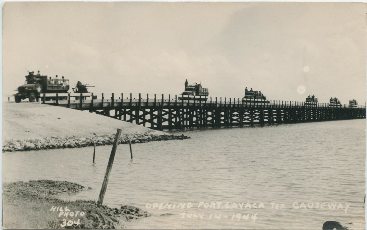
Figure 72. This 1944 image shows the State Highway 35 causeway, reopened after hurricane damage repair (Anonymous 1944).
