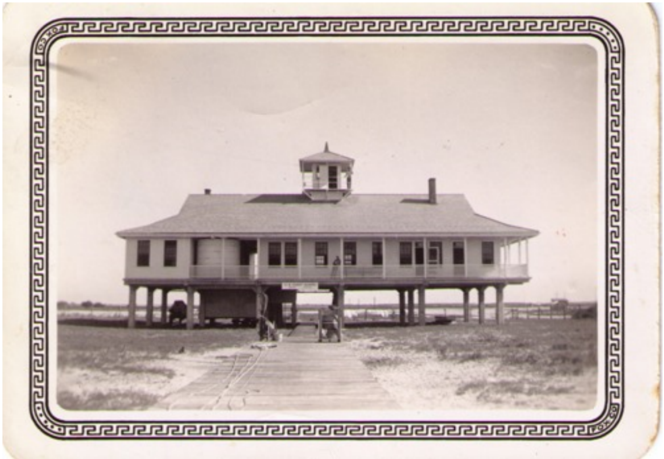
Figure 57. This 1932 image of the U.S. Coast Guard Station at Saluria shows the lifted building with its central lookout cupola (U.S. Coast Guard Heartland 2020).
