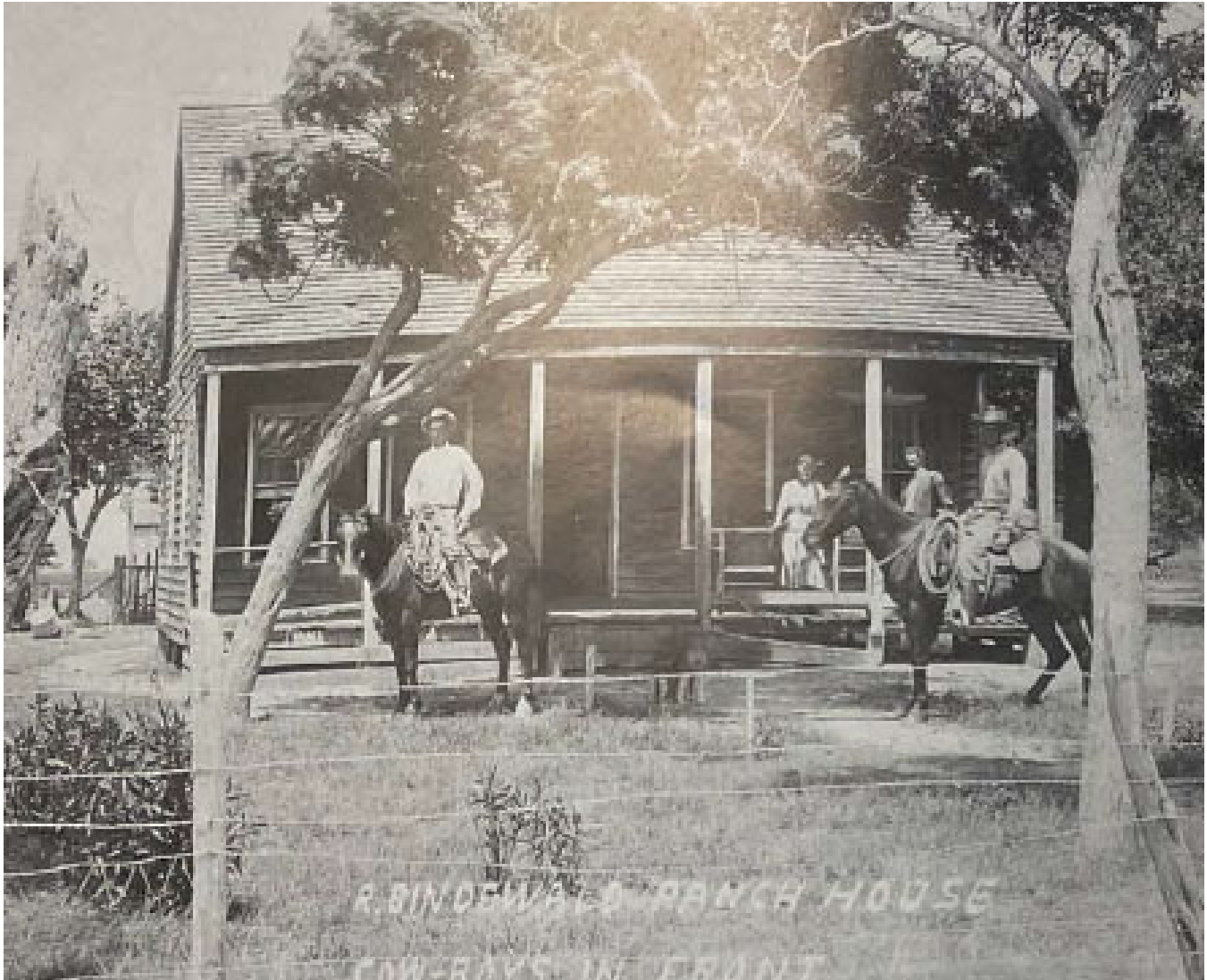
Figure 24. This undated image shows two cowboys in front of the Bindewald ranch house, where a woman is seated on the front porch. The wood-frame side-gable house has an integrated full-width porch with a shed roof. The house has horizontal clapboard siding and a pair of double hung windows on either side of the center front door. A barb-wire fence protects the domestic yard (Seadrift History Book Committee 2012, 108).
