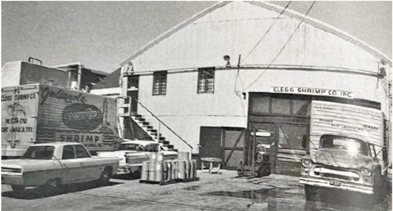
Figure 43. Although door, window, and some cladding materials have been replaced, the fenestration pattern on the Clegg Shrimp Company's southwest façade at the Municipal Harbor has changed little from its original configuration based on this undated image (Johnstone 2005, 96).
