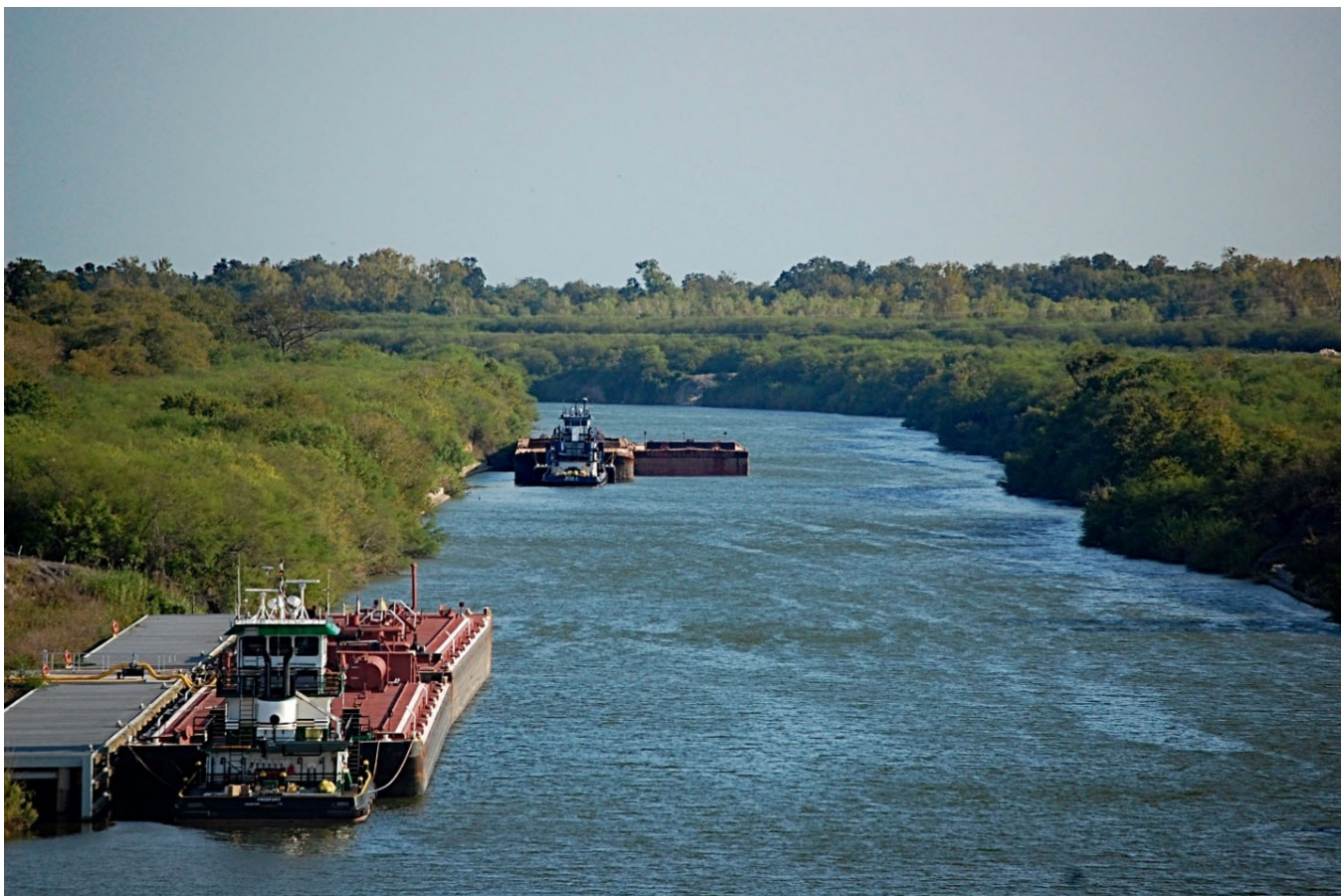
Figure 38. This current view of the 35-mile-long Victoria Barge Canal shows its present-day 125-foot width (Port of Victoria 2021).
