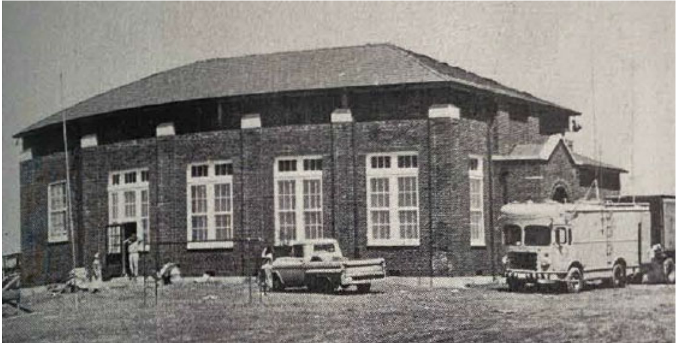
Figure 49. This 1962 image shows the 1936 PWA-sponsored Port O'Connor School after Hurricane Carla. The storm badly damaged the school, but it was repaired and is still in use. It may be the earliest extant school in the county (Johnstone 2002c, 3:51).
