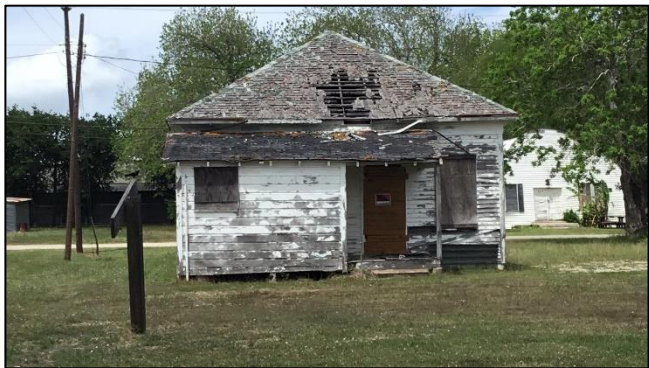
106/120 Austwell Road, rear (south) elevation; facing north.
