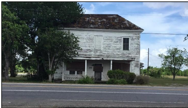
102 Austwell Road, side (west) elevation; facing east.
