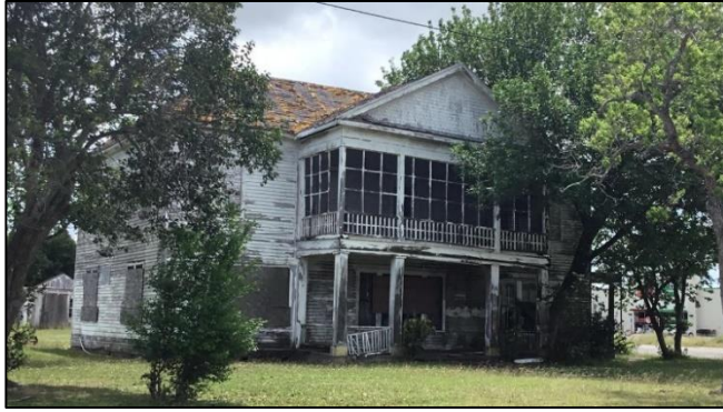
102 Austwell Road, front elevation; facing southwest.
