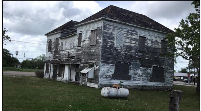
102 Austwell Road, side (east) elevation and rear (south) elevations; facing northwest.
