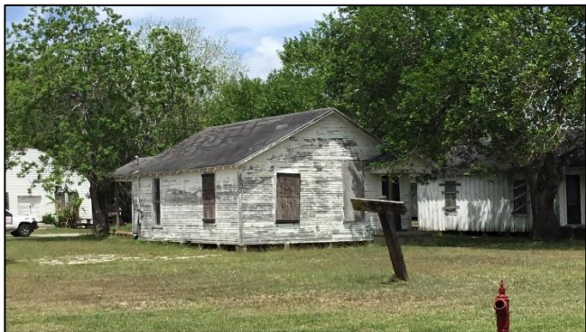
118 Austwell Road, rear (south) and side (west) elevations; facing northeast.
