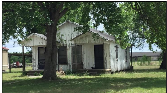
108 Austwell Road, front (north) and side (west) elevations; facing south.
