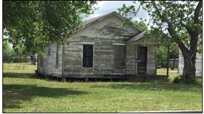
118 Austwell Road, front (north) and side (west) elevations; facing south.
