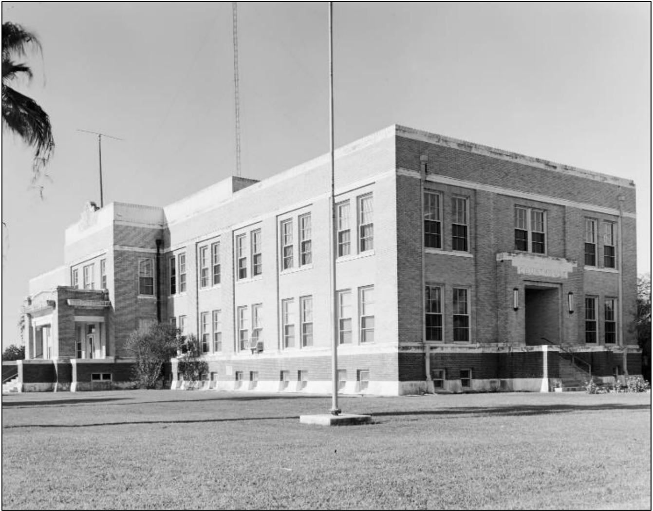
Figure 9: The Refugio County Courthouse (located at Courthouse Square), was constructed in 1917 and designed by San Antonio architect Atlee B. Ayers. The north wing, seen here, was extended in the 1950s dating to the photograph to after the 1950s. (Texas Historical Commission n.d.).
