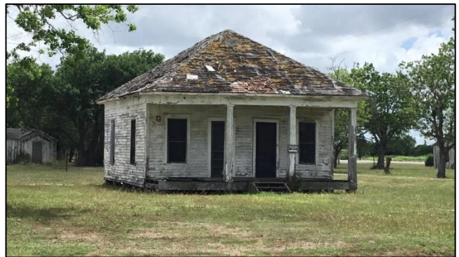
106/120 Austwell Road, front (north) and side (east) elevations; facing south.
