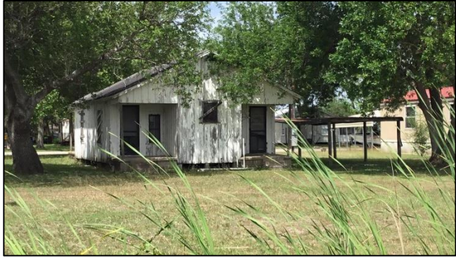
108 Austwell Road, rear (south) elevation; facing northeast.
