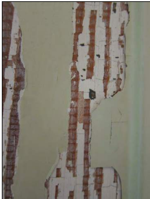
Figure 6: Dining room north window trim paint layers.
