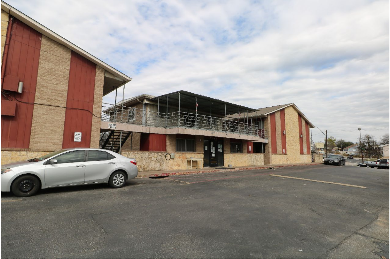
Photo 2: Exterior View, South Elevation of Office Building, Looking Northeast.
