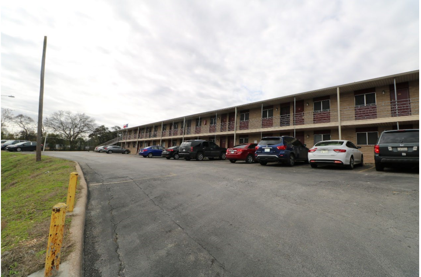
Photo 4: Exterior View, East Elevation, Looking Southwest.
