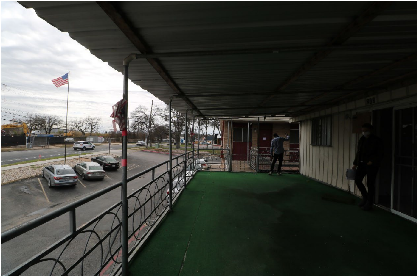
Photo 10: Exterior View, Office Building, Second Floor, Looking West.
