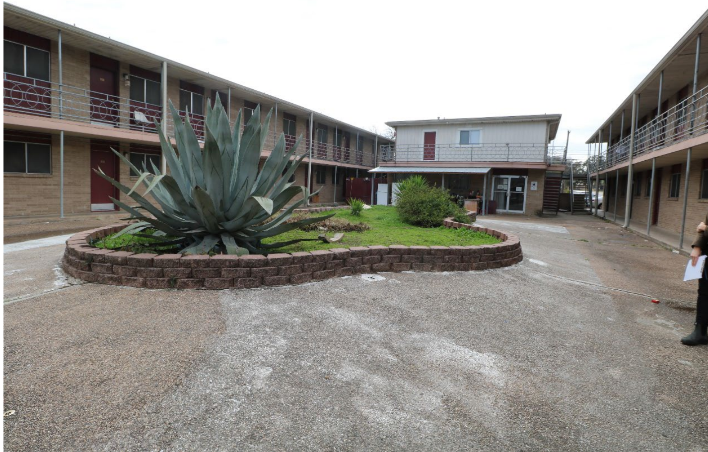
Photo 9: Exterior View, Courtyard, Looking Southeast.
