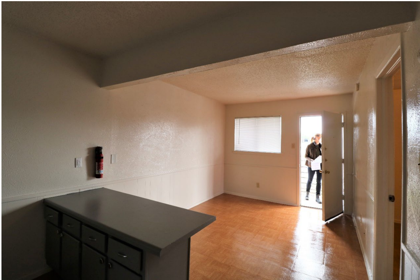
Photo 16: Interior View, Unit 241, Looking Northeast.
