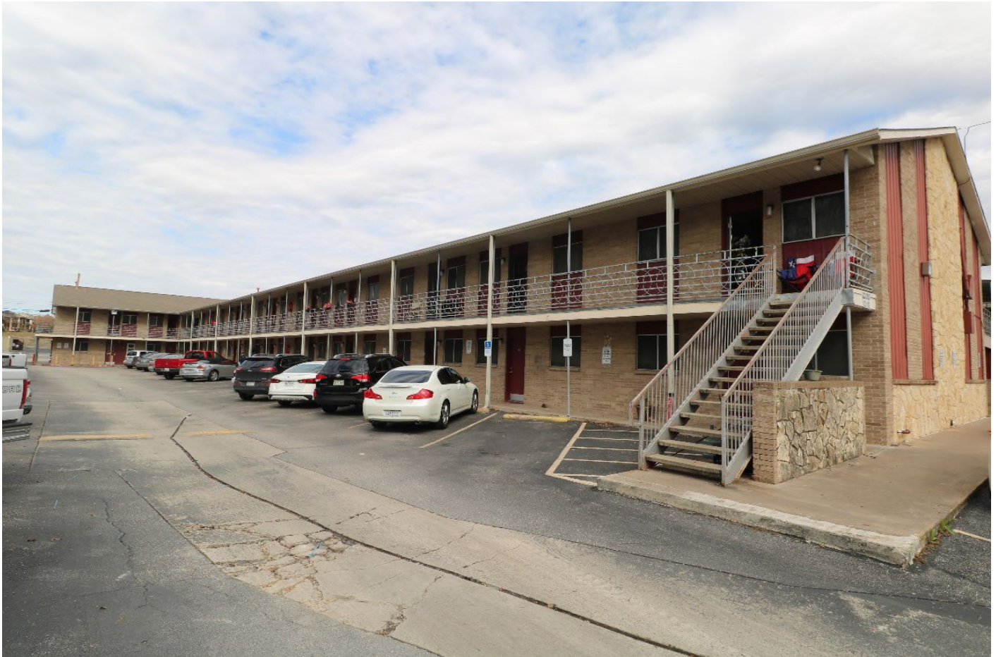
Photo 7: Exterior View, West Elevation, Looking Northeast.
