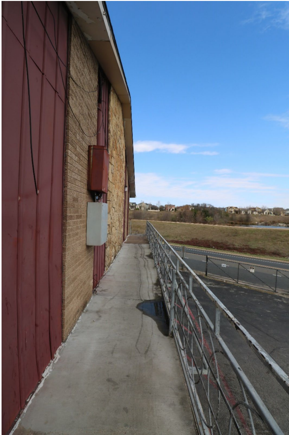
Photo 5: Exterior View, East Elevation, Looking North.
