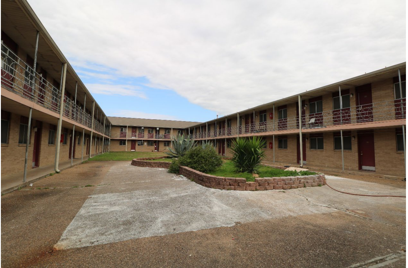
Photo 8: Exterior View, Courtyard, Looking North.
