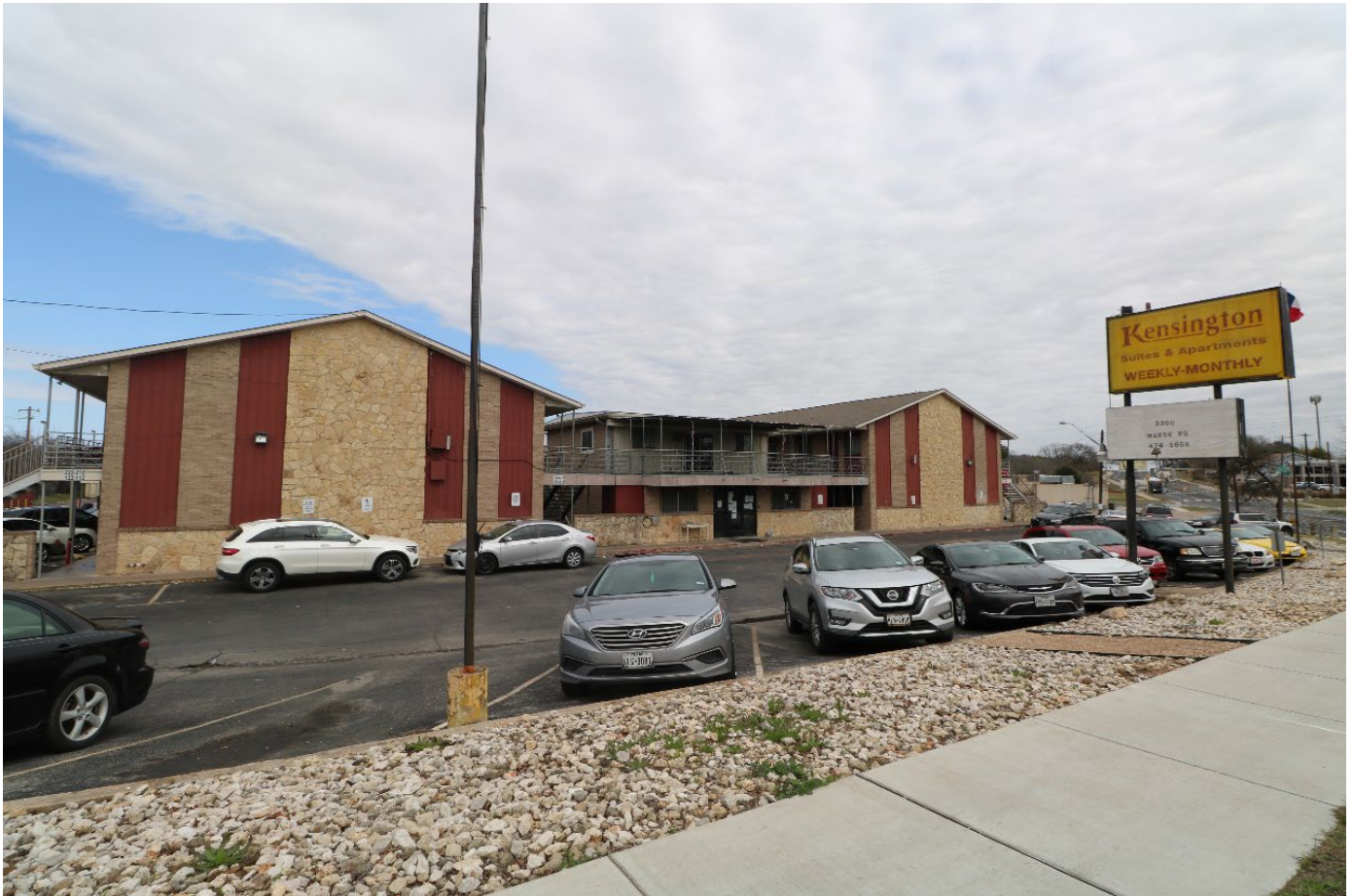
Photo 1: Exterior View, South Elevation, Looking Northeast.
