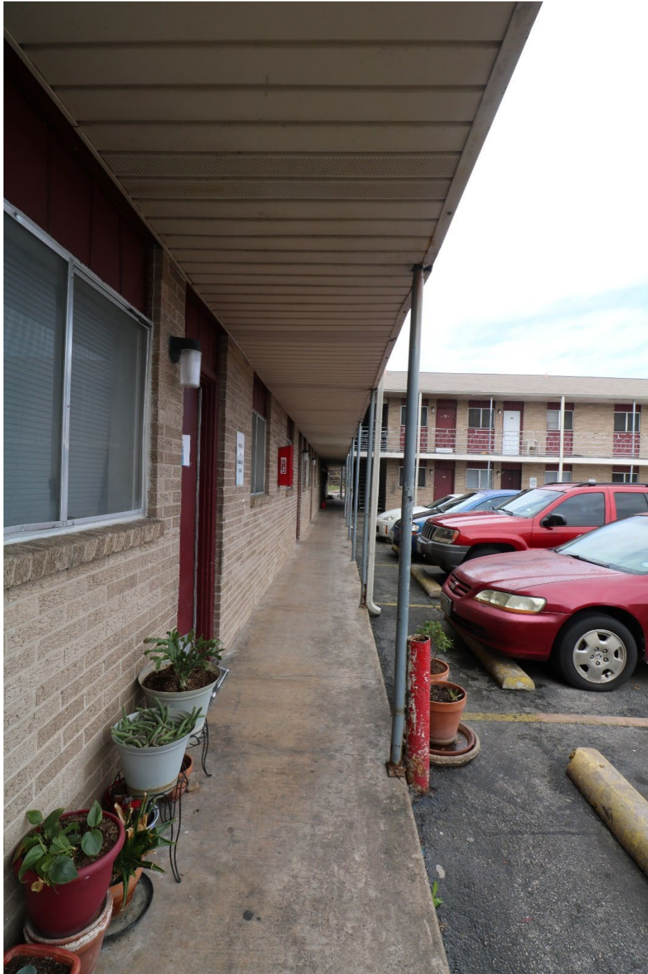
Photo 6: Exterior View, East Elevation, Looking West.
