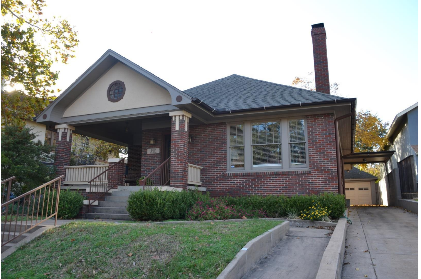
Photo 45. Photograph of 802 Rio Grande Street, facing west, 2019. Photo by HHM.
