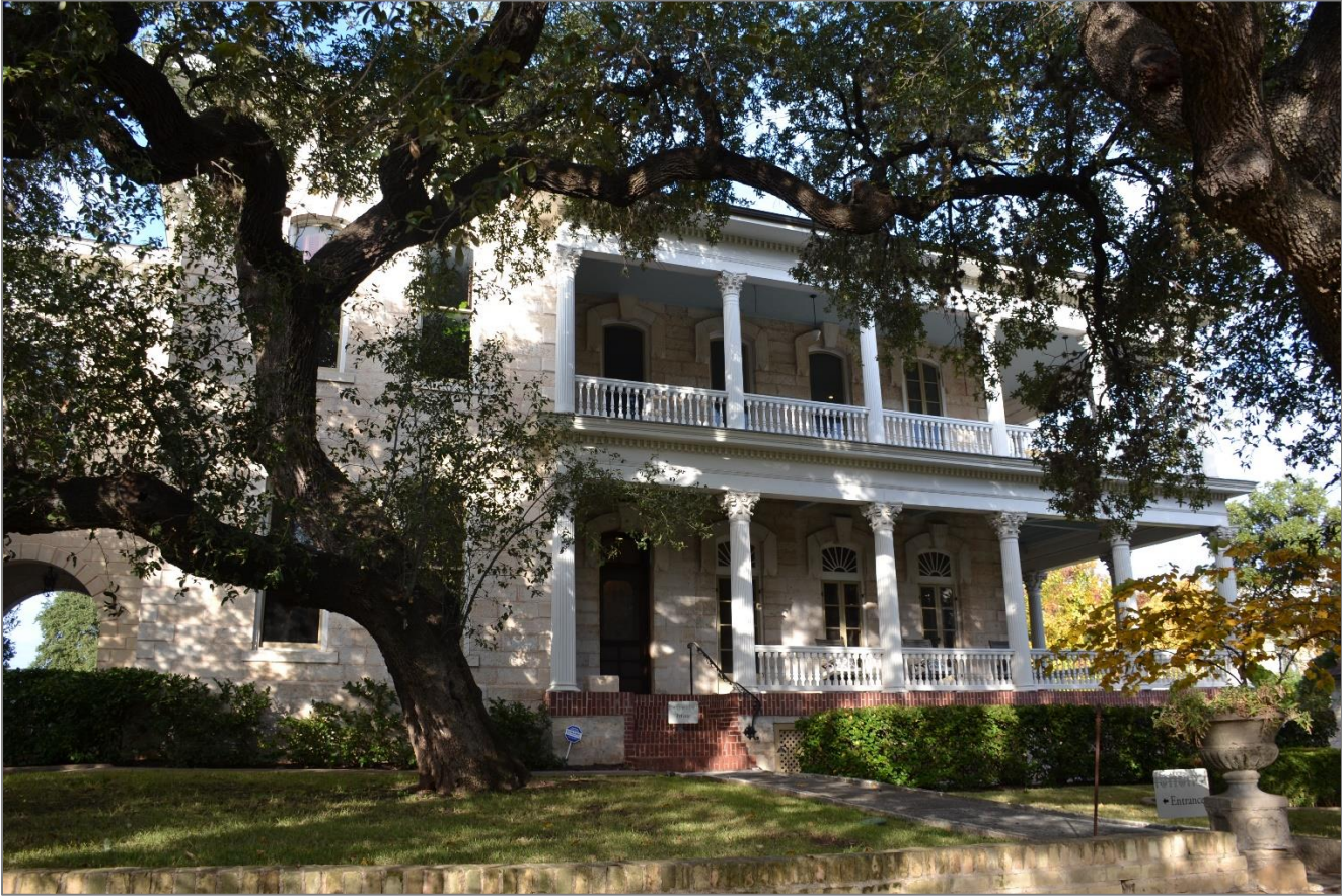
Photo 15. Photograph of the south-facing façade of 1003 Rio Grande Street, facing north by northeast, 2019. Source: HHM.
