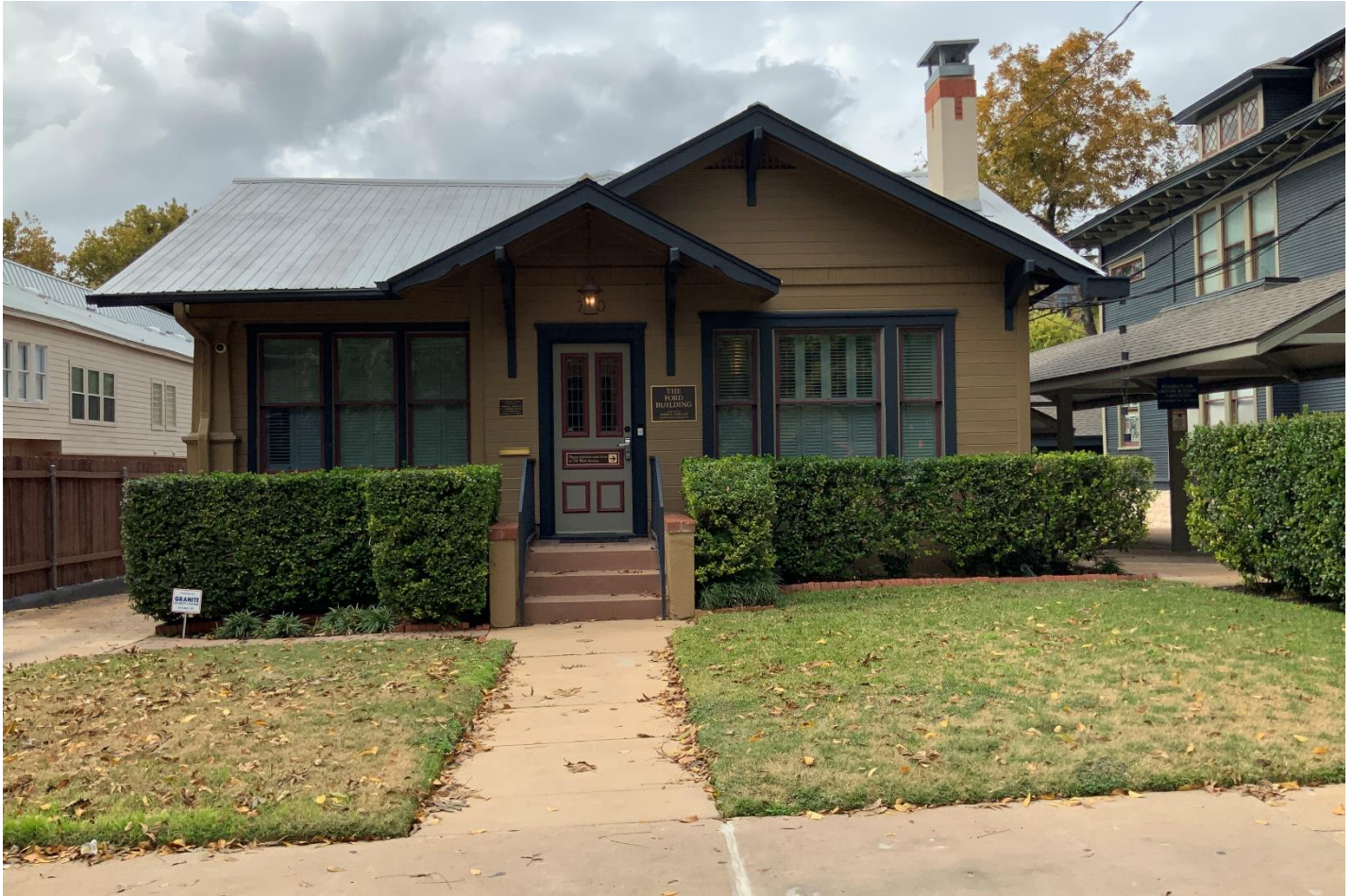
Photo 47. Photograph of 710 West Avenue, facing west, 2019. Photo by HHM.
