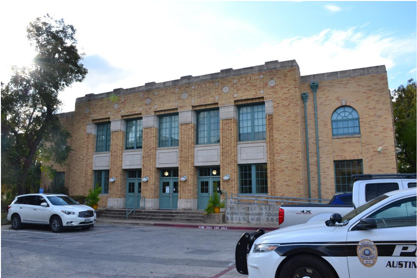
Photo 41. Photograph of 1218 West Avenue, facing west, 2019. Photo by HHM.
