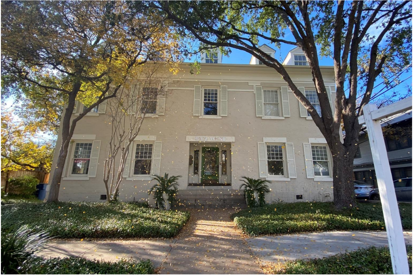
Photo 39. Photograph of 1002 West Avenue, facing west, 2019. Photo by HHM.
