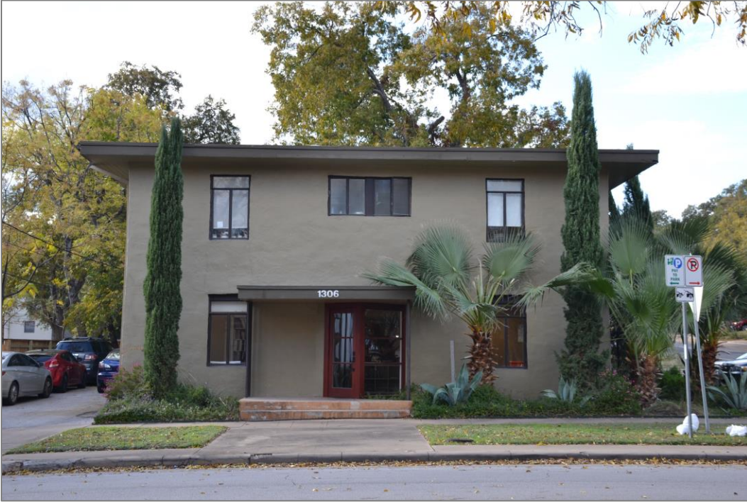
Photo 34. Photograph of an apartment complex constructed around 1945 at 1306 Rio Grande, facing east, 2019. Photo by HHM.
