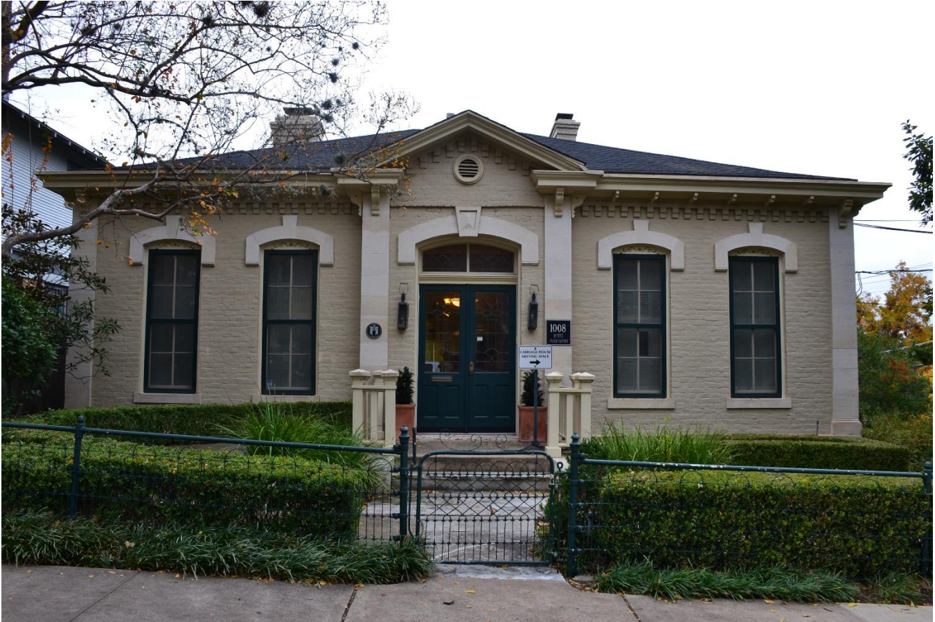
Photo 5. Photograph of 1008 West Avenue, facing west, 2019. Photo by HHM.
