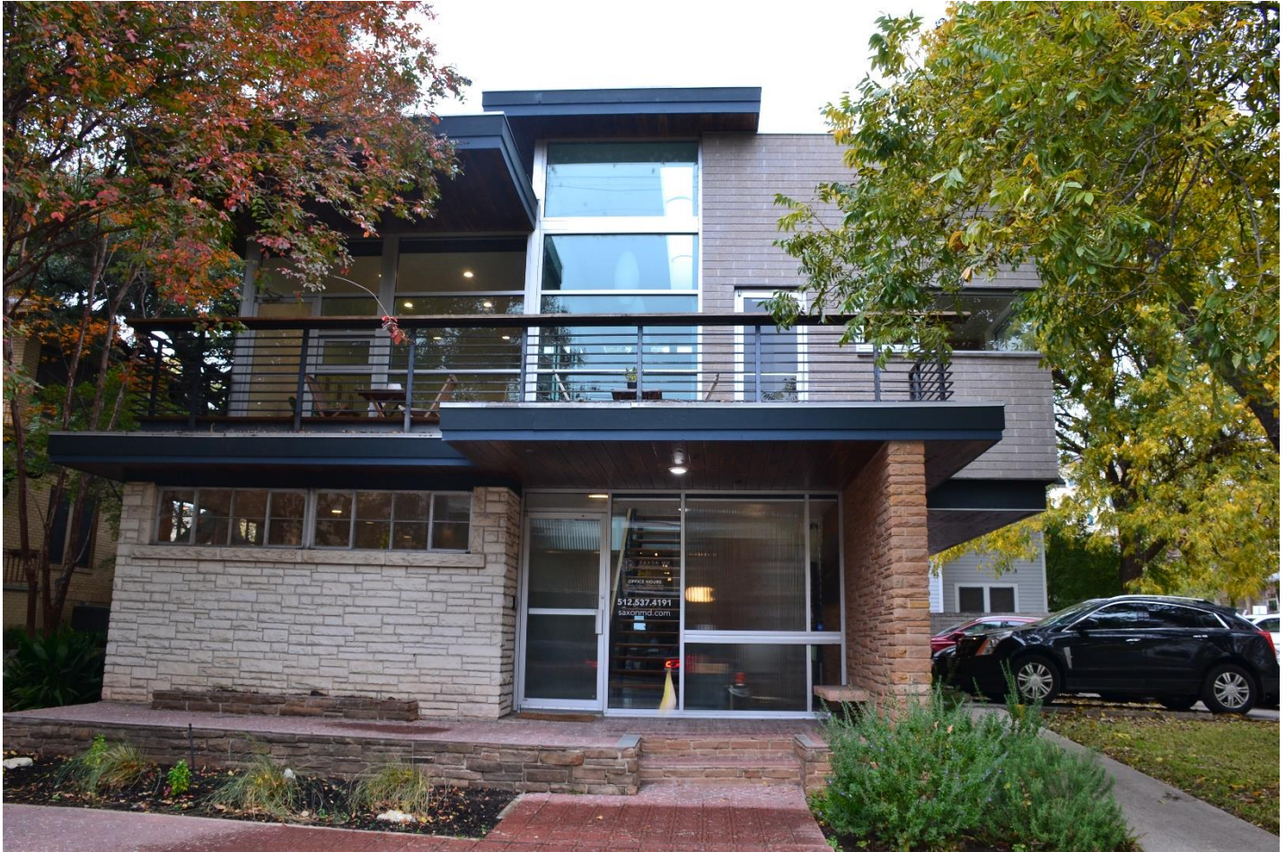
Photo 51. Photograph of 1100 Nueces Street, a noncontributing resource, facing north, 2019. Photo by HHM.
