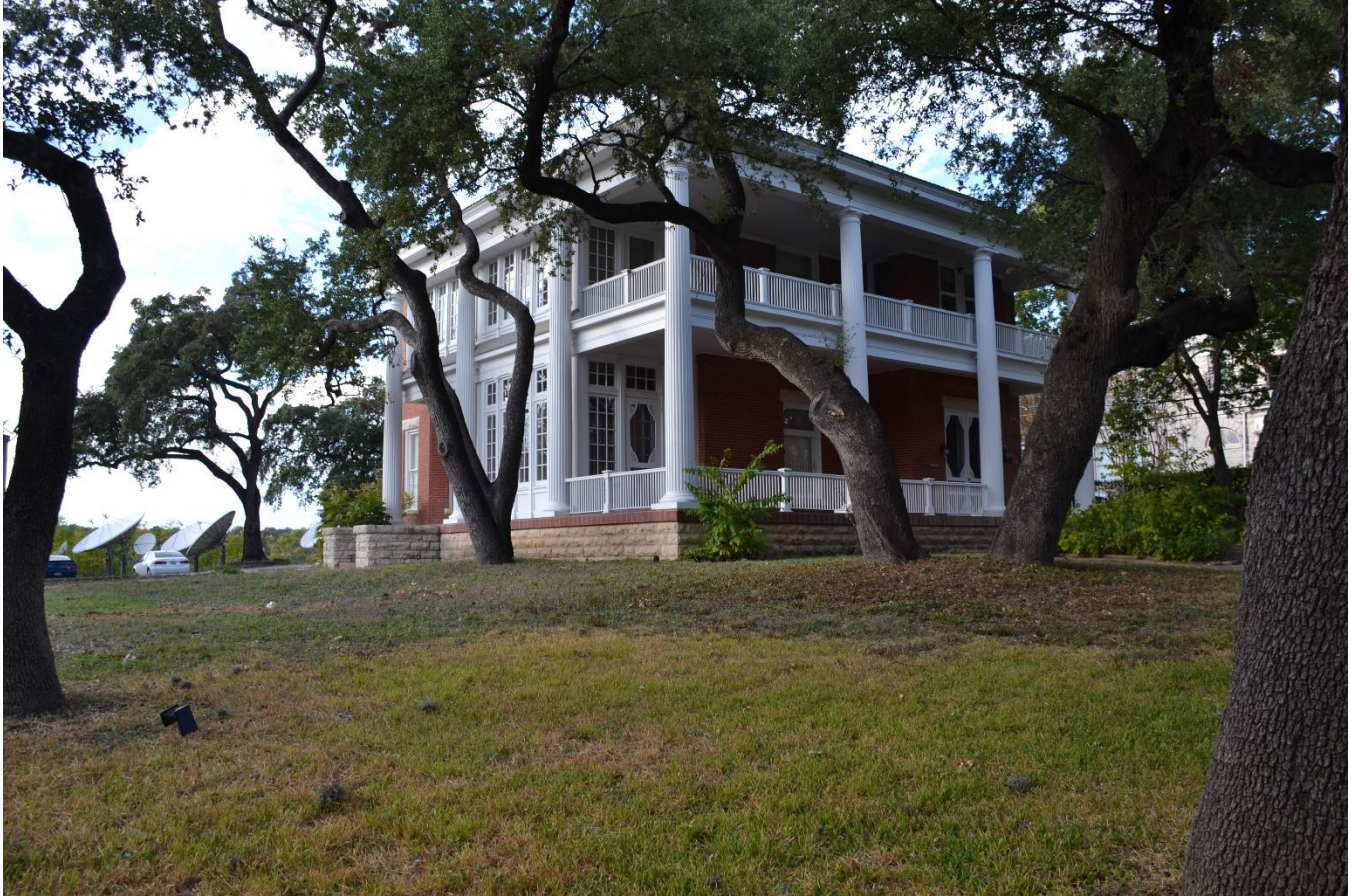
Photo 1. Photo of 1402 West Avenue, facing northwest, 2019. Photo by HHM.
