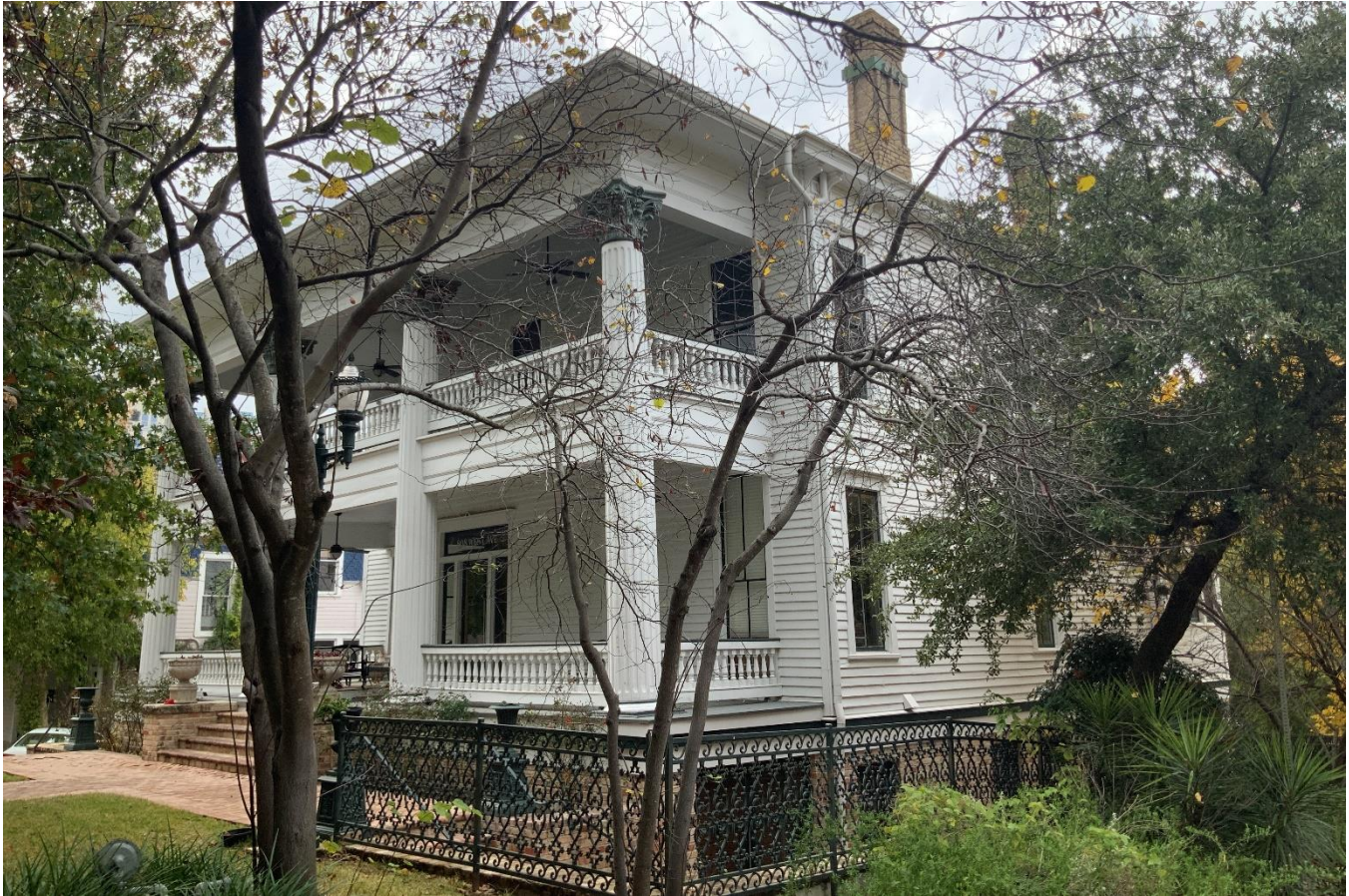
Photo 6. Photograph of 808 West Avenue, facing southwest, 2019. Photo by HHM.
