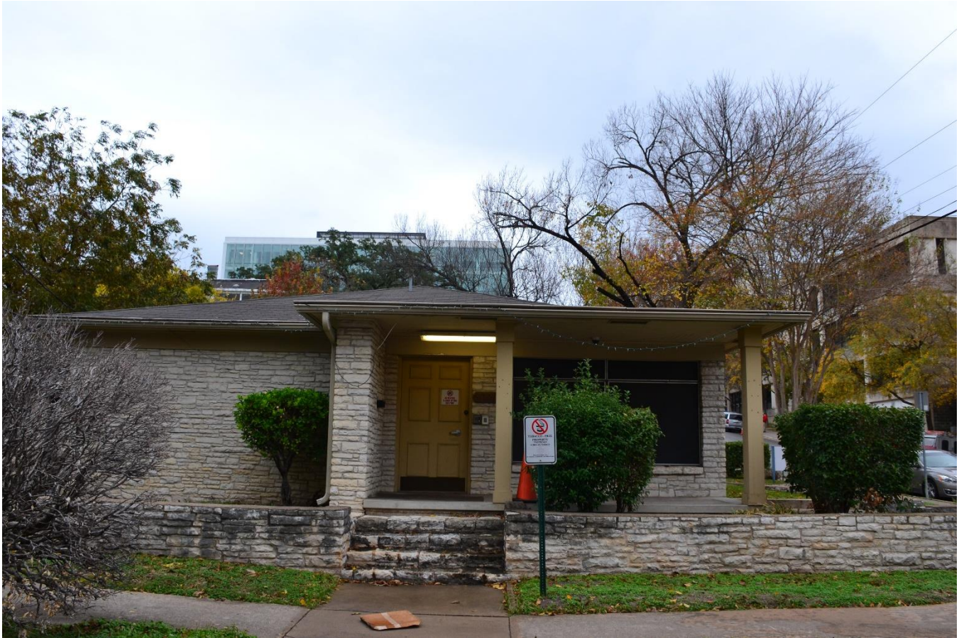
Photo 42. Photograph of 1101 Nueces Street, facing east, 2019. Photo by HHM.
