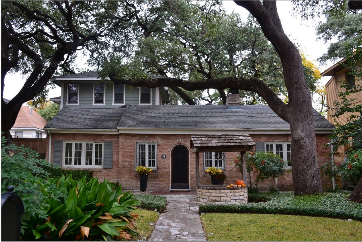
Photo 13. 604 W. 11 th Street, facing north, 2019. Note the original building's small scale and lack of architectural ornament. The building addition evident in the left portion of the photograph was added in 1930, along with plumbing and electricity. The upper story was added in 2004. Both are alterations made to the original residence. Photo by HHM.
