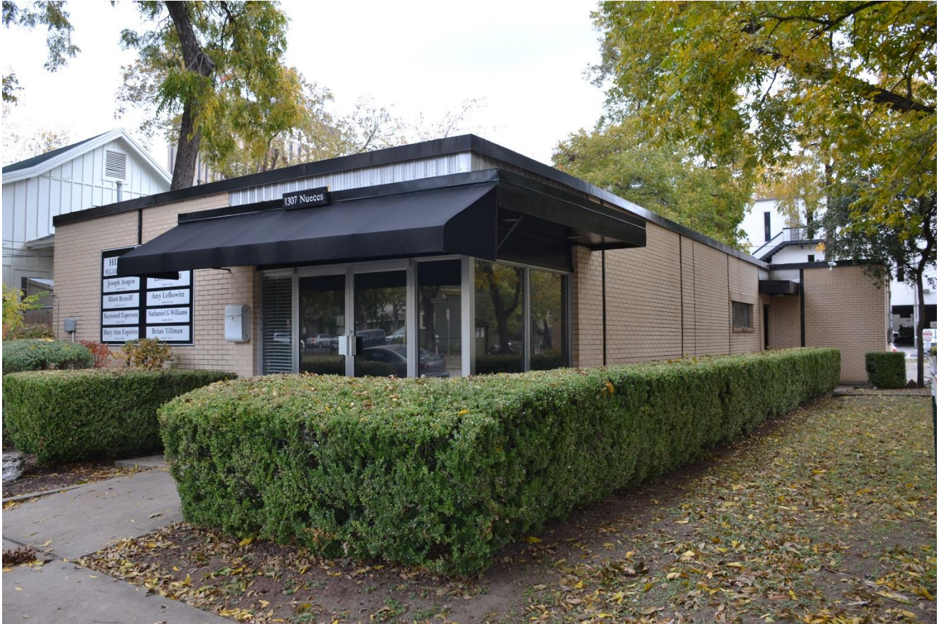
Photo 43. Photograph of 1307 Nueces Street, facing east, 2019. Photo by HHM.
