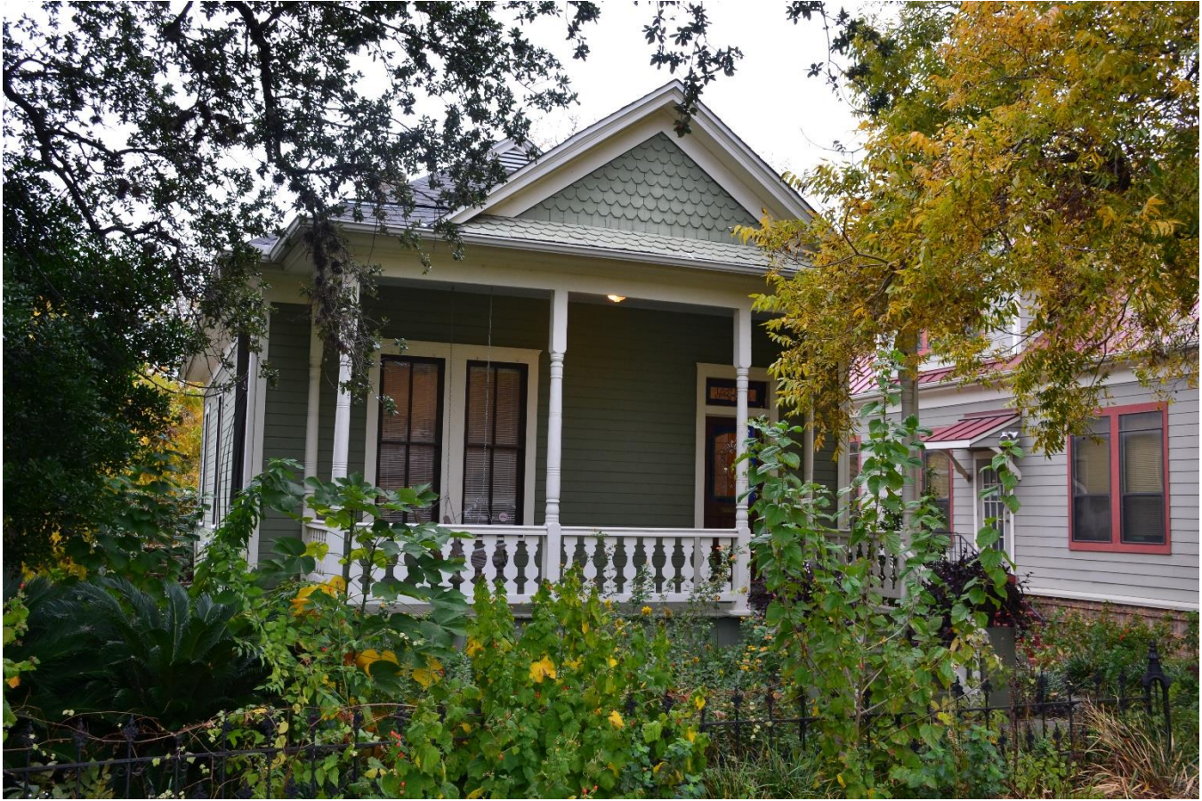
Photo 38. 1102 West Avenue, facing west, 2019. Photo by HHM.
