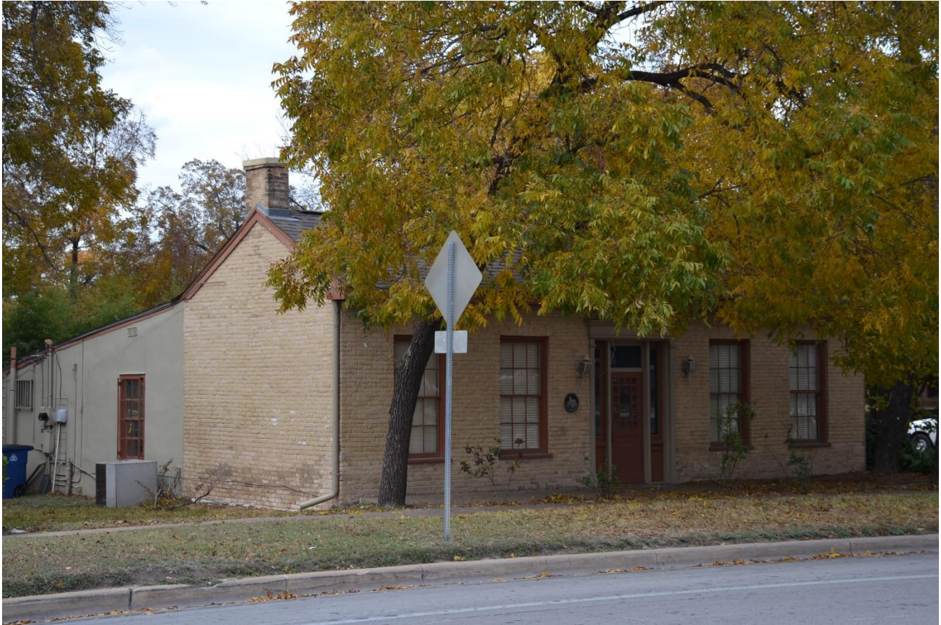
Photo 14. Photograph of 1306 Guadalupe Street, facing northwest, 2019. Photo by HHM.
