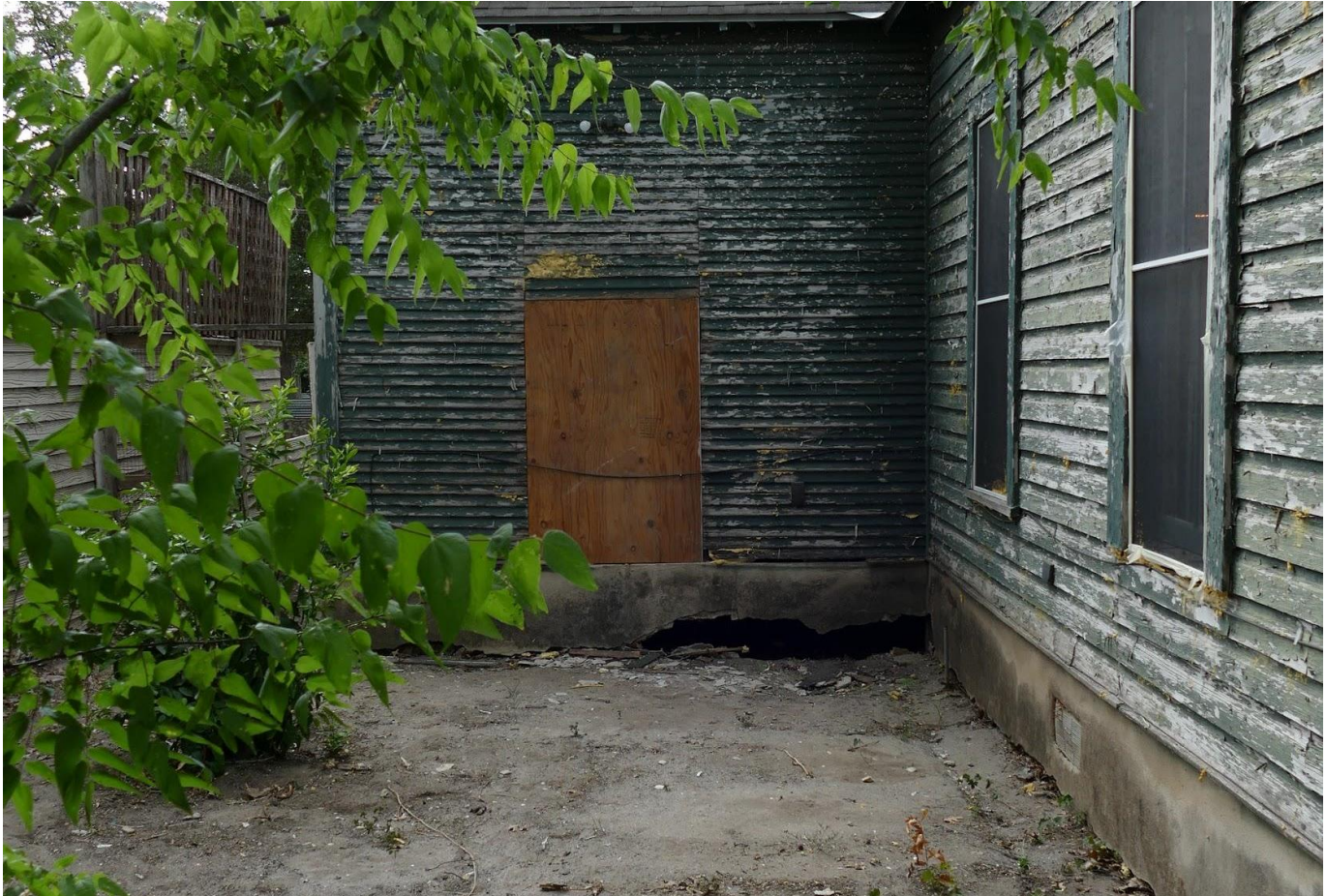
Photo 11: East wing North Elevation. View South.
