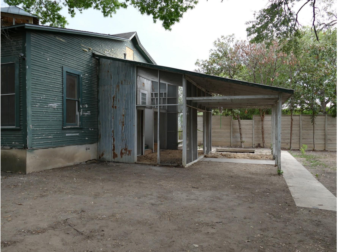
Photo 6: South Elevation, View East.
