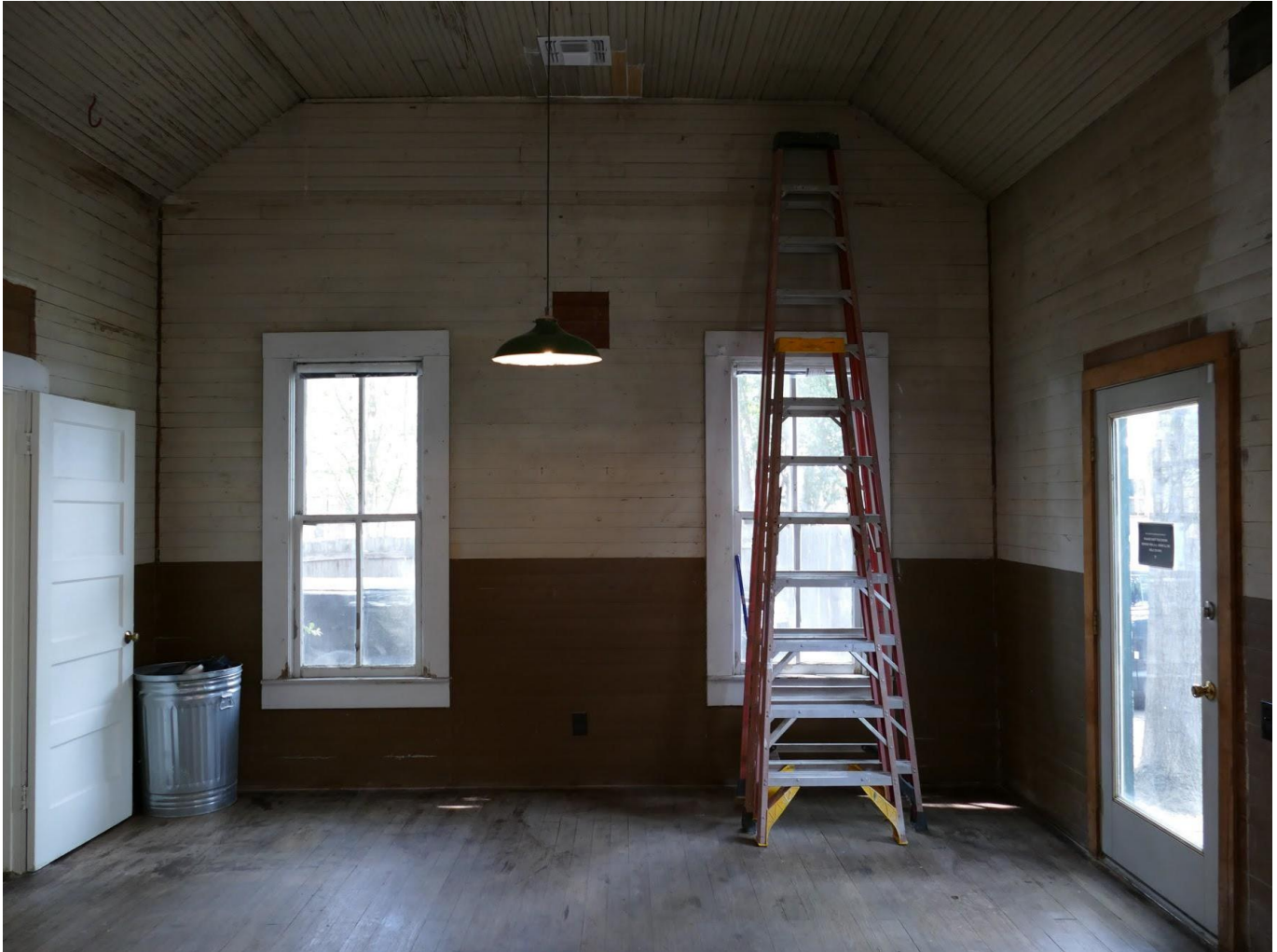
Photo 15: West wing/transsept. View West.
