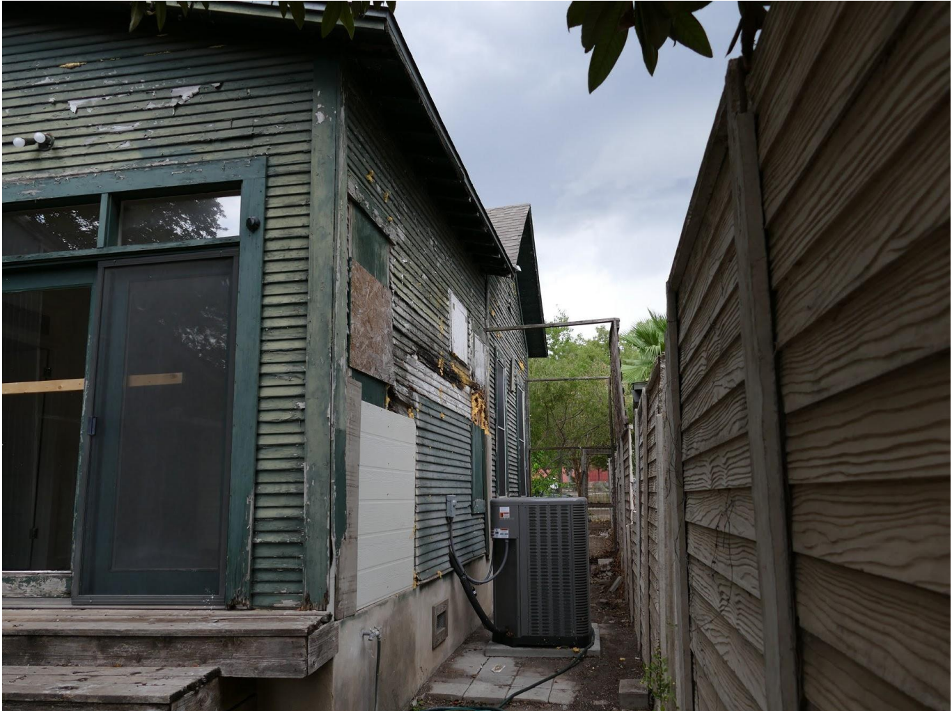
Photo 10: South and East Elevations. View North.
