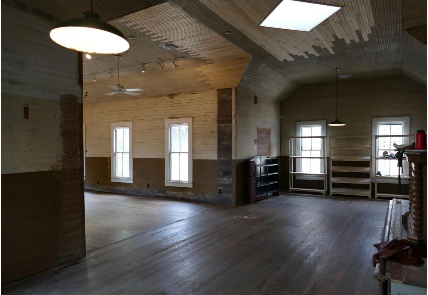
Photo 16: View from transept into nave. View Northeast.
