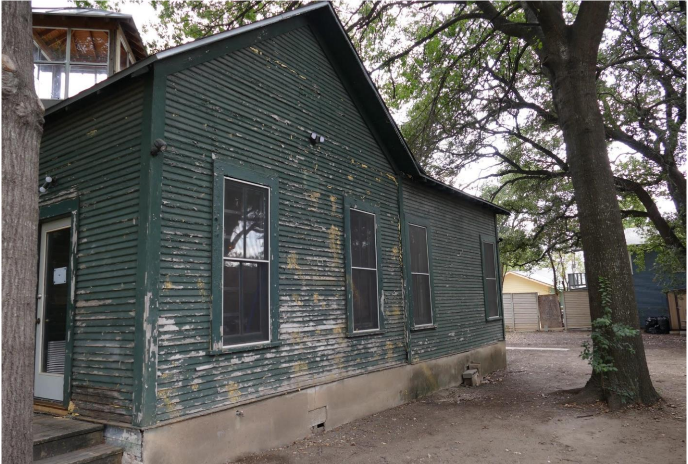
Photo 5: West Elevation. View Southeast.
