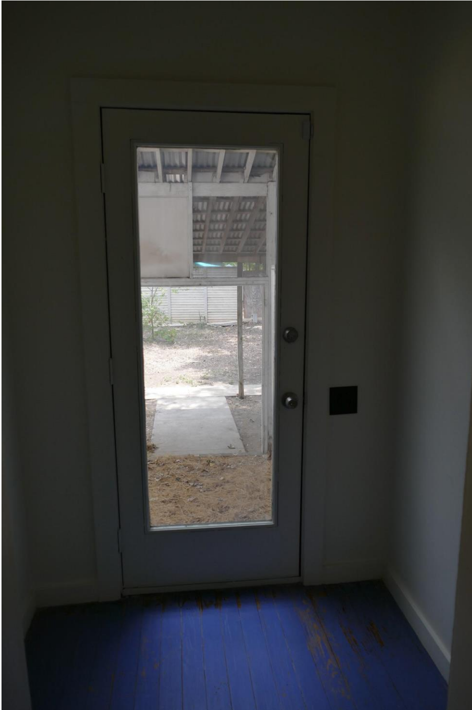
Photo 25: Rear hall with exterior door. View South.
