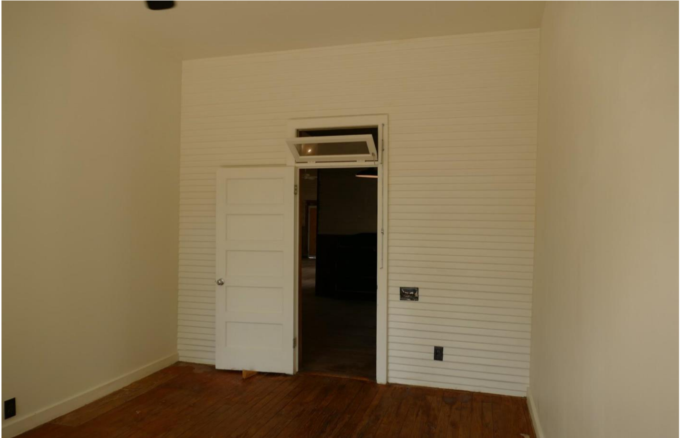
Photo 23: East room in rear addition. View North.
