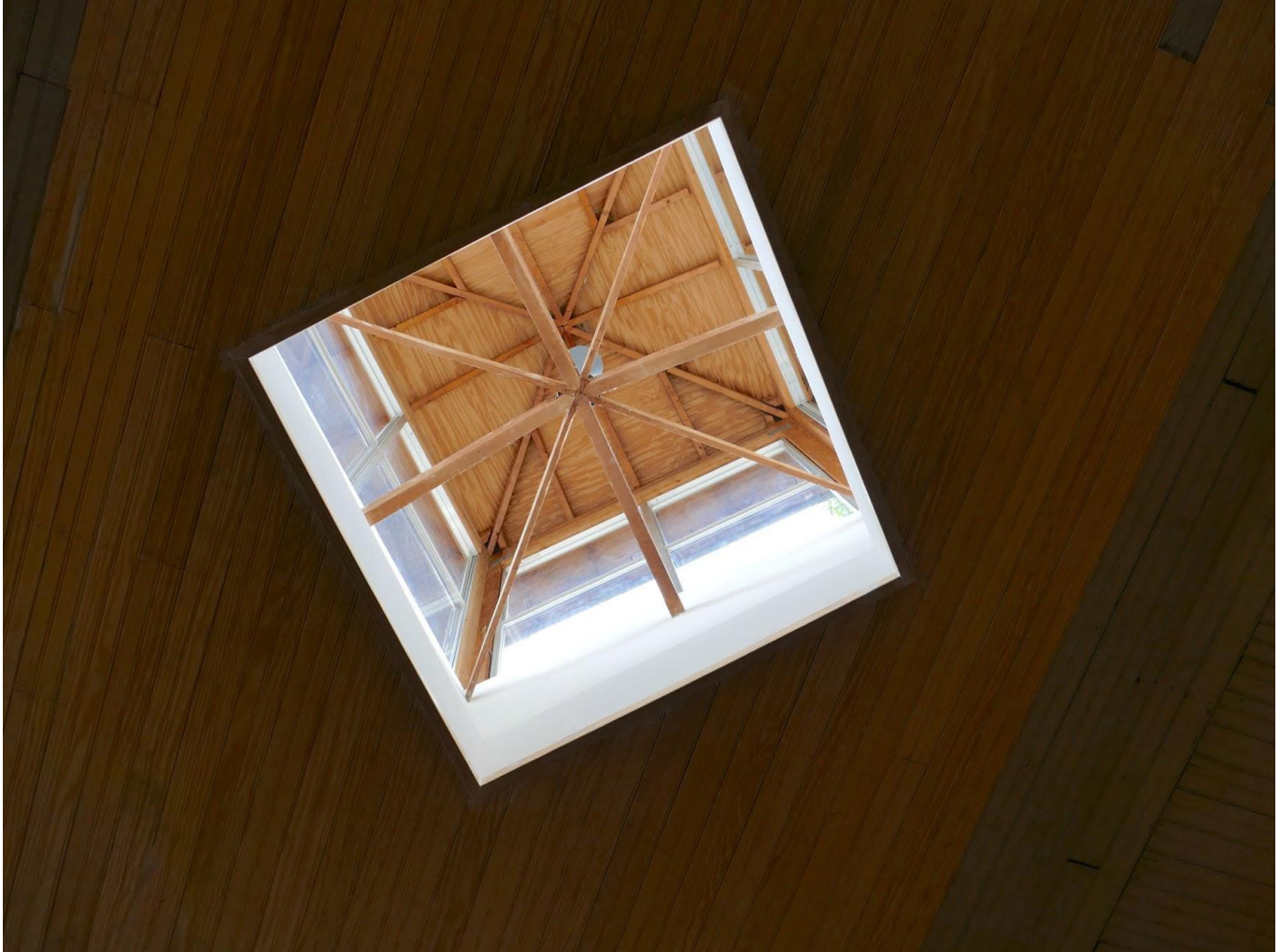
Photo 18: View of cupola above transept.
