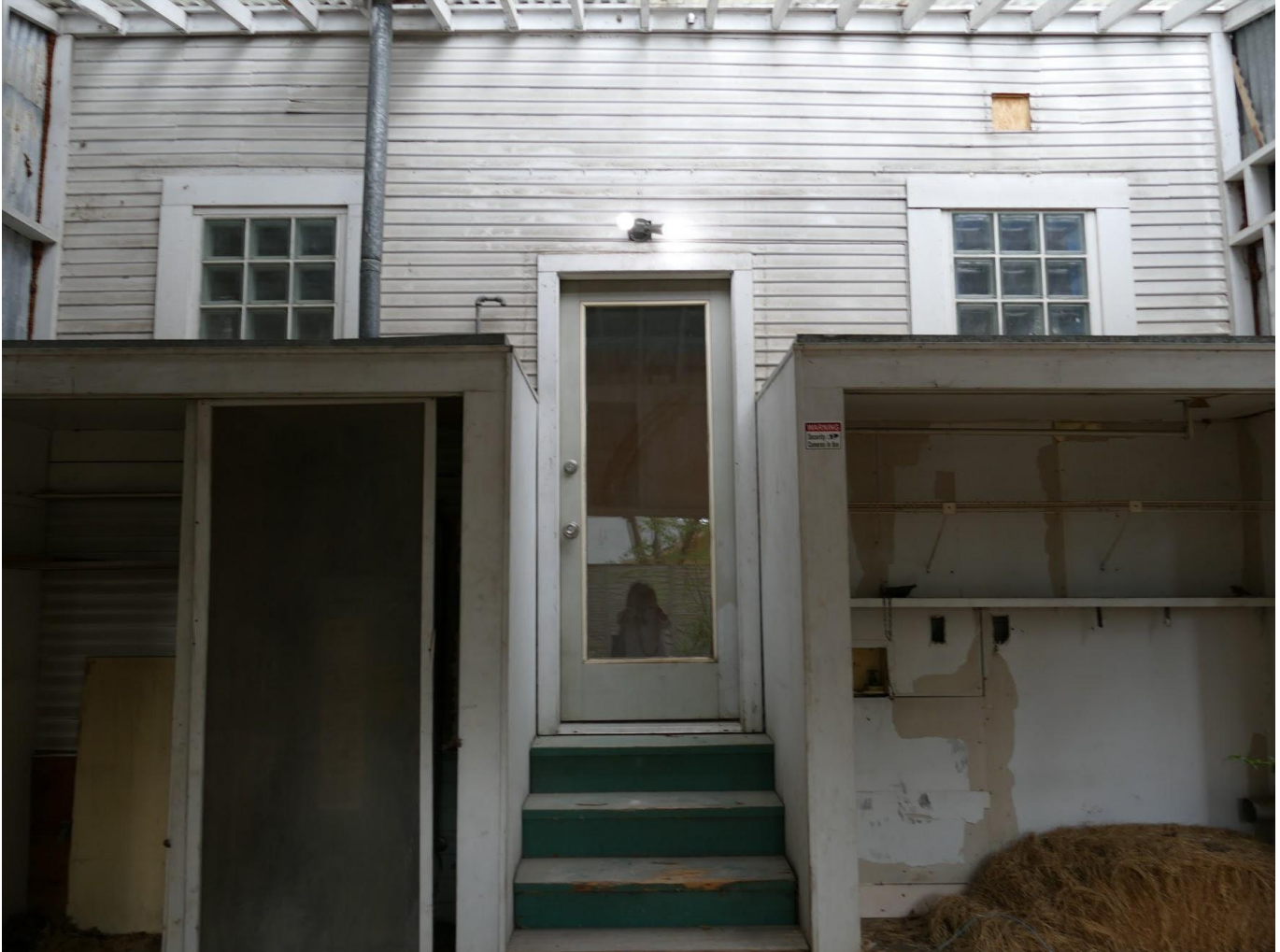
Photo 8: South Elevation beneath Shed. View North.
