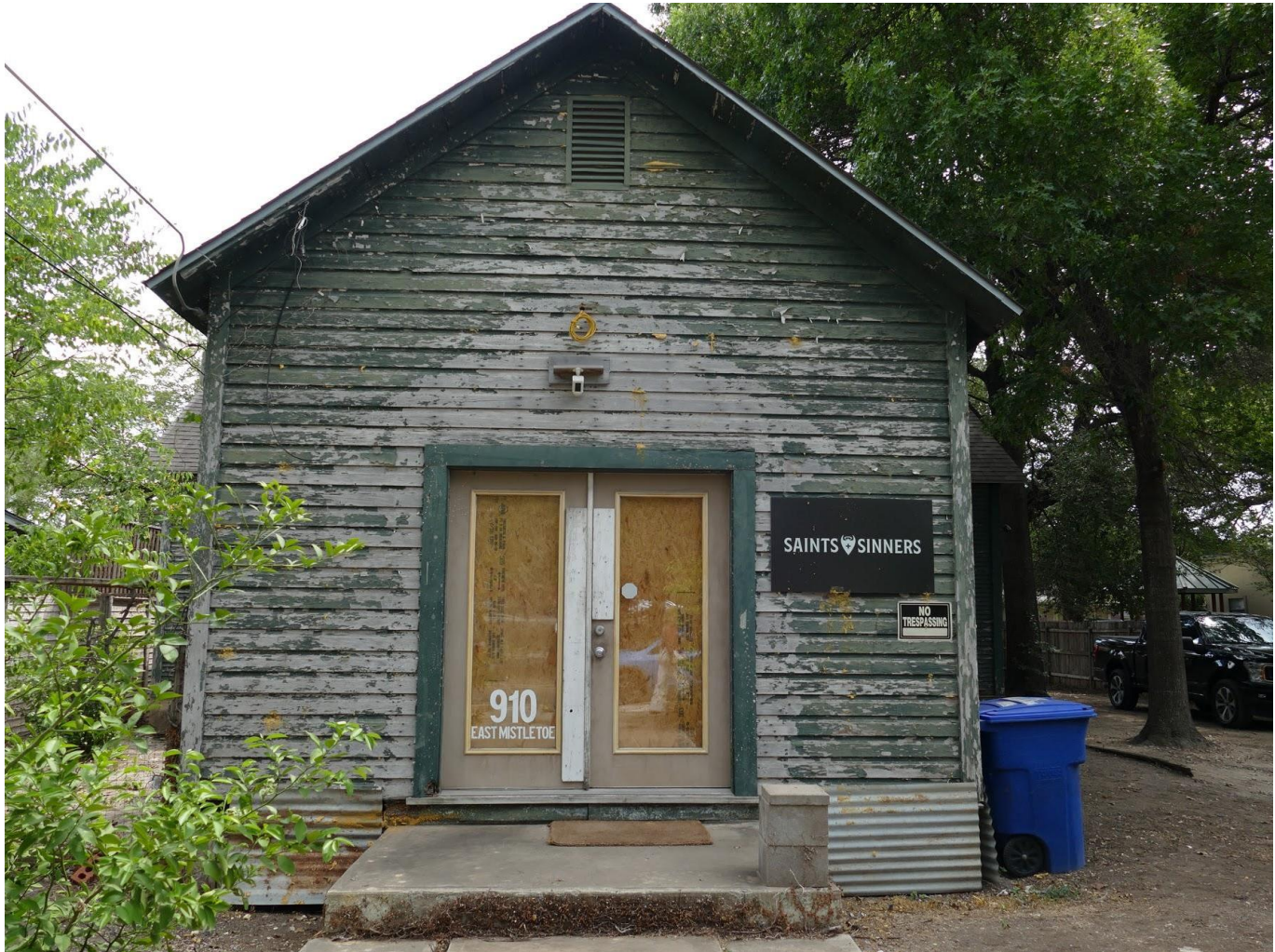
Photo 3: Primary (North) Elevation. View South.
