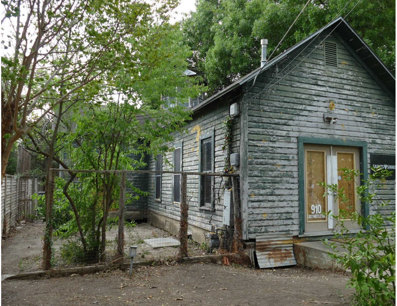
Photo 12: North and East Elevations. View Southwest.
