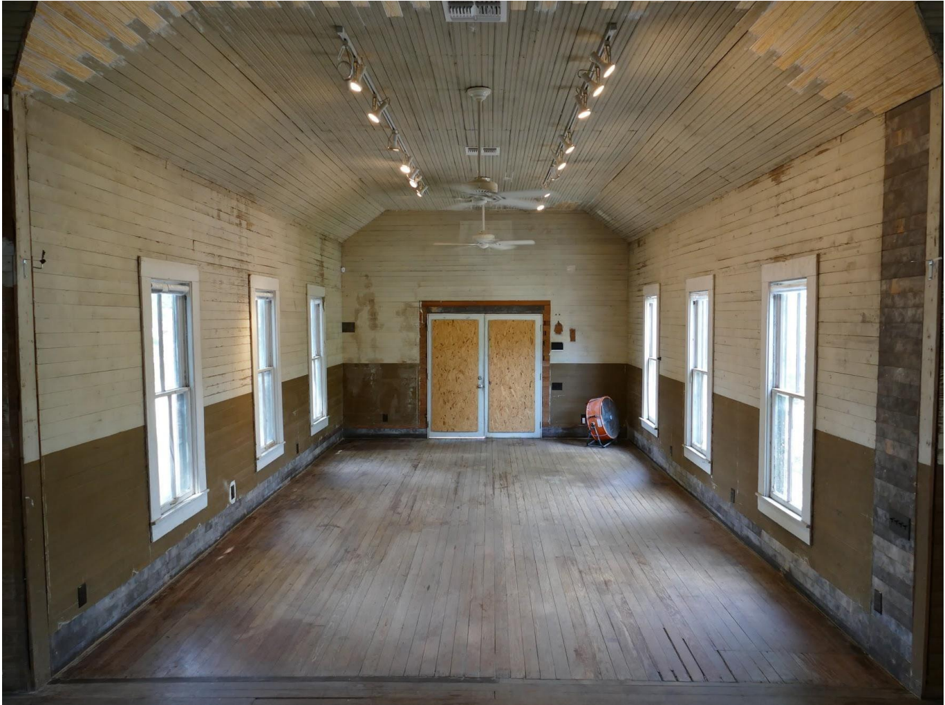
Photo 13: Nave facing main entrance. View North.
