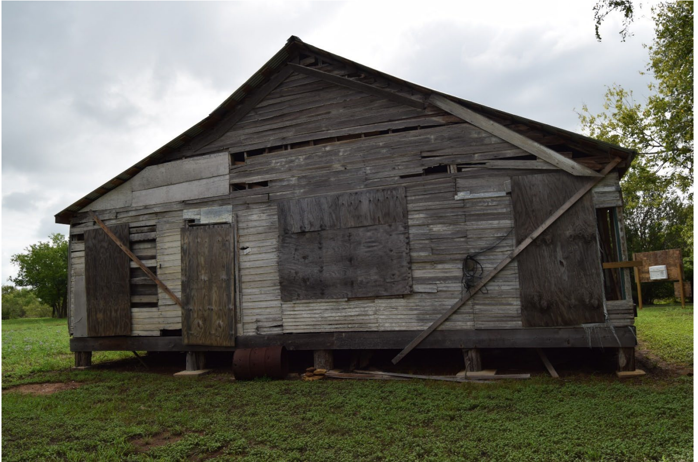
Photograph 9. West façade. Camera facing east.
