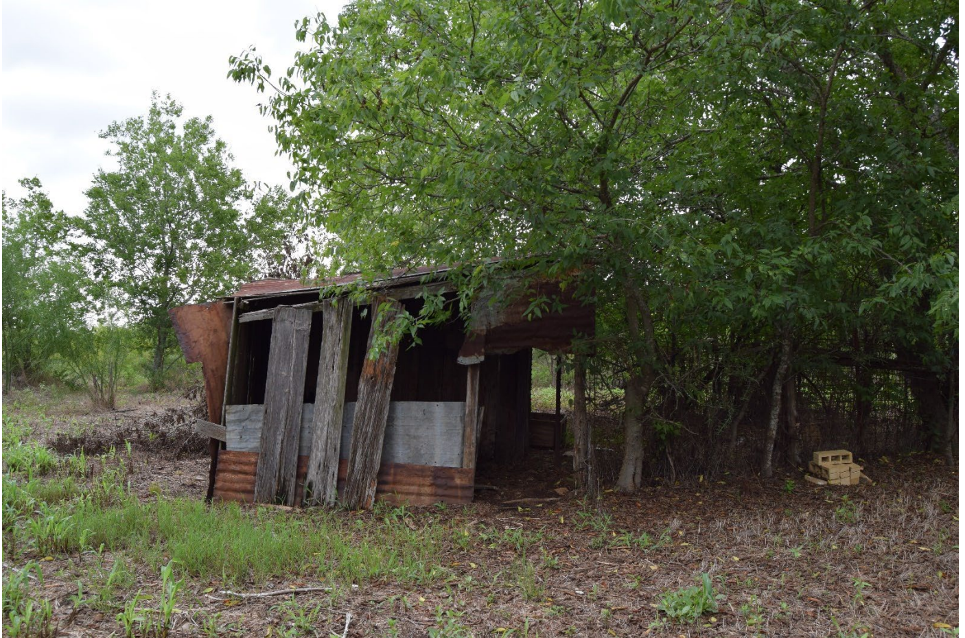
Photograph 24. Barn at north end of property. Camera facing east.
