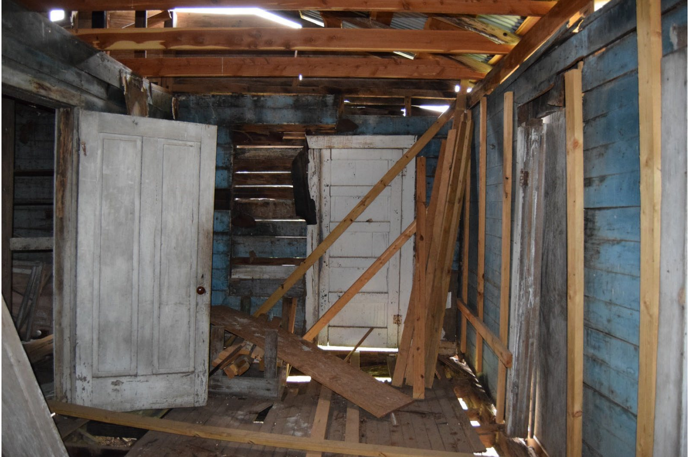
Photograph 19. Kitchen/Dining Room interior. Camera facing west.
