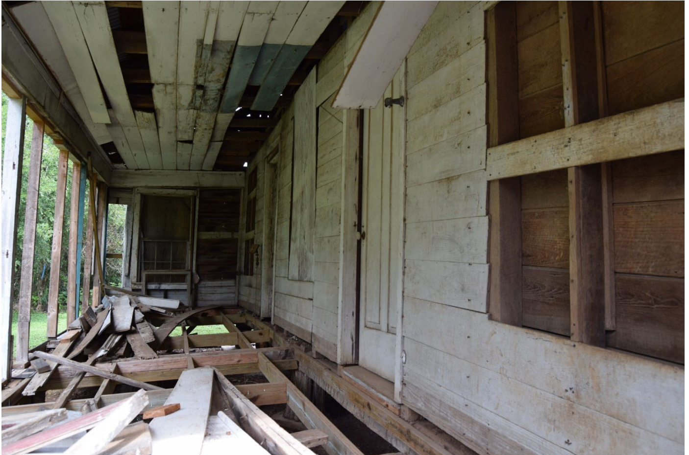
Photograph 4. Porch at south façade. Camera facing west.
