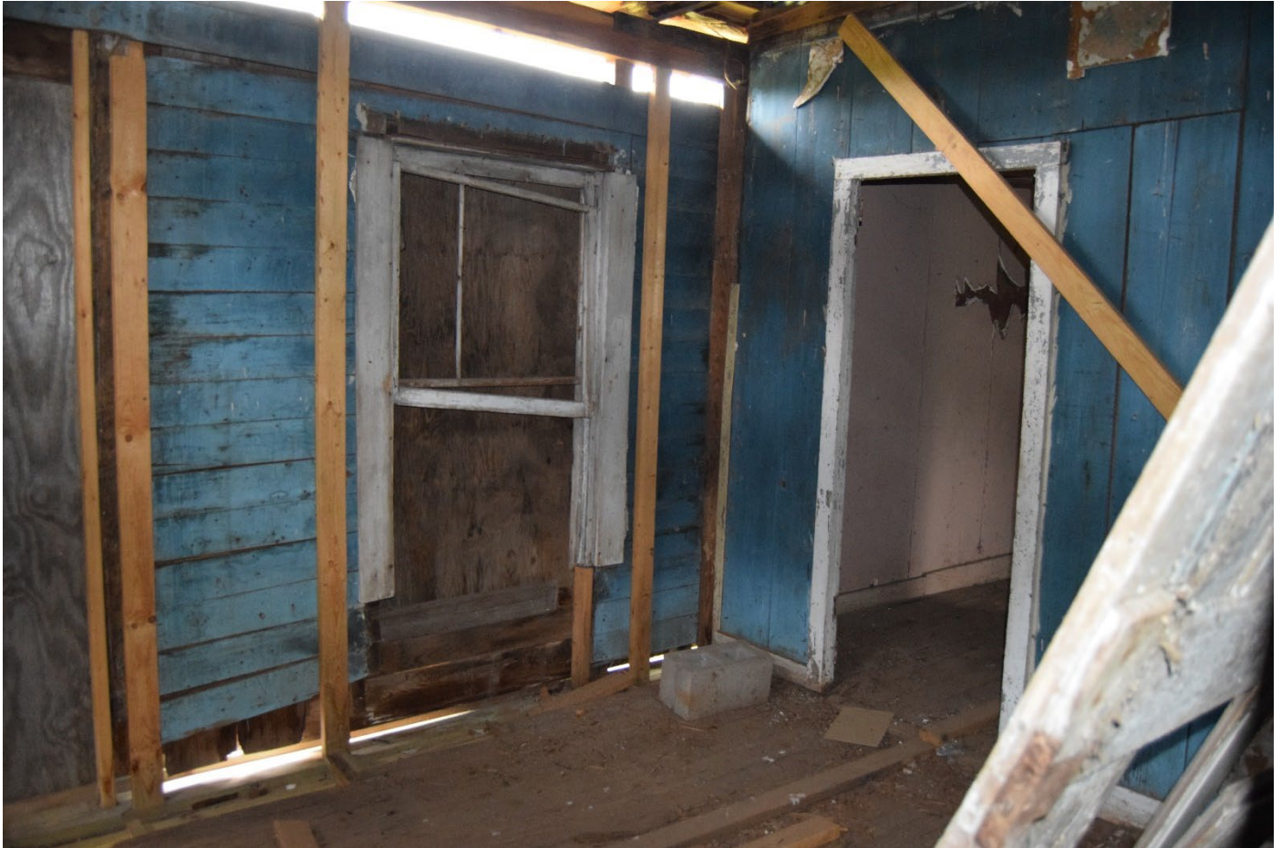
Photograph 20. Kitchen/Dining Room interior. Camera facing northeast towards Back Bedroom.
