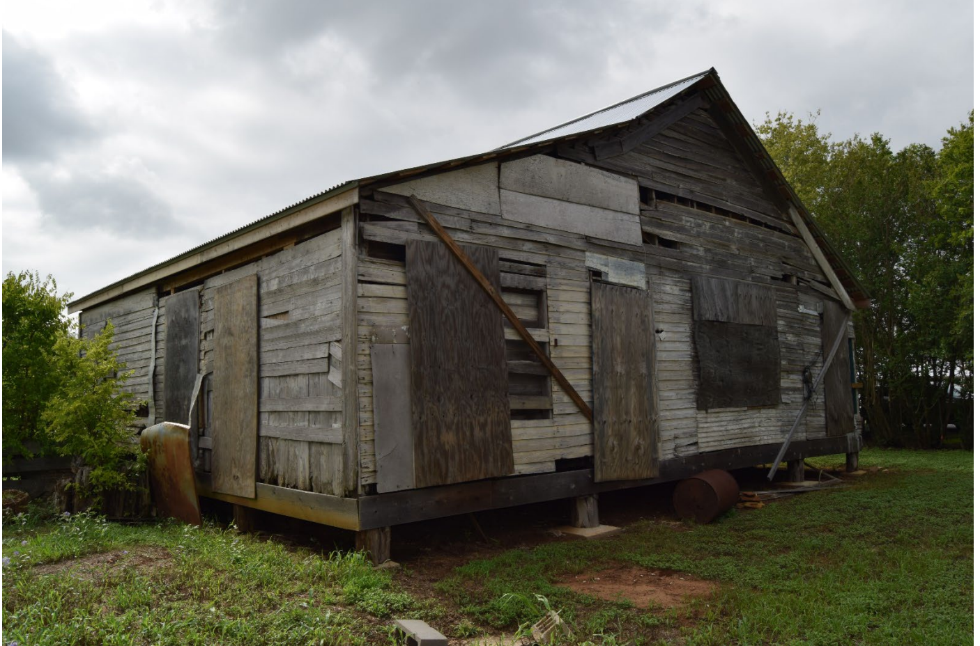
Photograph 8. North and west façades. Camera facing southwest.
