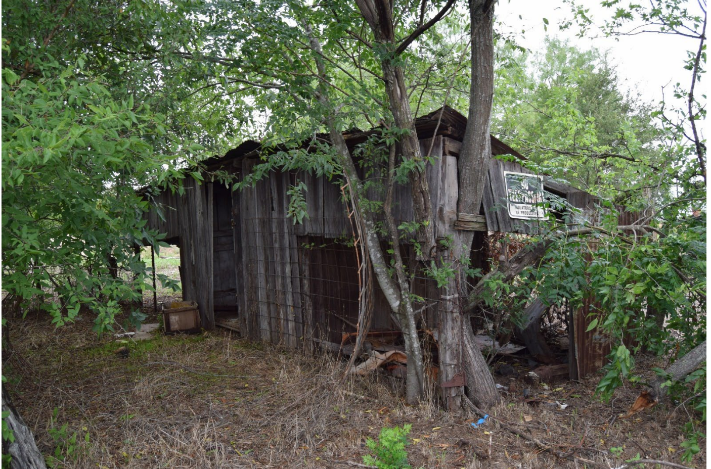
Photograph 23. Barn at north end of property. Camera facing northwest.
