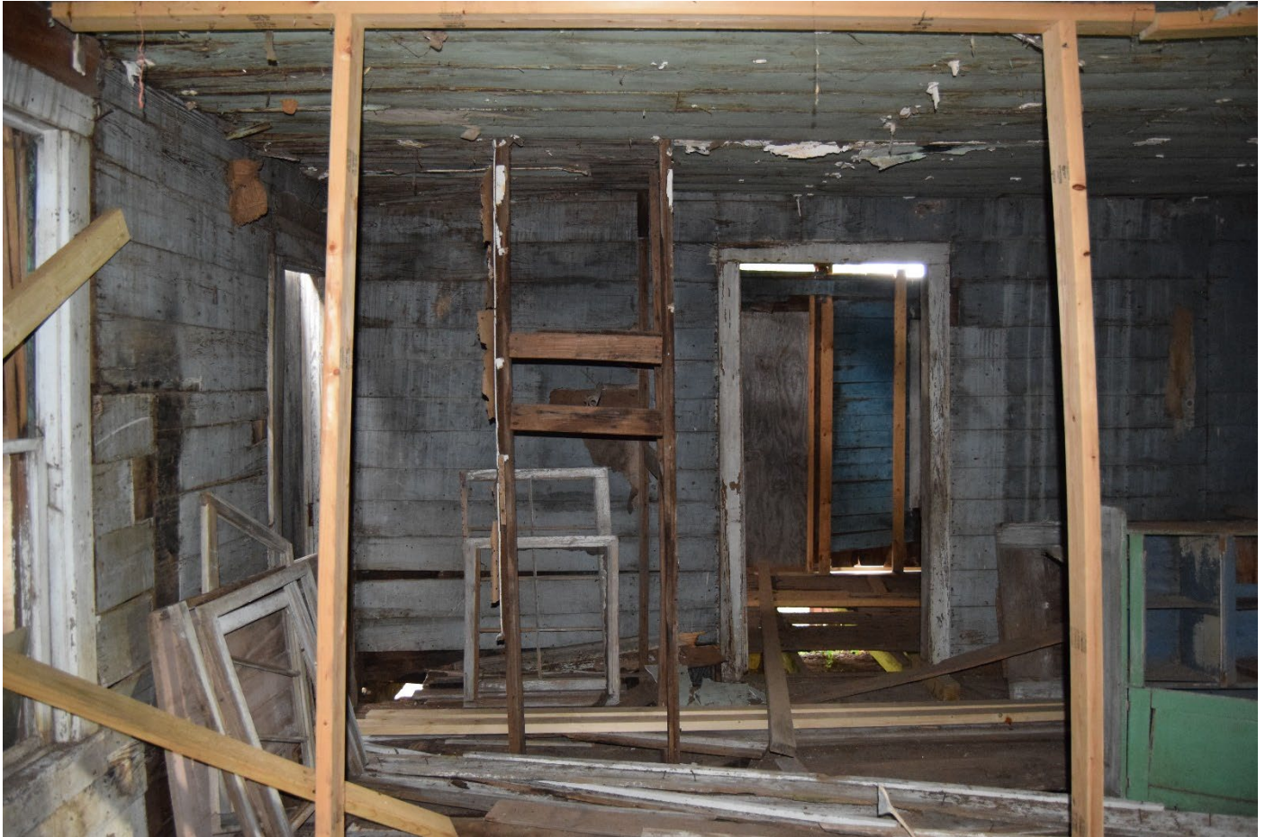
Photograph 12. Main Bedroom interior. Camera facing north towards Kitchen/Dining Room.
