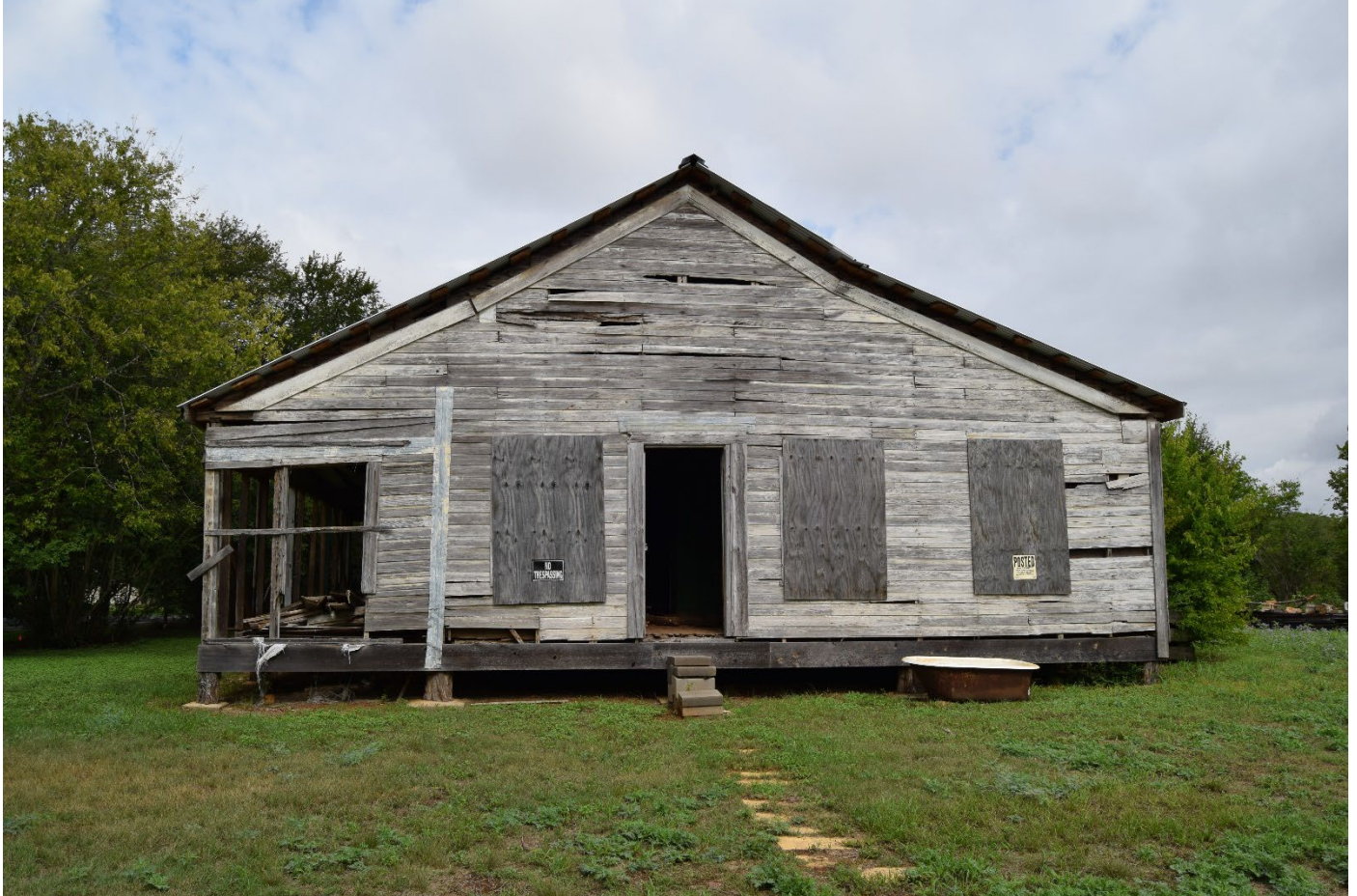
Photograph 5. East façade. Camera facing west.
