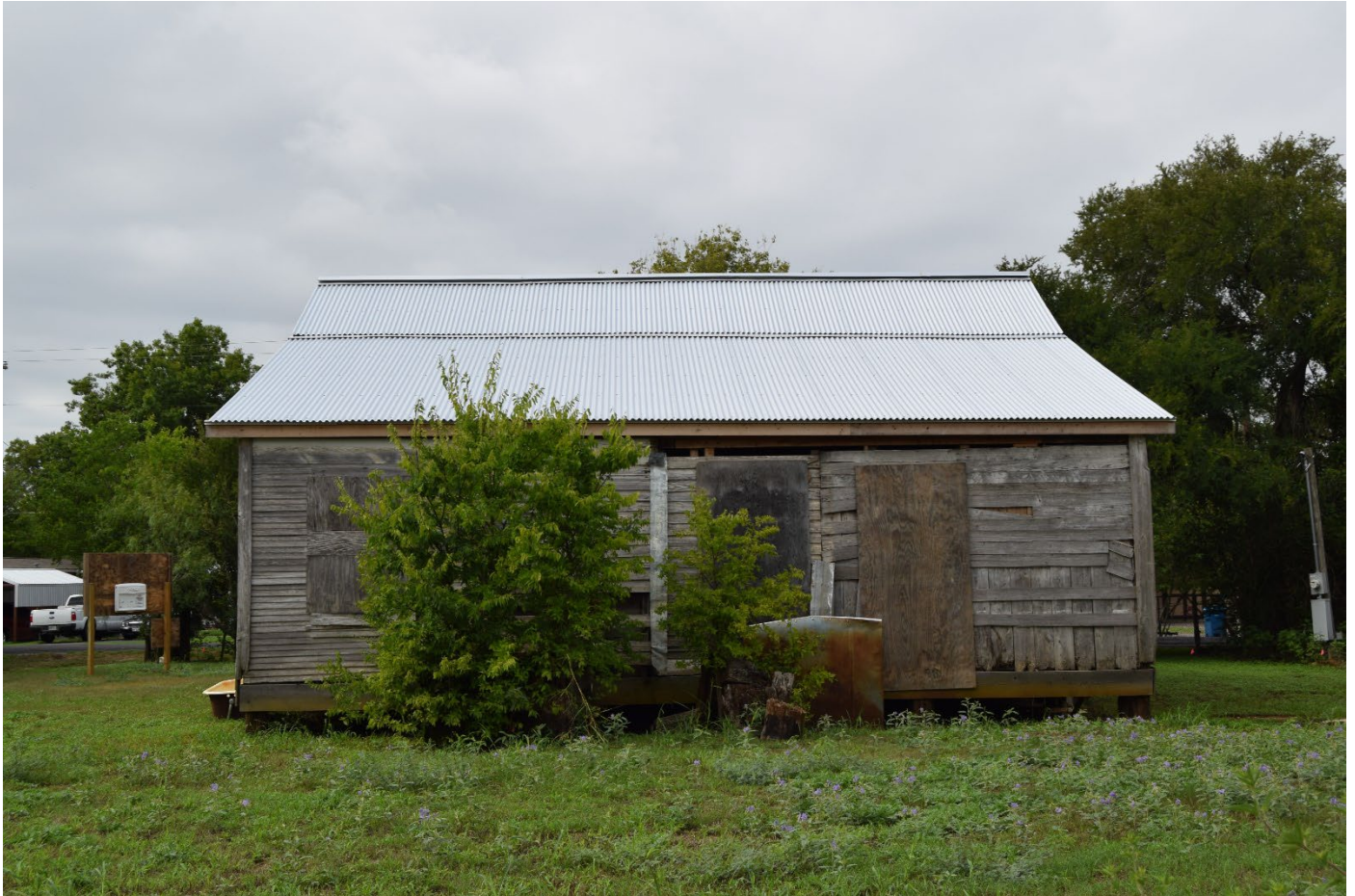
Photograph 7. North façade. Camera facing south.
