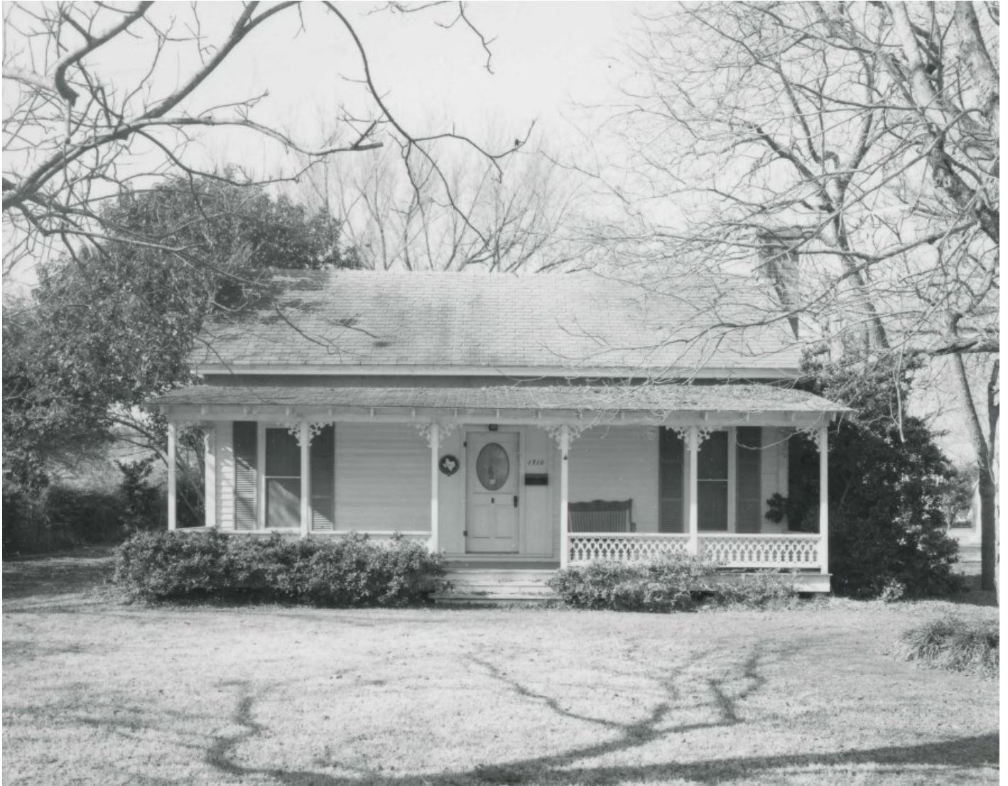
Figure 15. The ca. 1830 Jenkins House at 1710 Main Street in Bastrop, Texas. 196
