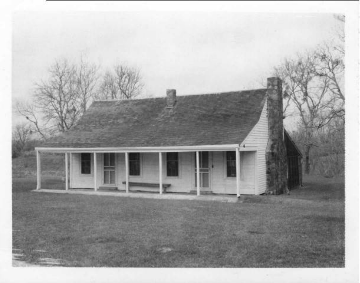
Figure 14. The ca. 1836 Thomas Barnett House in Rosenberg, Fort Bend County, Texas, is an example of house with a dual-pitched roof and two rooms without an open breezeway, like the Burleson House. 195
