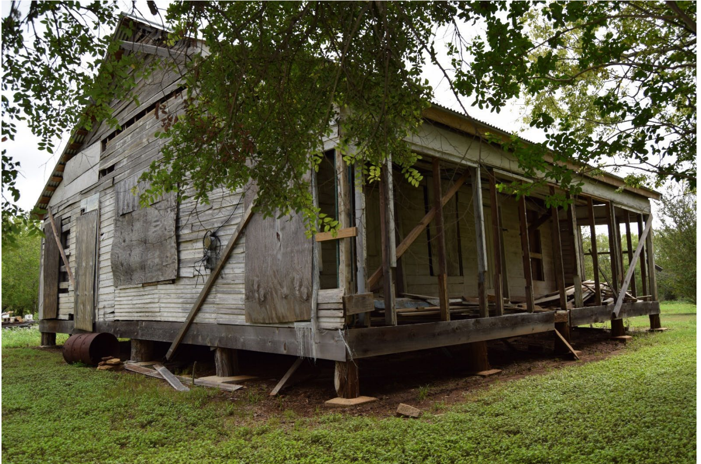
Photograph 2. West and south façades. Camera facing northeast.
