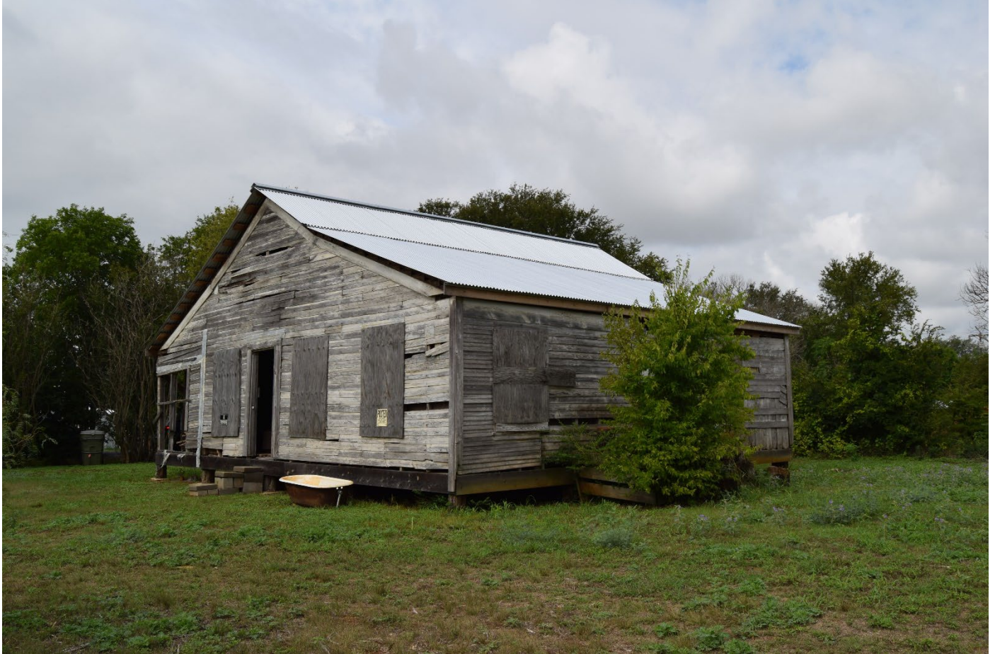
Photograph 6. North and east façades. Camera facing southwest.
