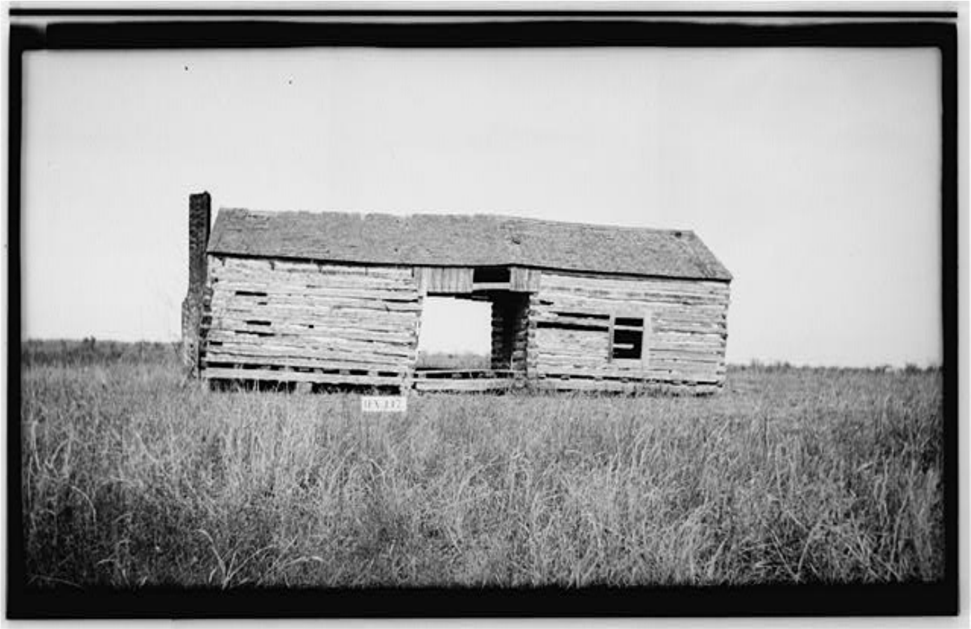
Figure 13. The early 1840s Tom Ireland House in Webberville, Texas, an example of a double-crib cabin or dog-trot house with a breezeway separating two rooms, a common early Texas house form. 194
