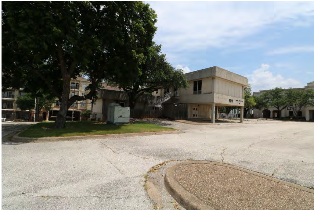
Photo 28: 1969 Outpatient Services Building, North and West Elevations, looking southeast.
