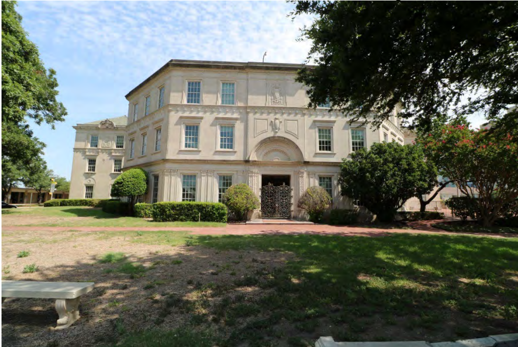
Photo 1: 1929-1958 Section, South Elevation, looking north.
