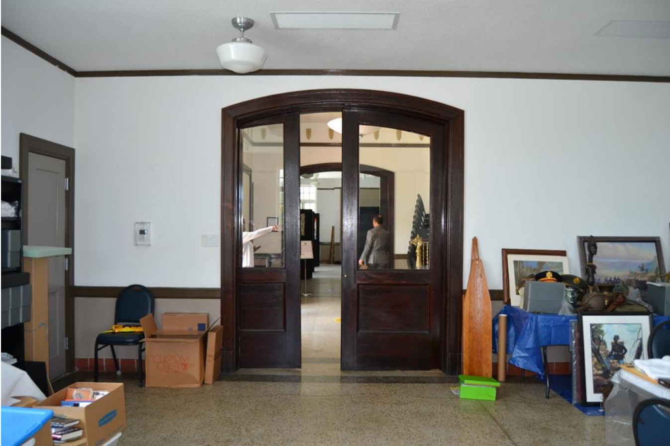
Photo 17. Original sliding pocket door in former club room opening to front wing historic-period entrance lobby. Camera facing southwest.
