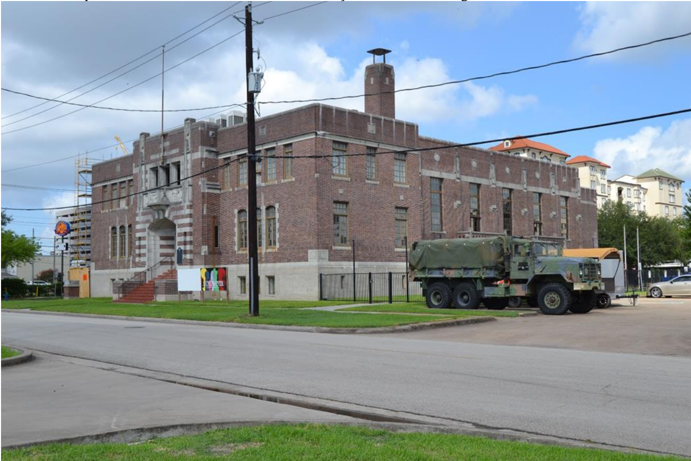
Photo 2. Oblique of front southeast and side northeast façades. Camera facing south.
