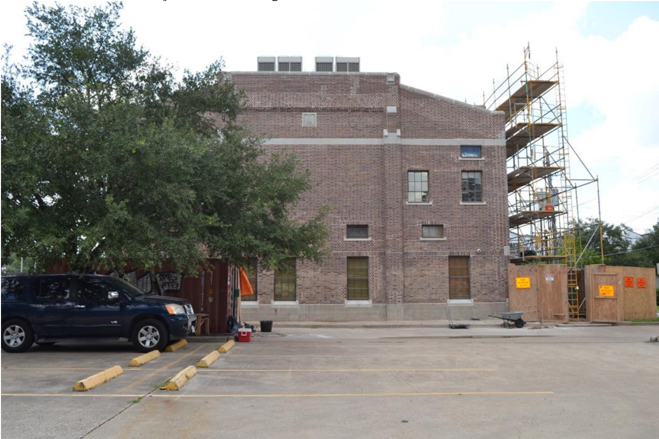
Photo 12. Rear northwest façade. Camera facing southeast.
