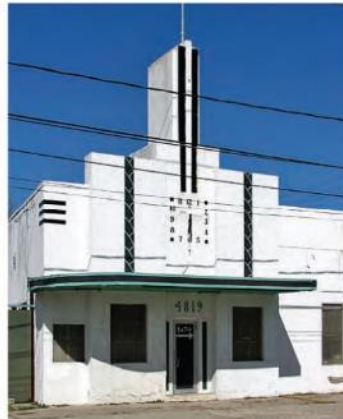
15. 4819 Harrisburg Blvd, Formerly Sterling Laundry & Cleaning Co. 1935. Photo by David Bush.
