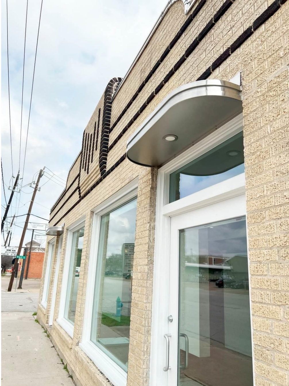
Photo 3: Primary (west) elevation showing metal awnings and display windows and entrances. February 17, 2023.
