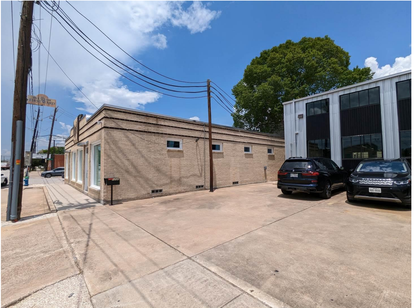
Photo 7: South elevation with adjacent building at 1224 Houston Avenue at right. June 8, 2023.
