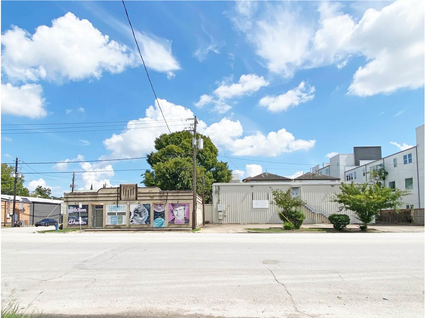
Figure 18: Knapp Building C. 2021 Prior to Rehabilitation.
