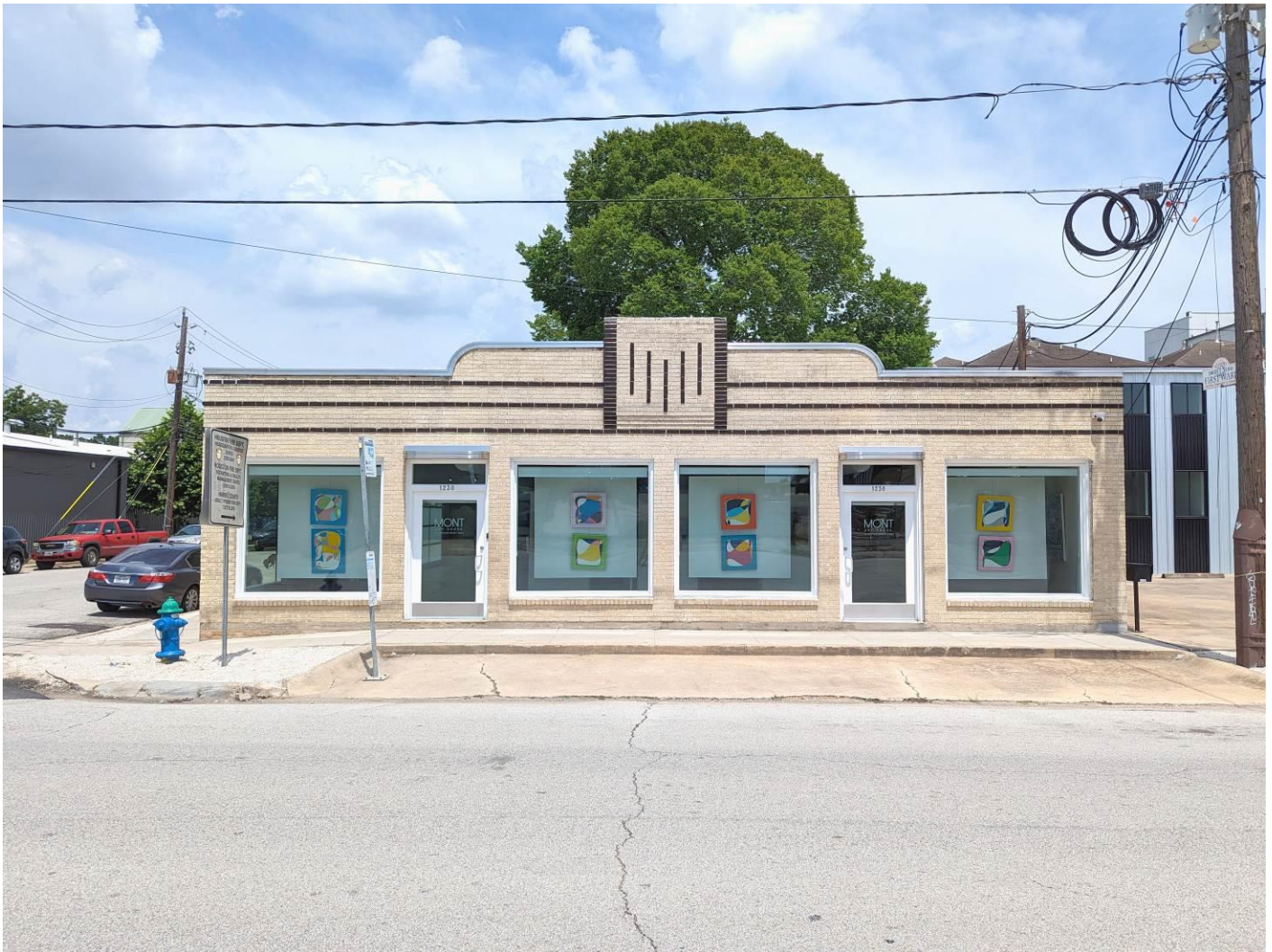
Photo 1: Primary (west) elevation facing Houston Avenue. June 8, 2023.
