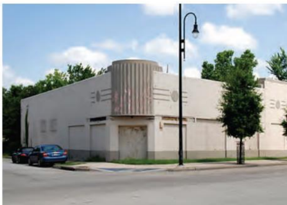
8. 5210-5216 Alameda Rd, Formerly Minimax Grocery Store No.2 1938. Photo by Jim Parsons.
