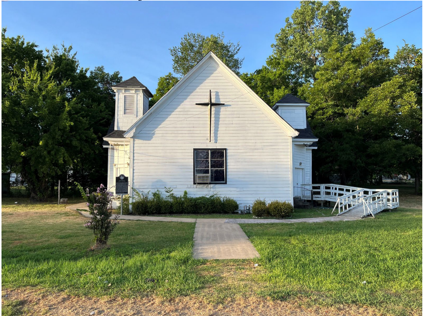
Photo 3: North elevation, camera facing south.
