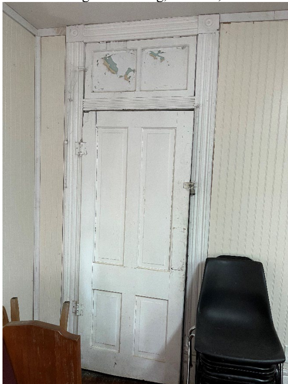
Photo 16: Original molding, transom, and door inside the dining room. Camera looks east.
