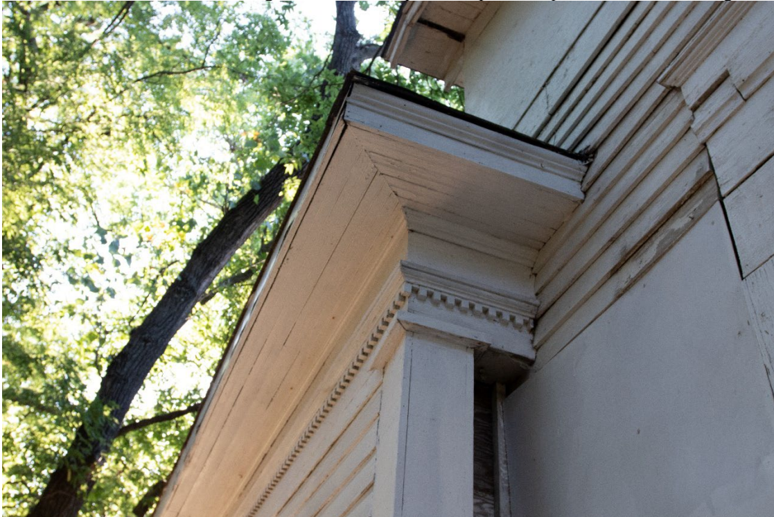
Photo 9: Dentilled wood molding and modest “capitals” top corner posts. Camera looking at south elevation.
