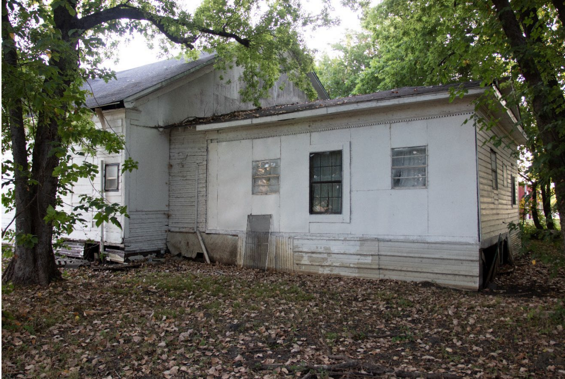
Photo 8: West elevation showing rear addition. Camera looks northeast.
