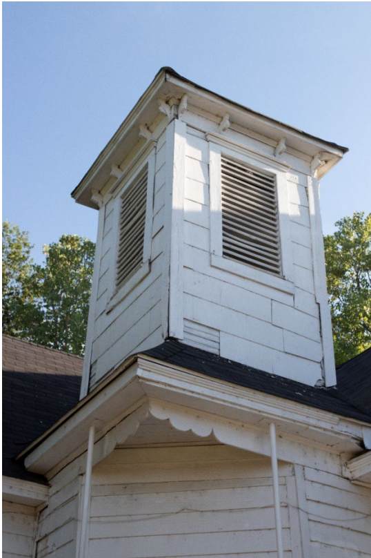
Photo 5: Detail of northeast tower.
