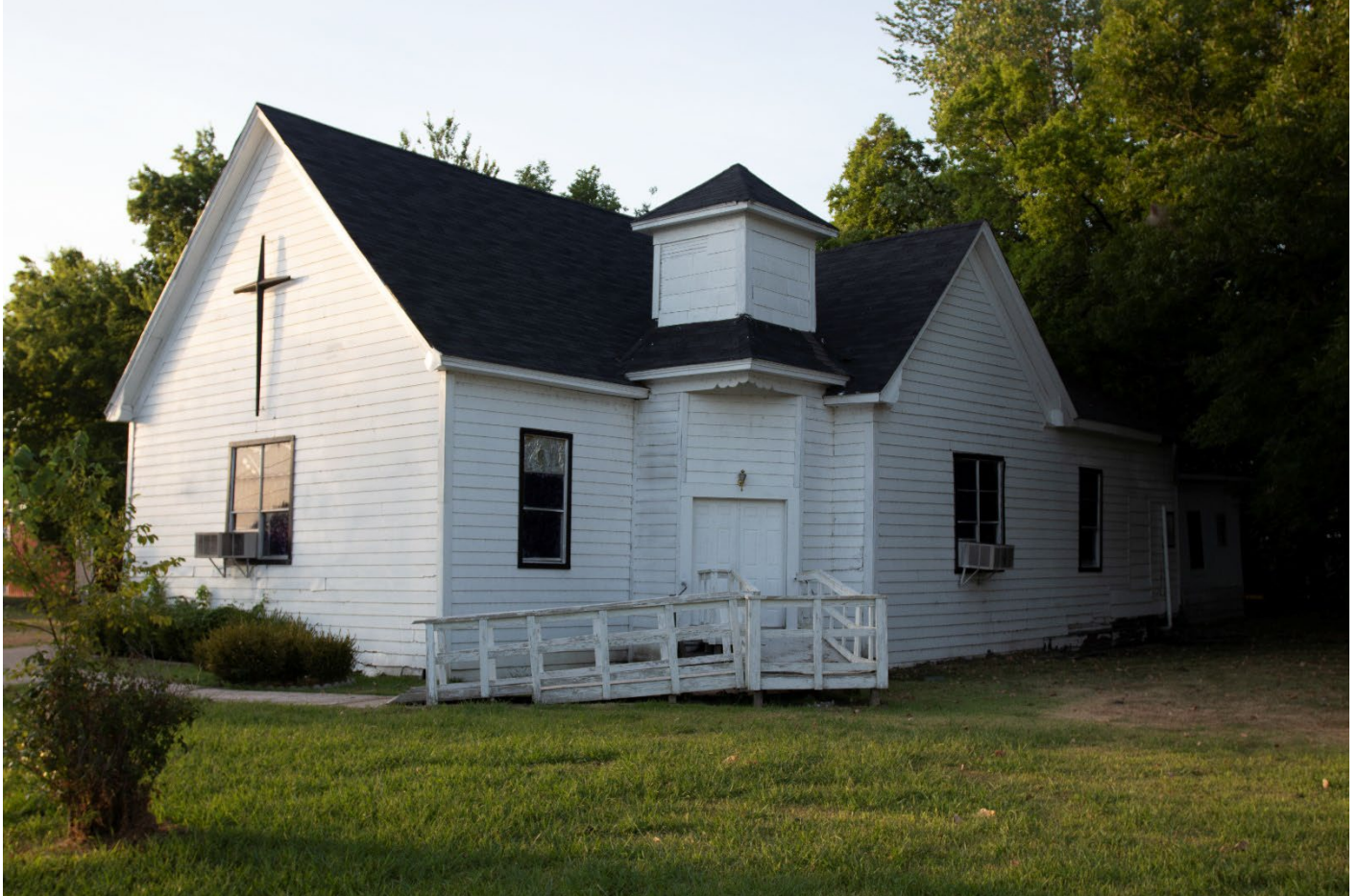
Photo 7: Northwest oblique showing second of two main entrances. Scalloped trim is original. Camera looks southeast.
