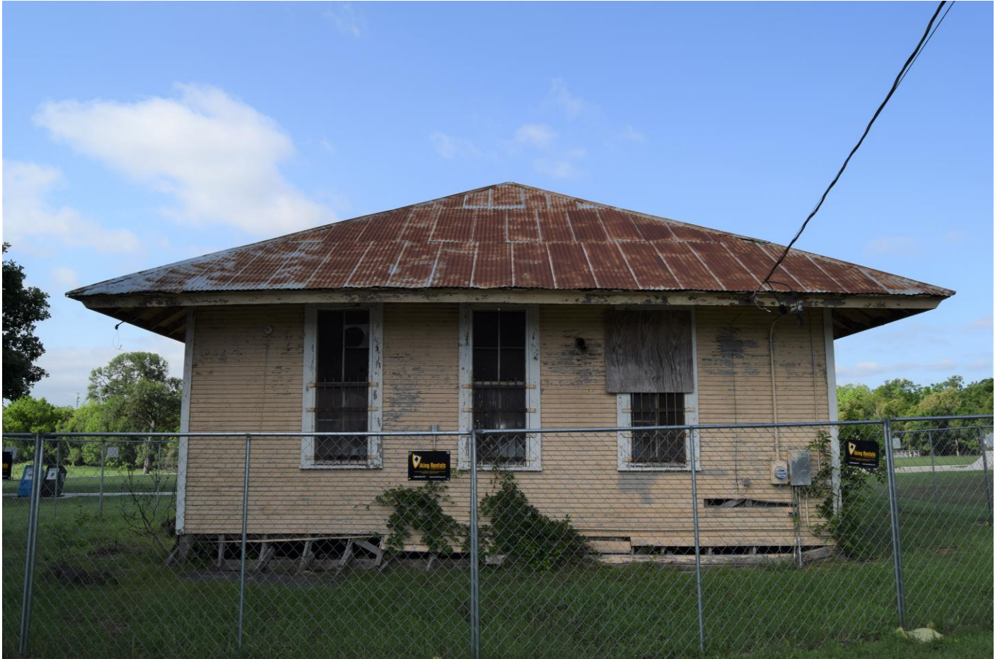
Photograph 6. Northeast exterior façade, view facing southwest.
