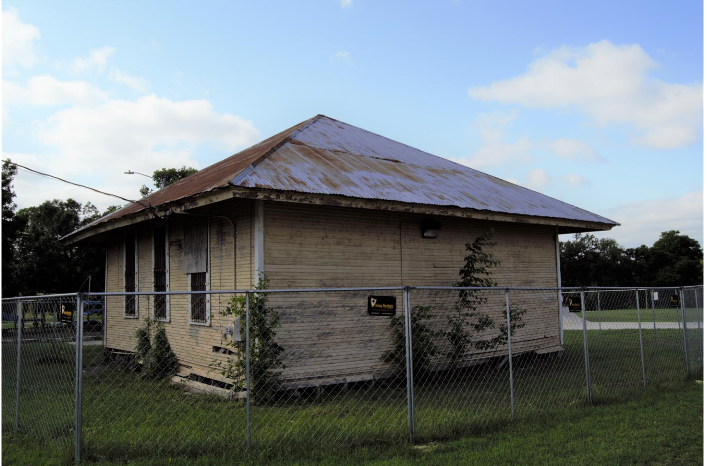
Photograph 7. North exterior oblique, view facing south.
