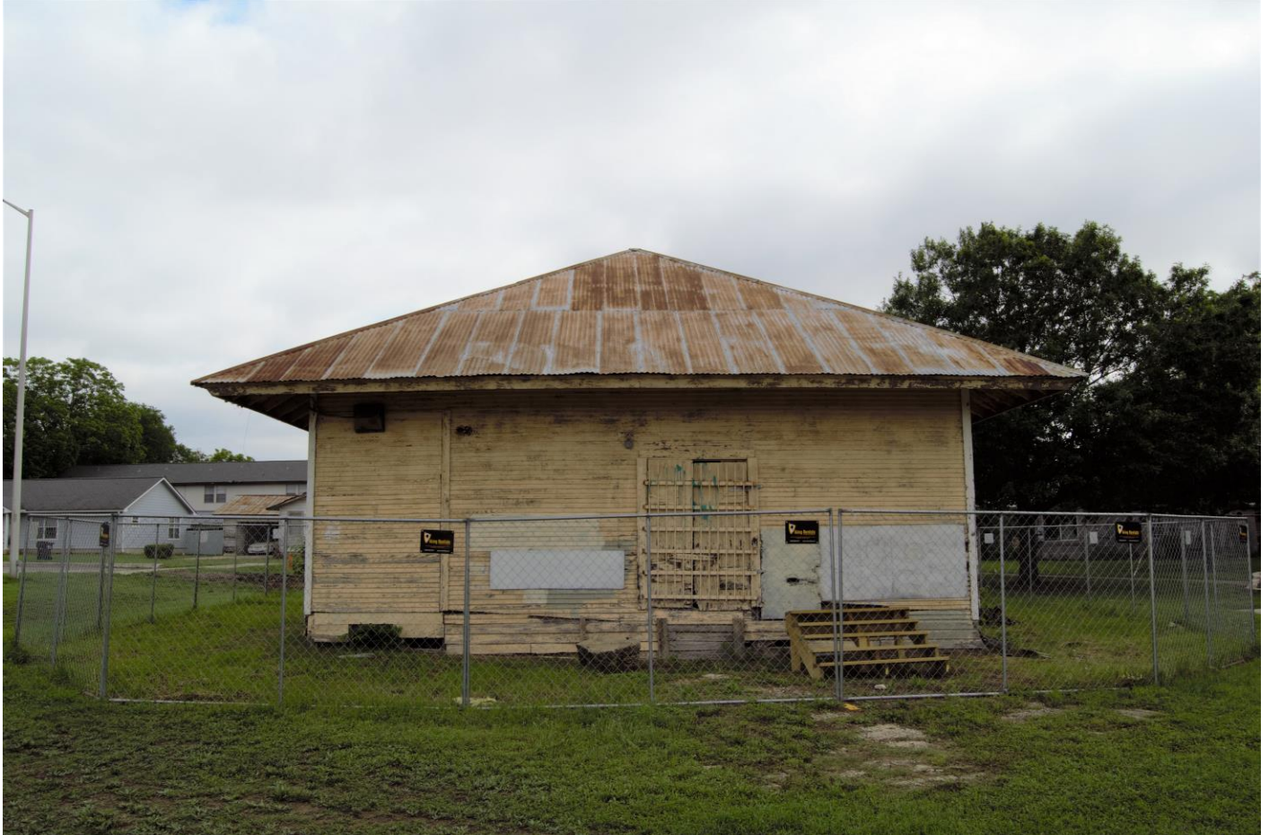
Photograph 2. Primary (southwest) exterior façade, view facing northeast.
