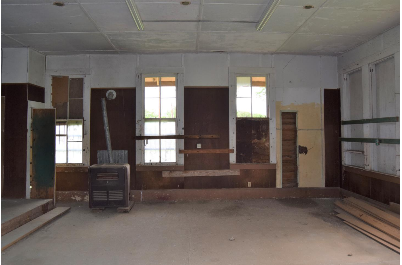
Photograph 8. Northeast wall of interior, view facing northeast.
