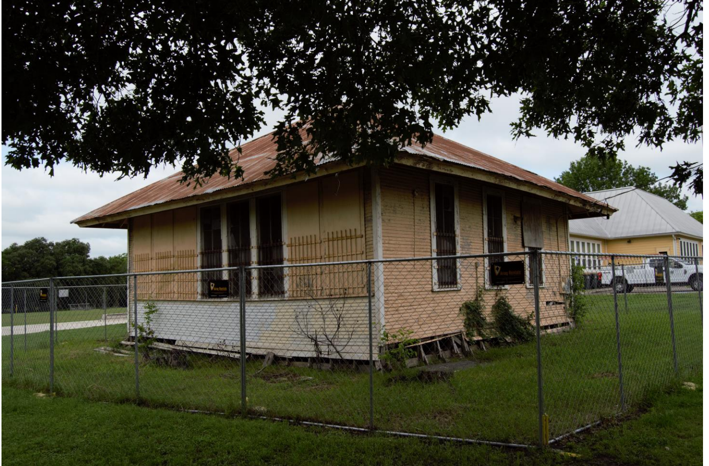
Photograph 5. East exterior oblique, view facing west.
