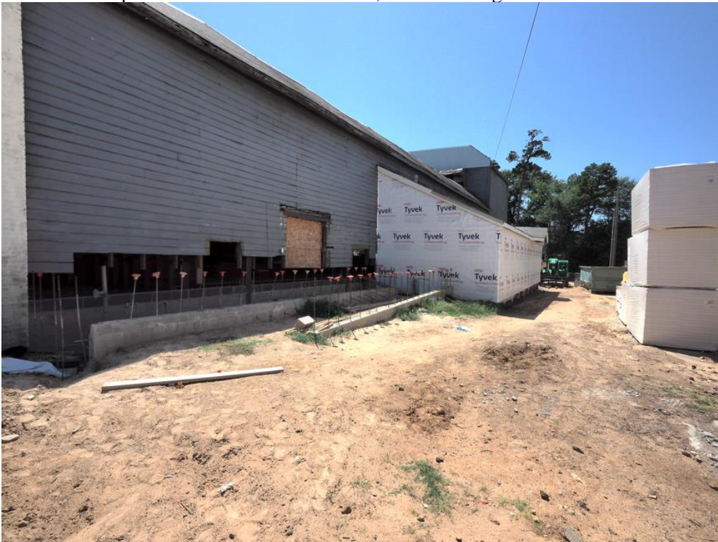
Photo 4. Oblique view of northeast elevation, camera facing west.
