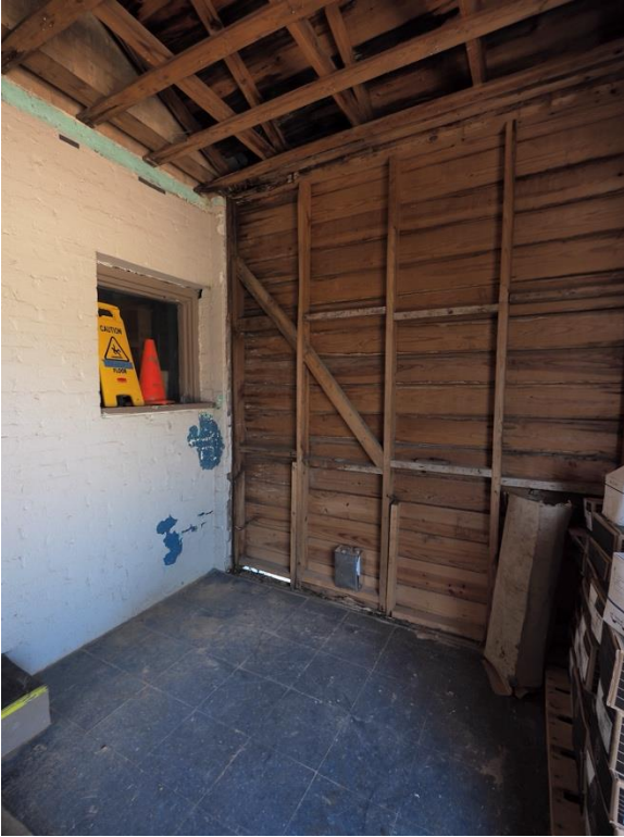
Photo 7. Interior view of vestibule with original ticket window, camera facing north.
