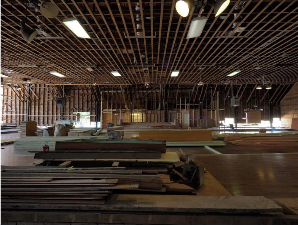
Photo 18. View of steel wall structure, visible during construction, camera facing northwest.
