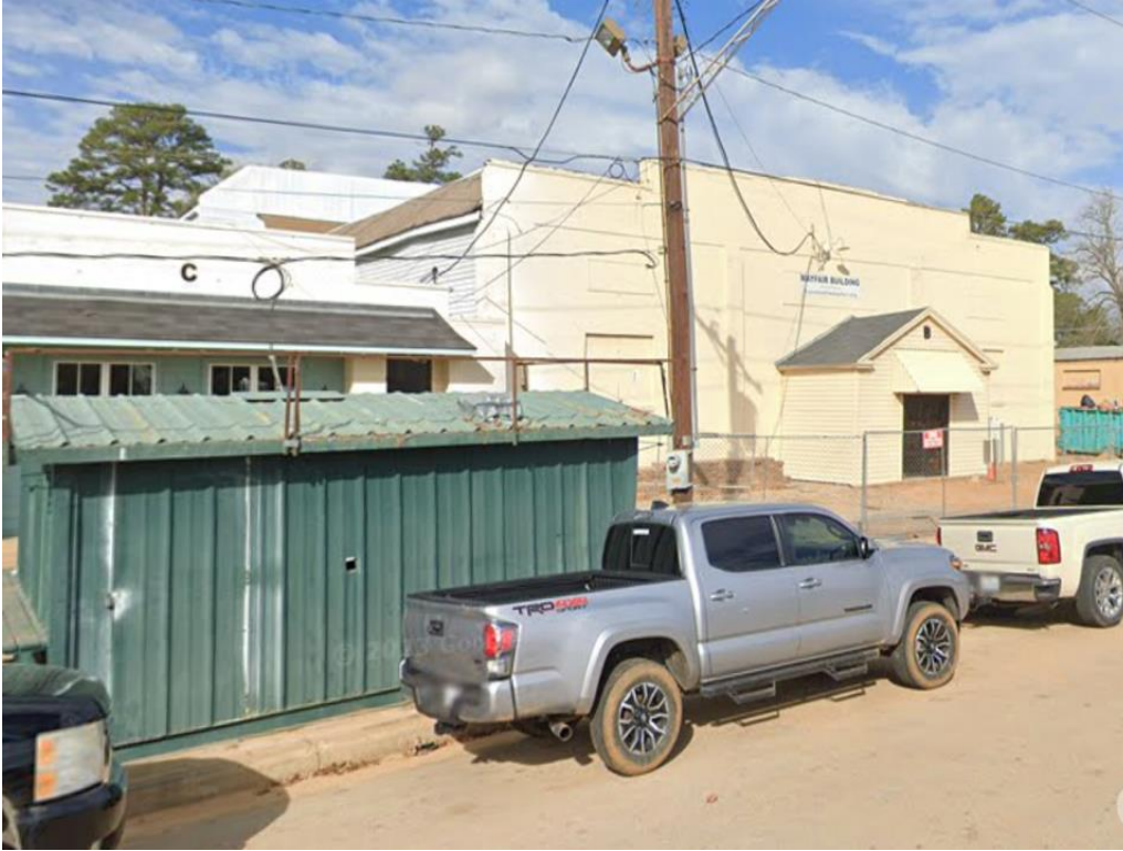
Photo 5. Oblique view of front façade and southwest elevation, camera facing north.
