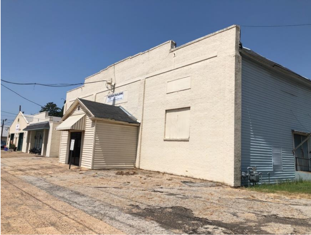
Photo 3. Oblique view of front façade with vestibule, camera facing west.
