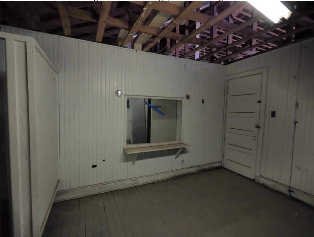
Photo 16. Interior dressing room behind stage, camera facing south.
