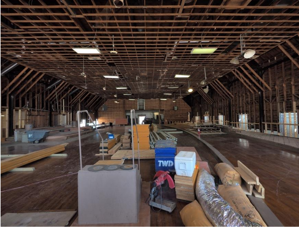
Photo 9. Interior view from rear wall, camera facing southeast.
