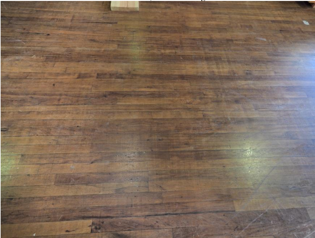
Photo 19. Detail view of oak dance floor, camera facing northwest.
