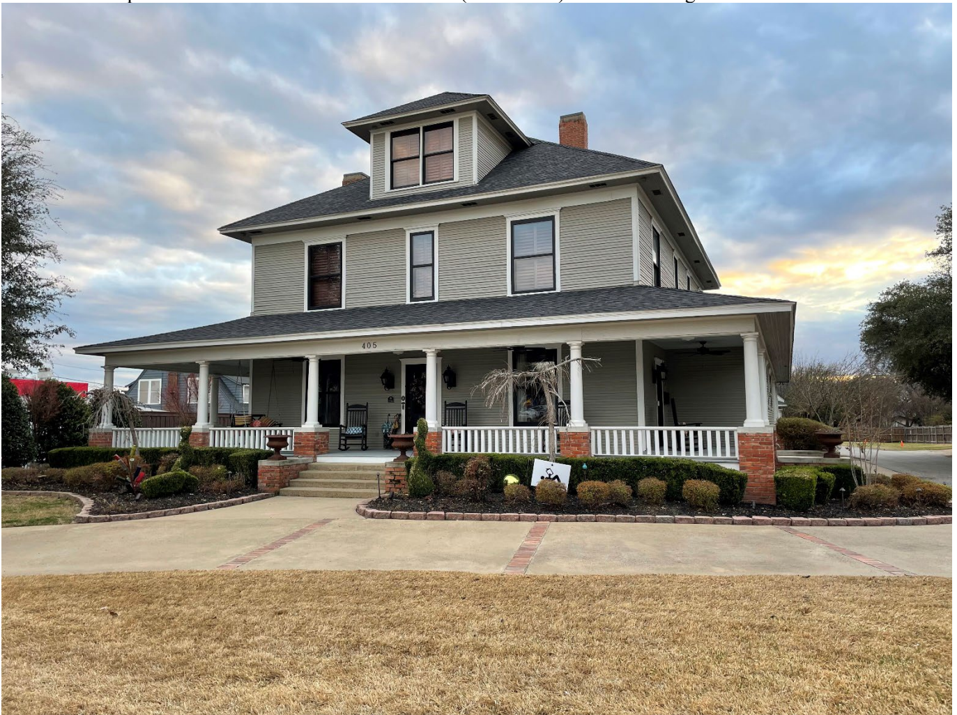
Photo 14. Oblique view of 405 West Marvin Avenue A (Resource 2). Camera facing southwest.
