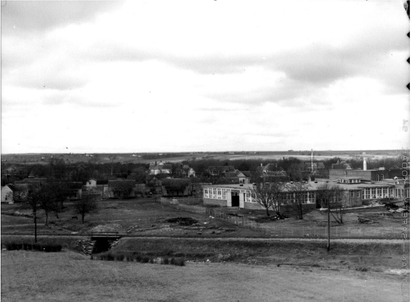
Figure 4. View of the Waxahachie Cotton Mill along the Houston and Texas Central Railway, just south of the West Marvin Avenue-Patrick Street Historic District, looking north, date unknown. Source: Ellis County Museum.
