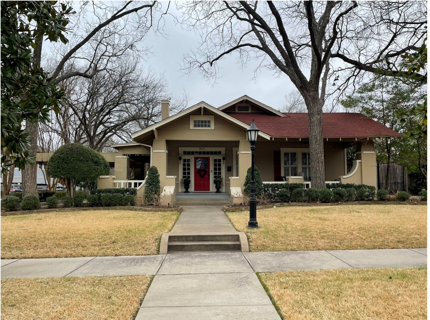
Photo 34. Frontal view of 905 West Marvin Avenue A (Resource 55). Camera facing southwest.
