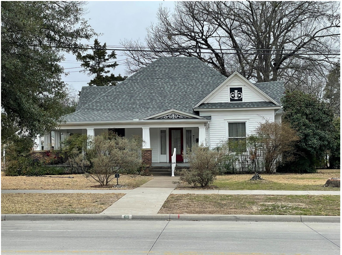
Photo 26. Frontal view of 611 West Marvin Avenue A (Resource 34). Camera facing southwest.
