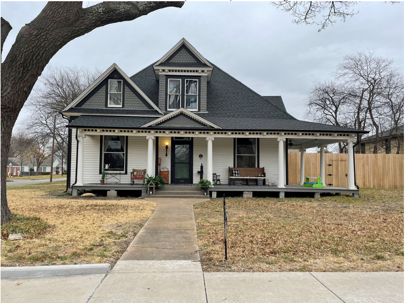
Photo 22. Frontal view of 514 West Marvin Avenue (Resource 23). Camera facing northeast.
