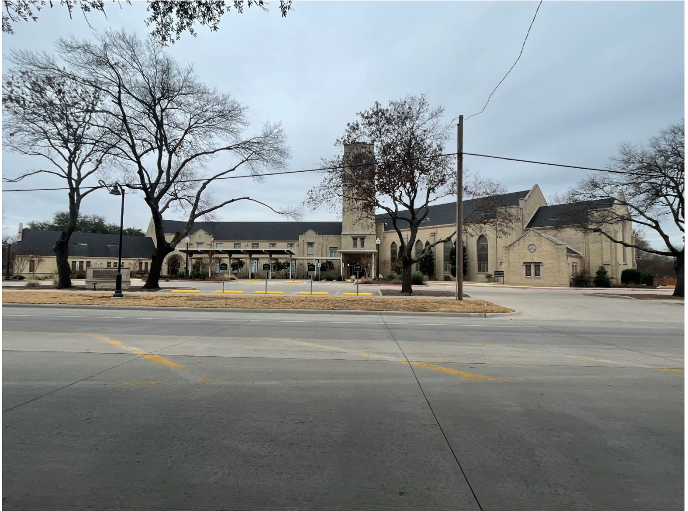
Photo 20. Oblique view of First United Methodist Church (Resource 16), located at 505 West Marvin Avenue A. Camera facing south.
