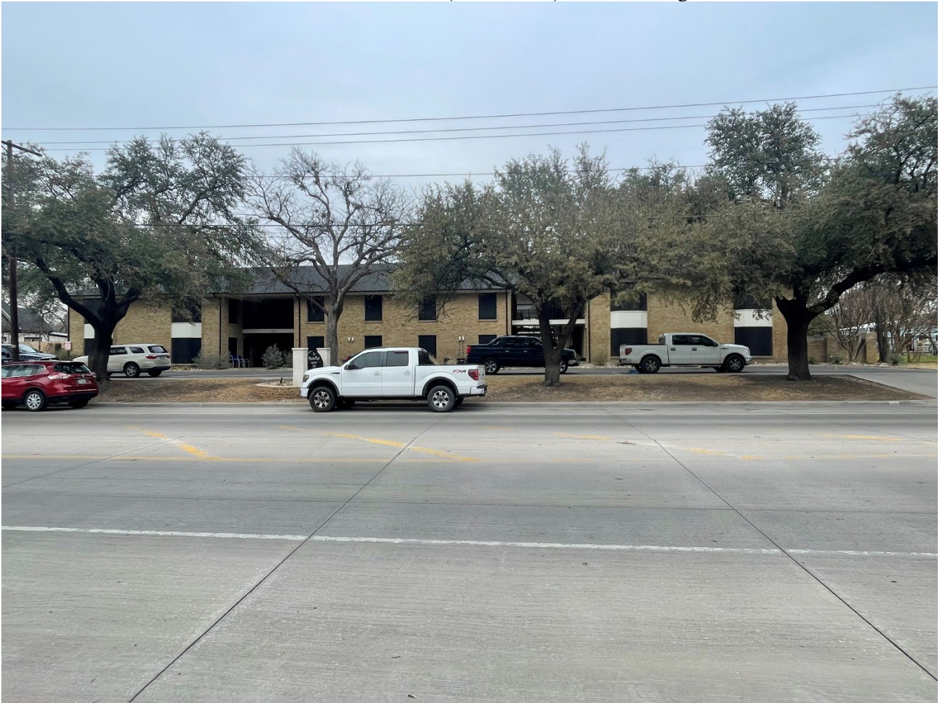
Photo 21. Frontal view of 506 West Marvin Avenue A (Resource 18). Camera facing northeast.
