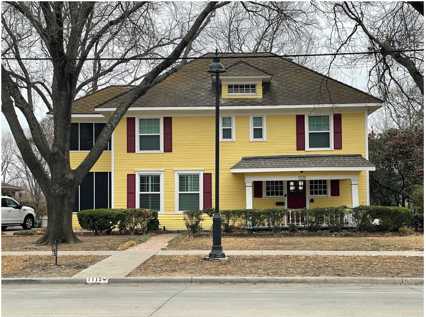
Photo 44. Frontal view of 1119 West Marvin Avenue A (Resource 80). Camera facing southwest.
