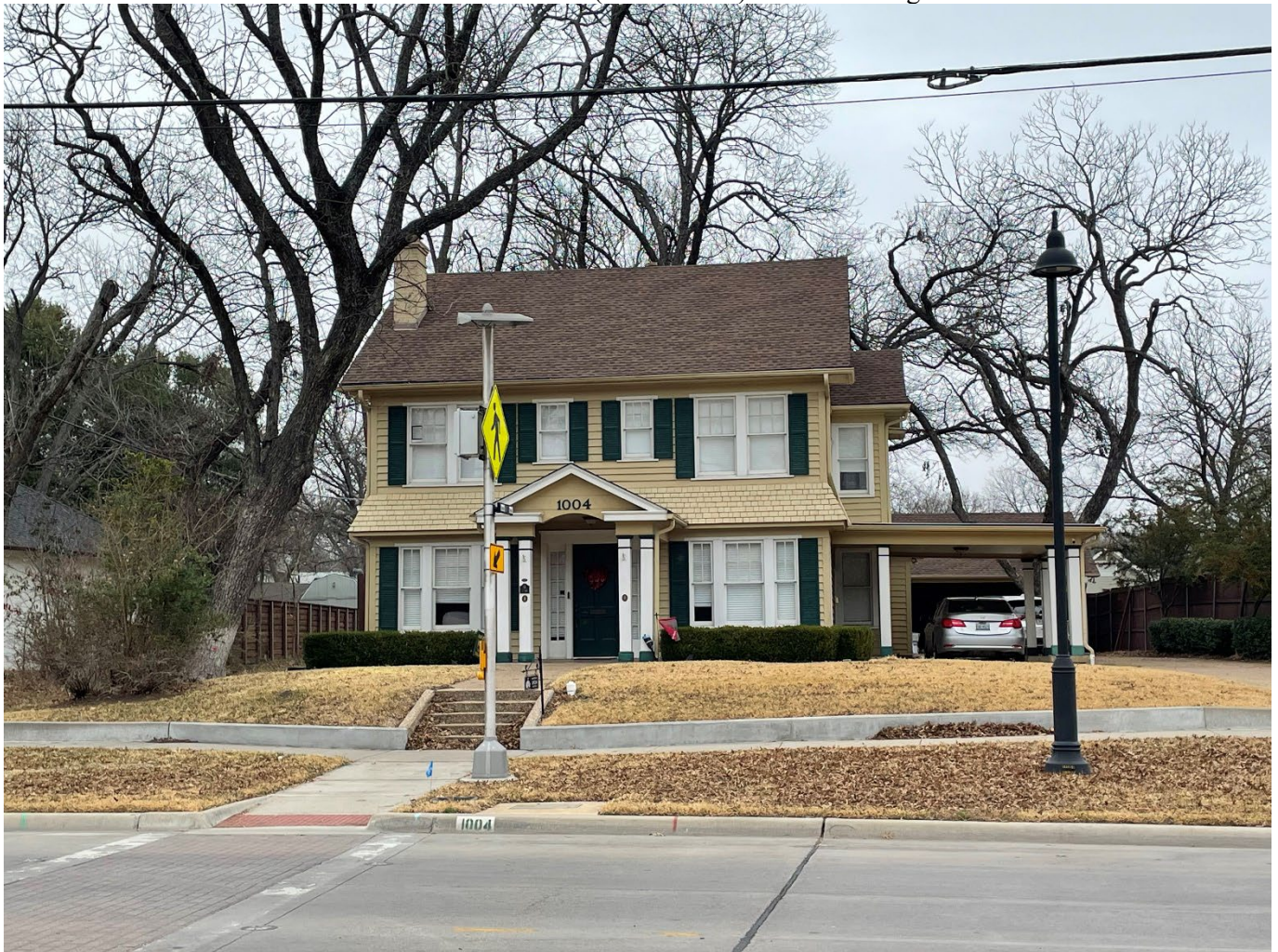
Photo 41. Frontal view of 1004 West Marvin Avenue (Resource 70). Camera facing northeast.
