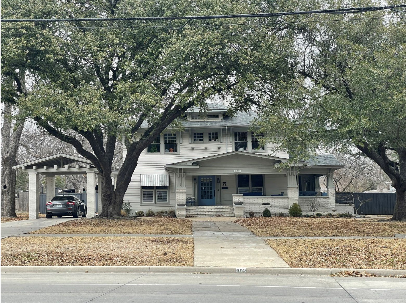
Photo 33. Frontal view of the E.F. Phillips House, 902 West Marvin Avenue (Resource 54). Camera facing northeast.
