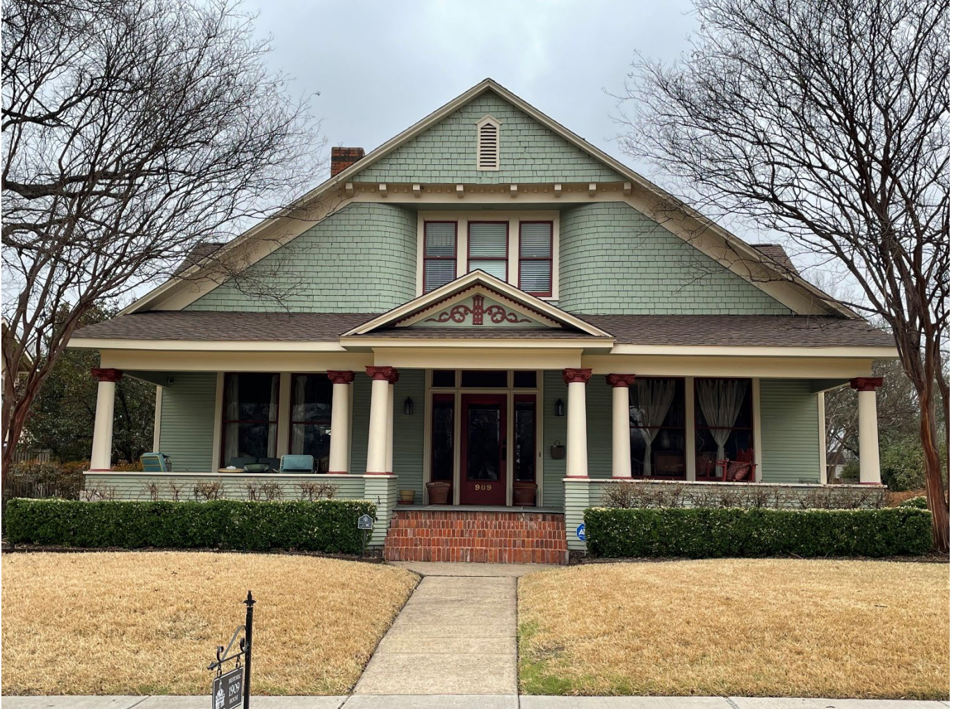
Photo 36. Frontal view of the Dr. L.H. Graham House, 909 West Marvin Avenue A (Resource 58). Camera facing southwest.
