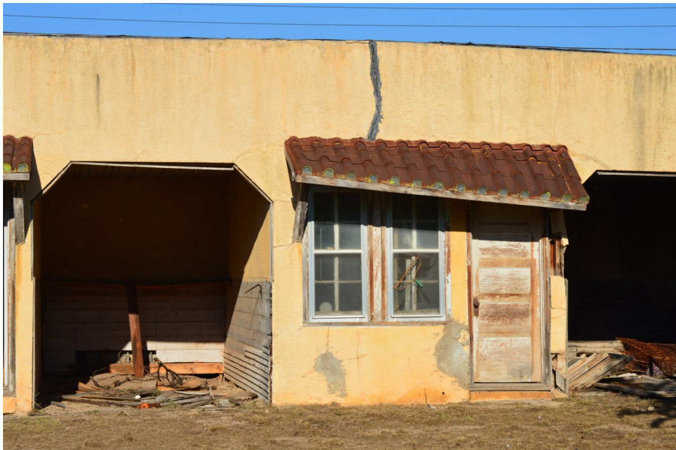
Photo 9 Open car bays, camera facing north
