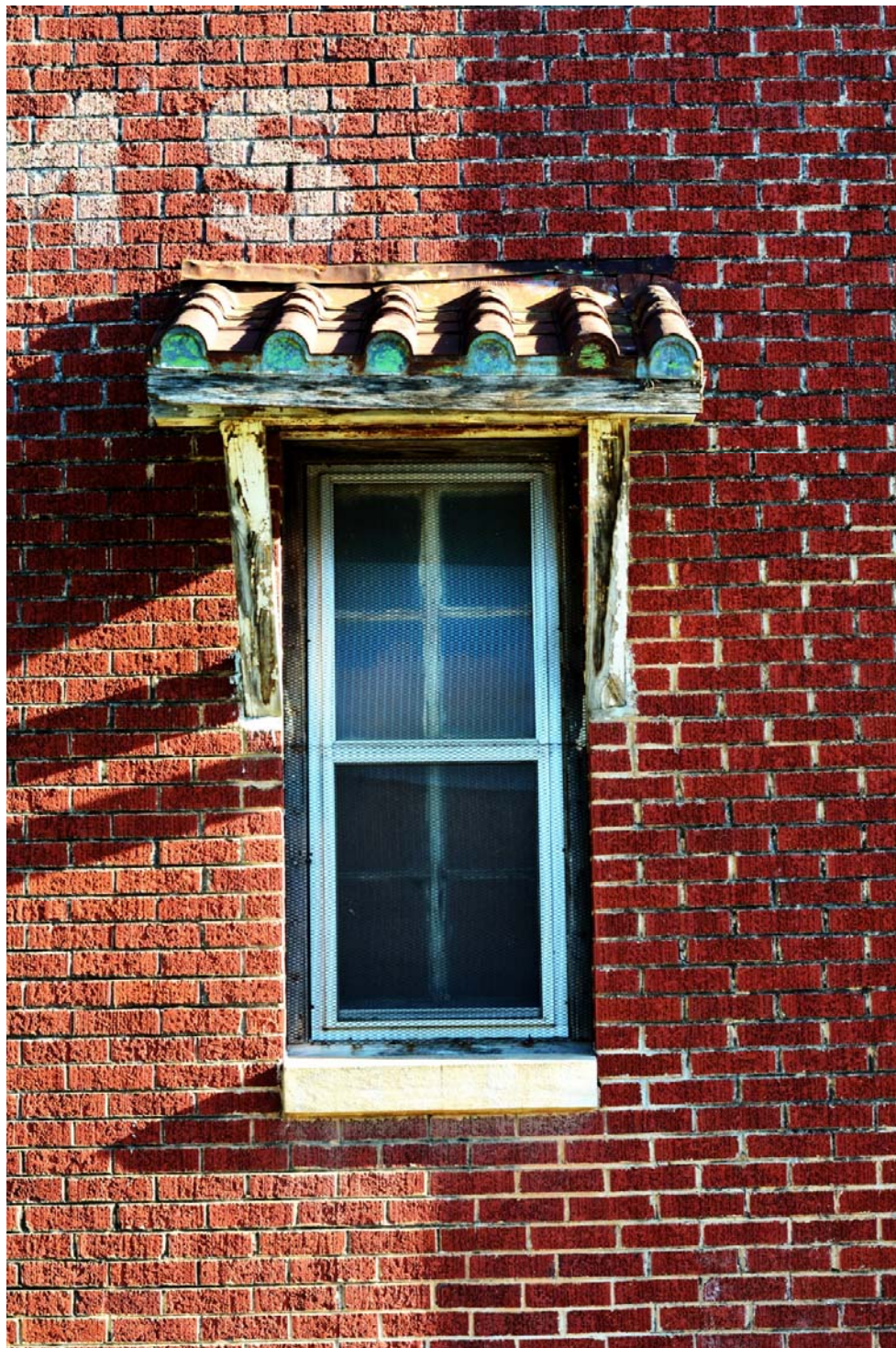
Photo 5: Original window on north elevation, camera facing south
