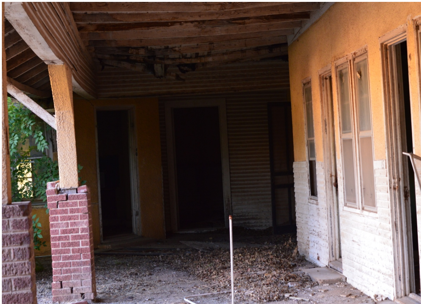
Photo 8 Western row of rooms with awning, camera facing south
