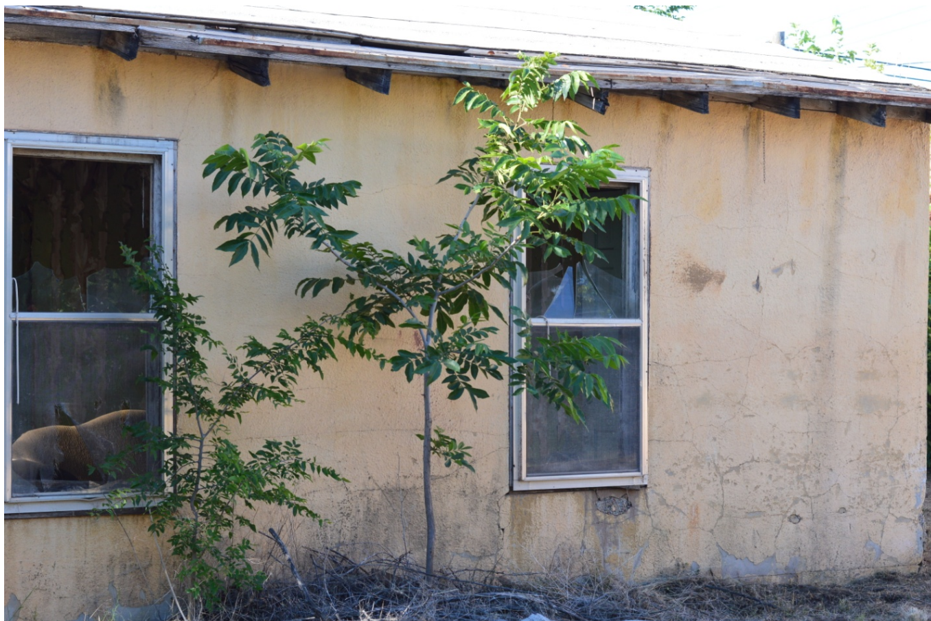
Photo 12 Shed addition with sloped roof, camera facing north
