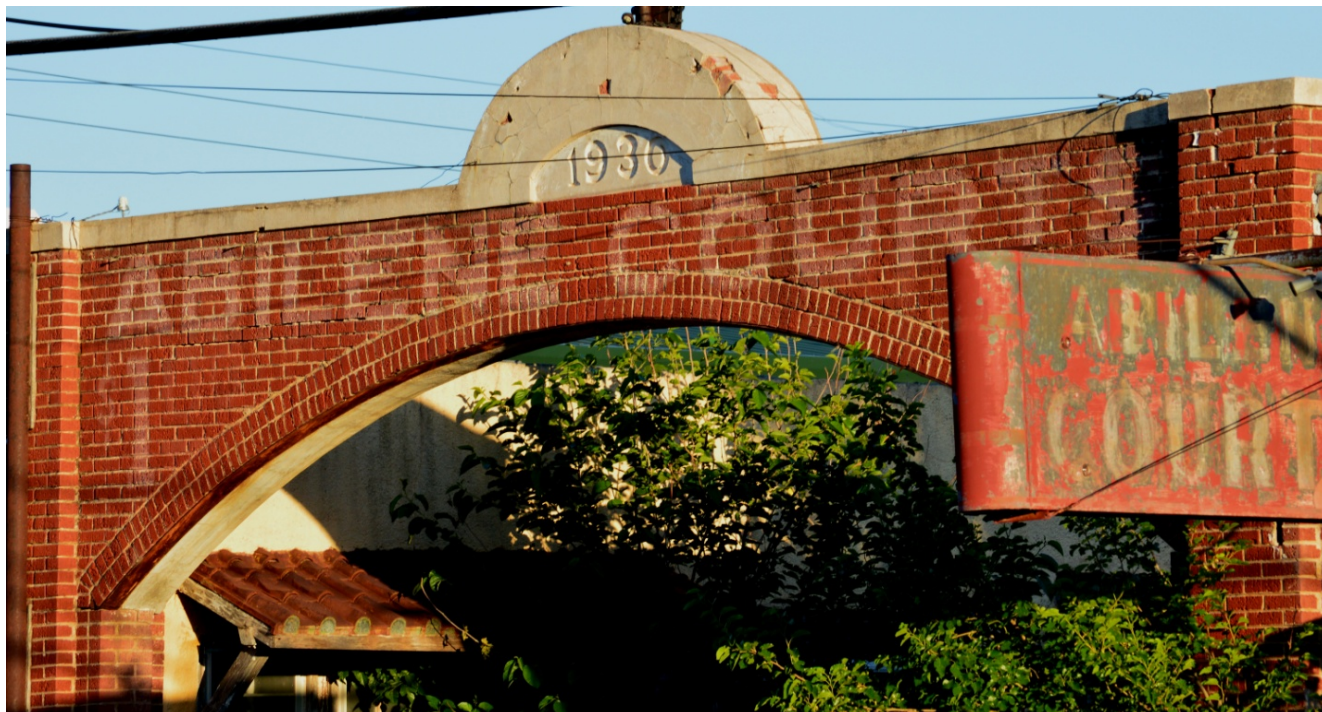
Photo 2 Archway over drive, camera facing southeast
