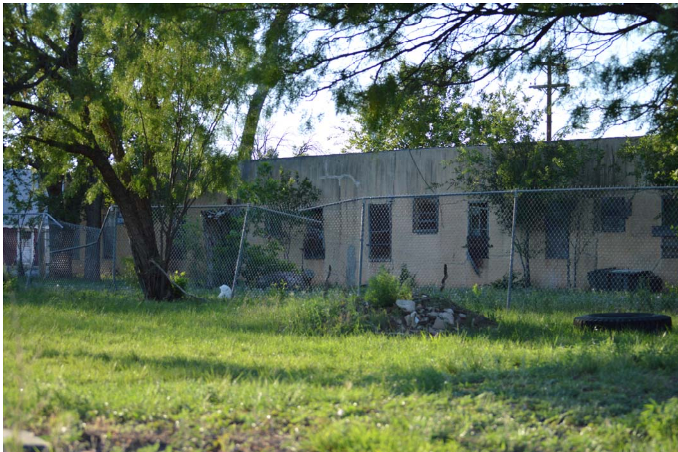
Photo 13 Southern façade, camera facing northwest
