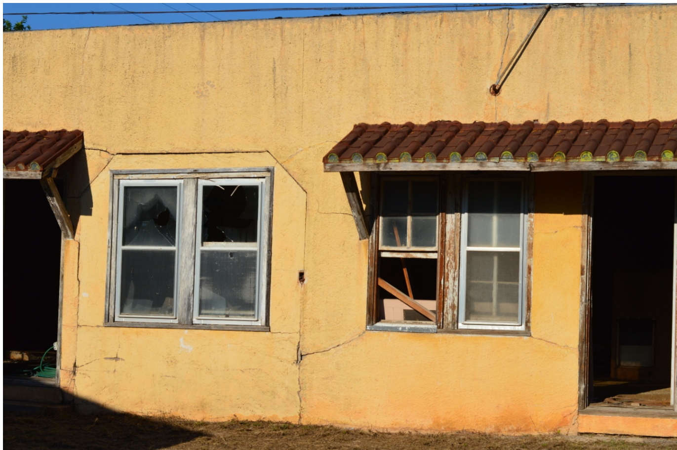
Photo 10 Open car bays, camera facing north
