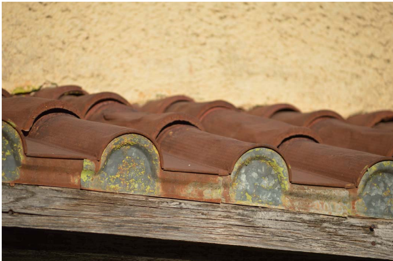
Photo 11 Metal roof cover detail
