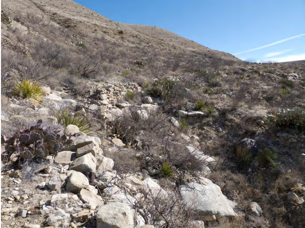
Photograph 8: Overview of Road Segment 6 (2Z) with stone retaining wall and fill (2Q).
