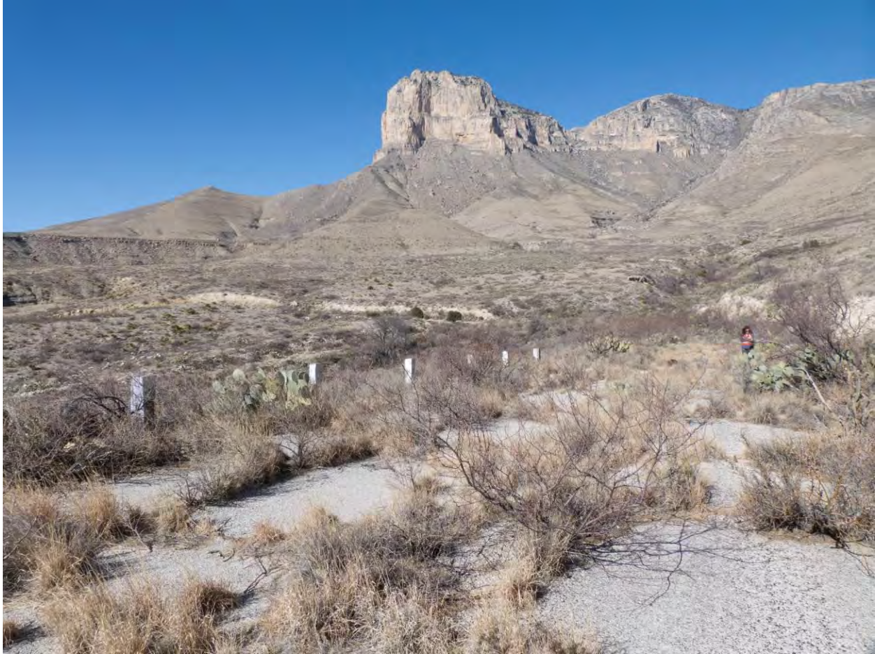
Photograph 15: 1937 US Highway 62 (Road Segment 1/2U) with Masonry Guard Posts (2J)
