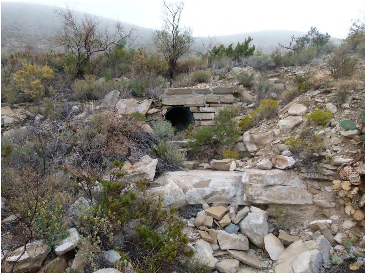
Photograph 14: 1937 Metal Culvert and Stone Headwall (TYP.) along Road Segment 1 (2A).
