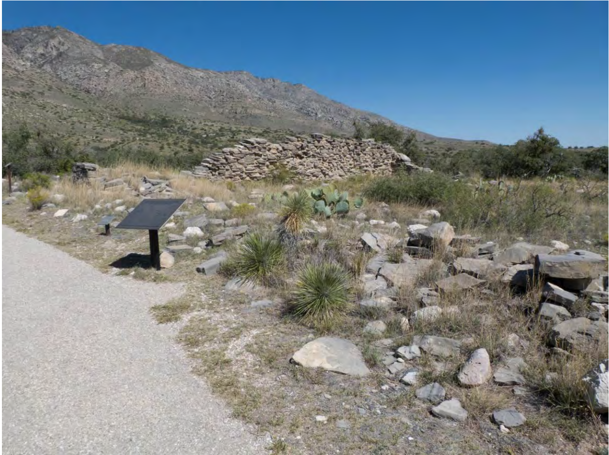
Photograph 1: Pinery Station Ruins (1C) (NRIS 74000281; 41CU193)
