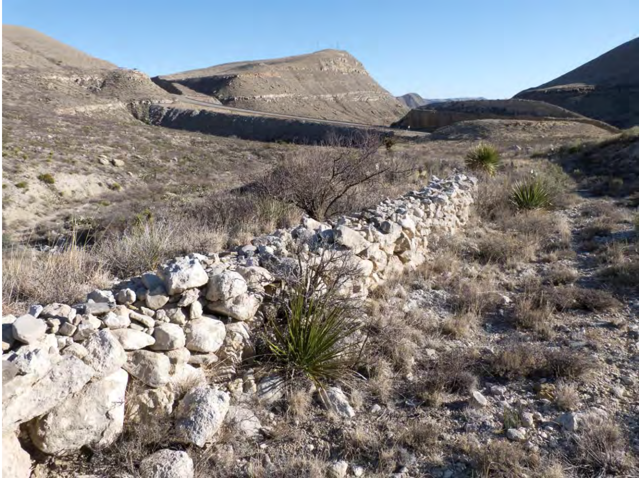
Photograph 13: Stone Guard Fence (2K) on Road Segment 2 (2V). Overview of Valley, current US Highway 62/180 fill and alignment in background.
