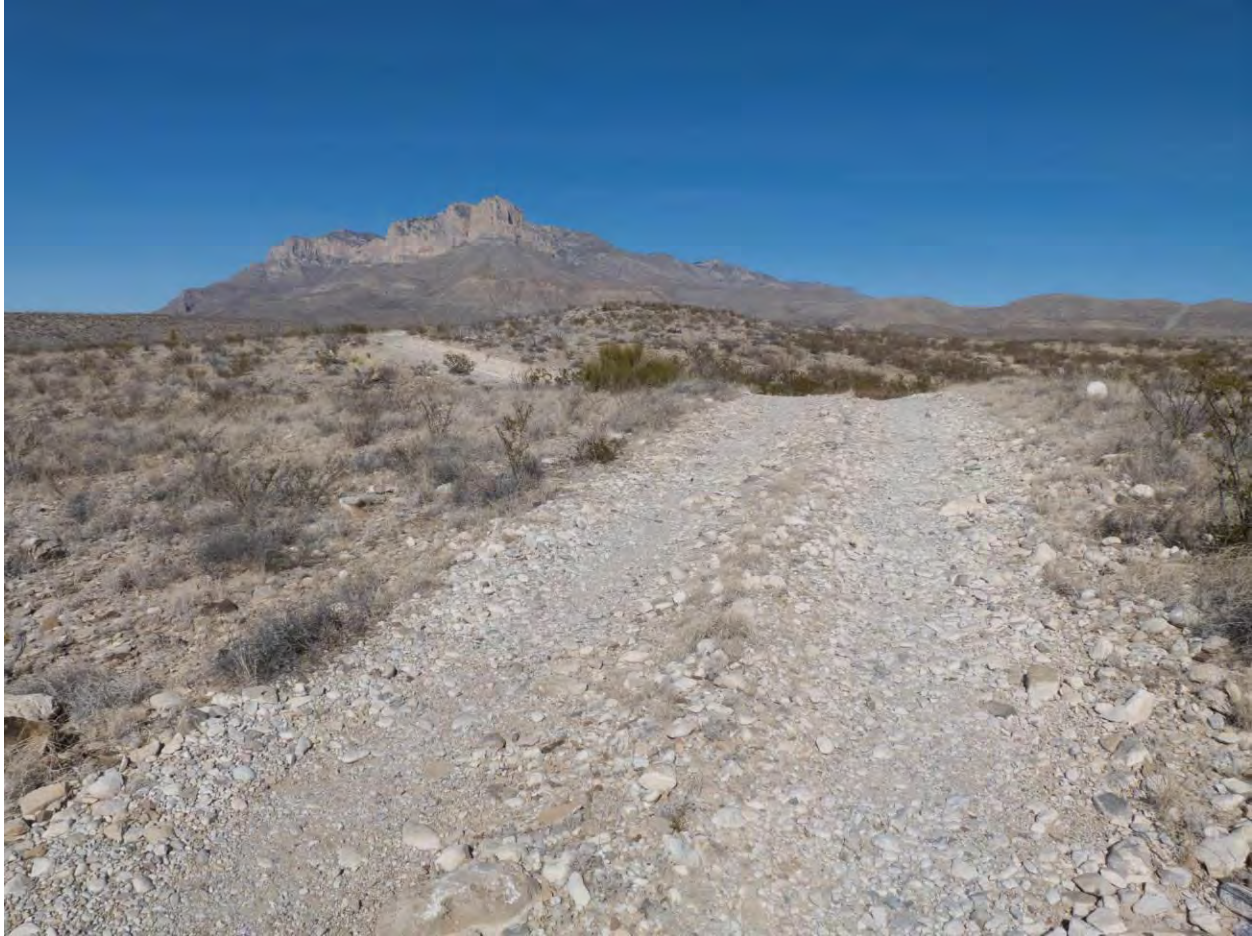
Photograph 16: Overview of Road Segment 27 (3C) – Williams Ranch Road.
