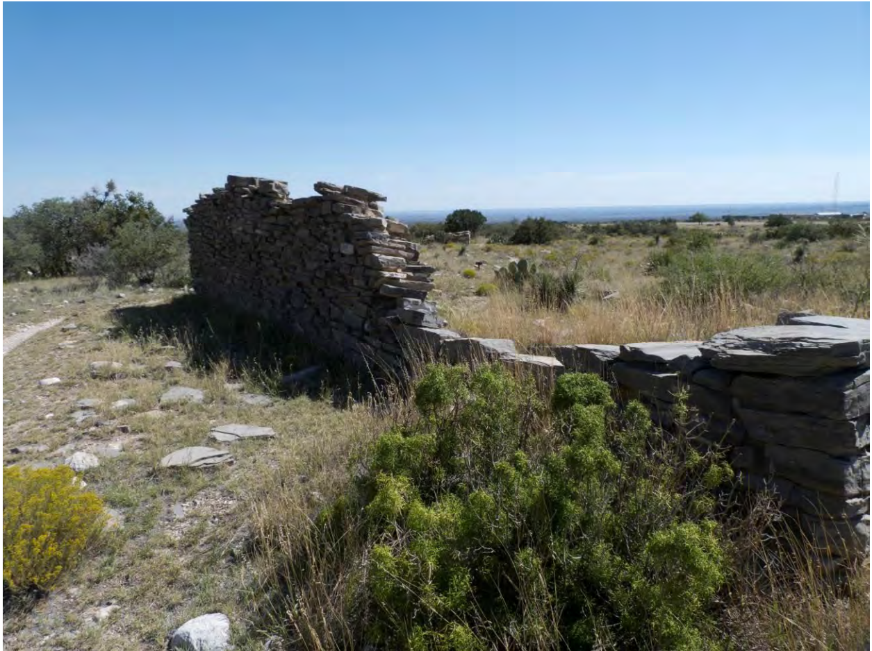
Photograph 2: Pinery Station Ruins (1C) (NRIS 74000281; 41CU193)
