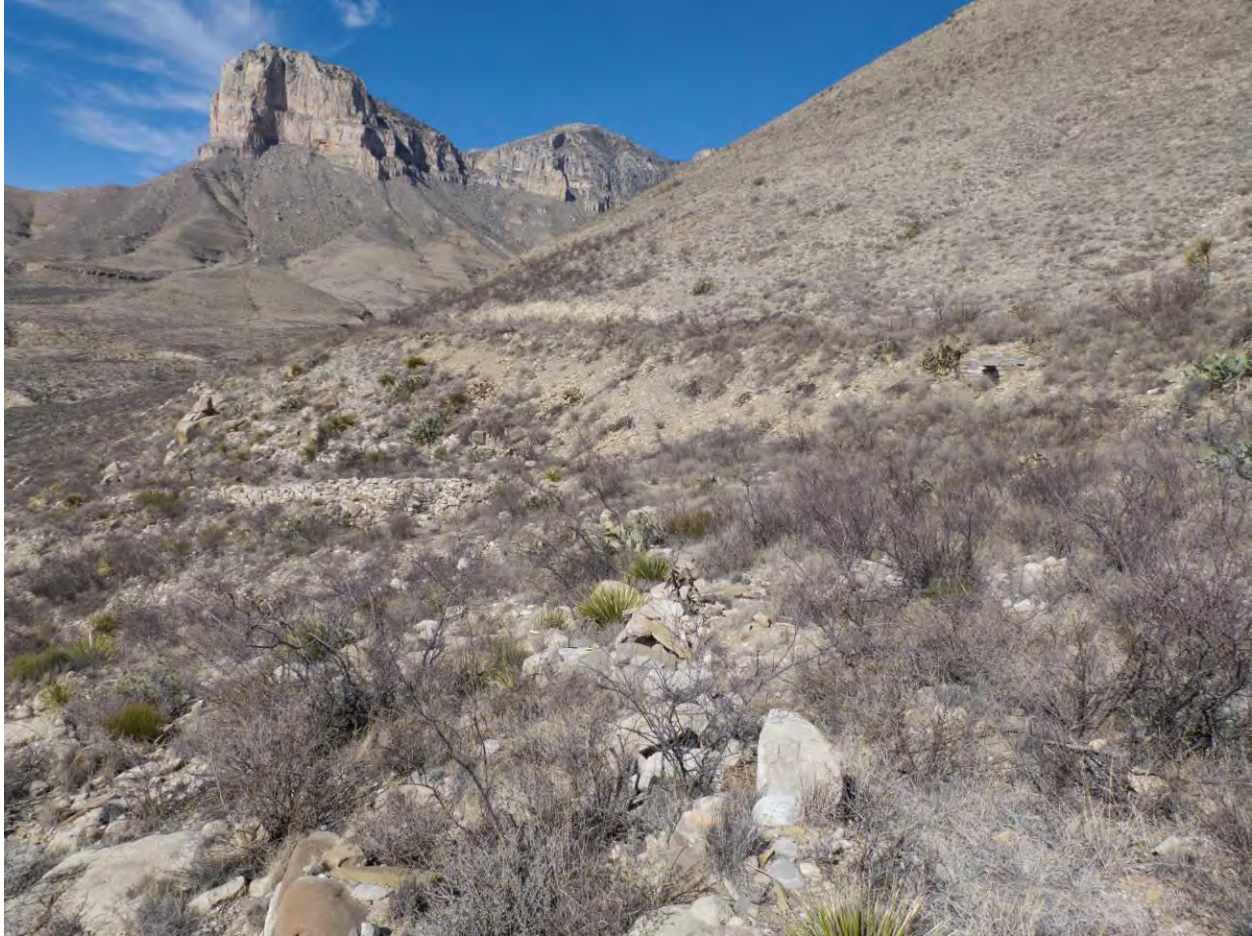
Photograph 7: Overview of Road Segment 6 (2Z) with stone retaining wall (2Q) and Road Segment 1 (2U) with culvert headwall (2C).
