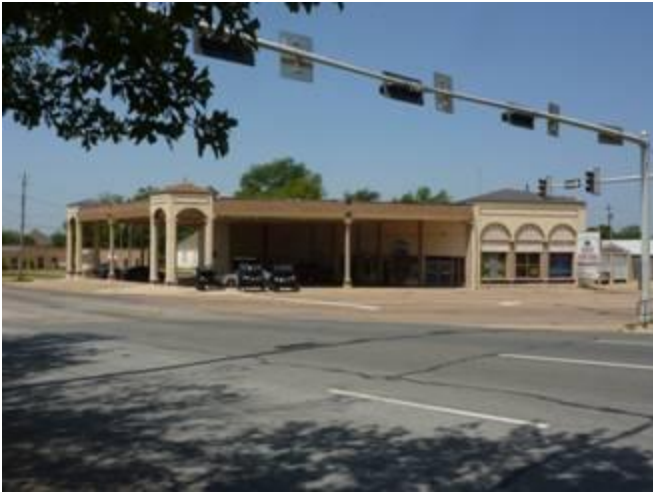
Photo Courtesy of THC staff: Auto repair shop in Texarkana
